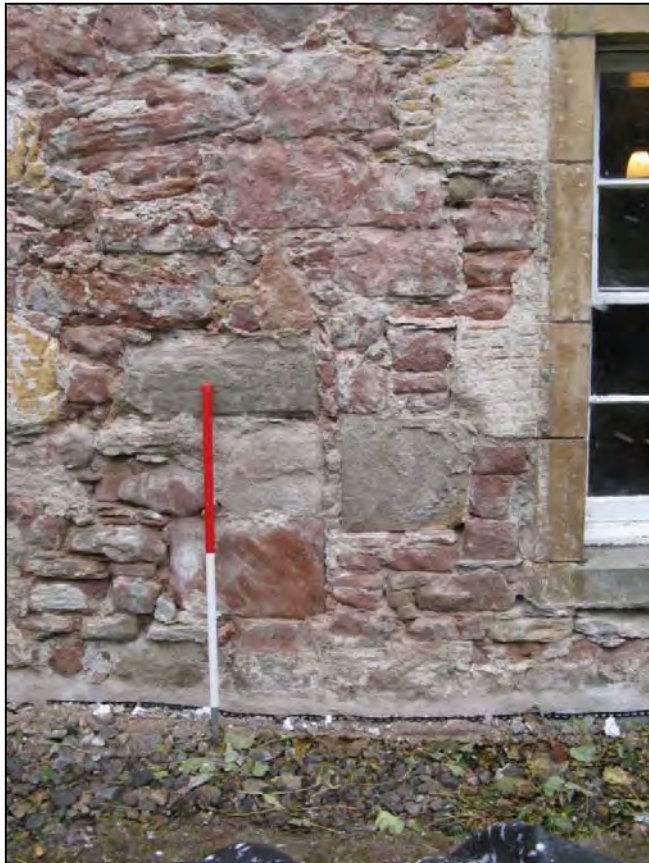
Plate 13 Quoins in S wall, approximately opposite corner of N aisle
