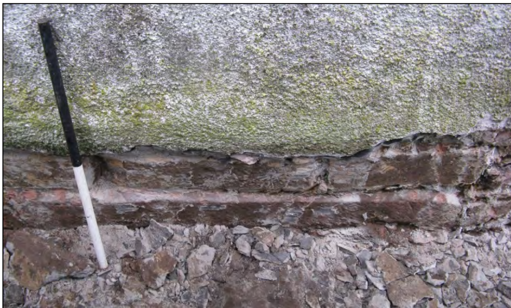
Plate 6 Dressed flat slabs reused in foundations: north wall of west aisle
