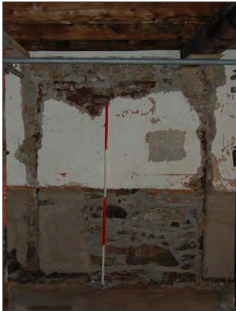
Plate 7 Blocked doorway (interior view)
