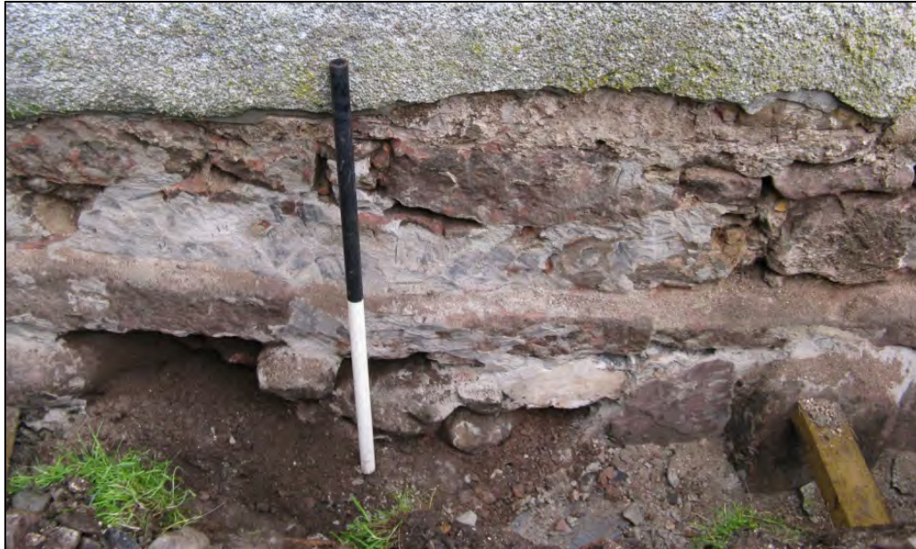
Plate 5 Dressed flat slabs reused in foundations: south wall of west aisle
