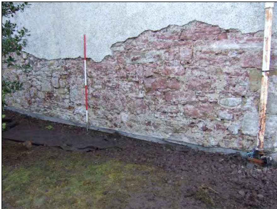
Plate 8 Blocked doorway opening visible in N wall of W aisle
