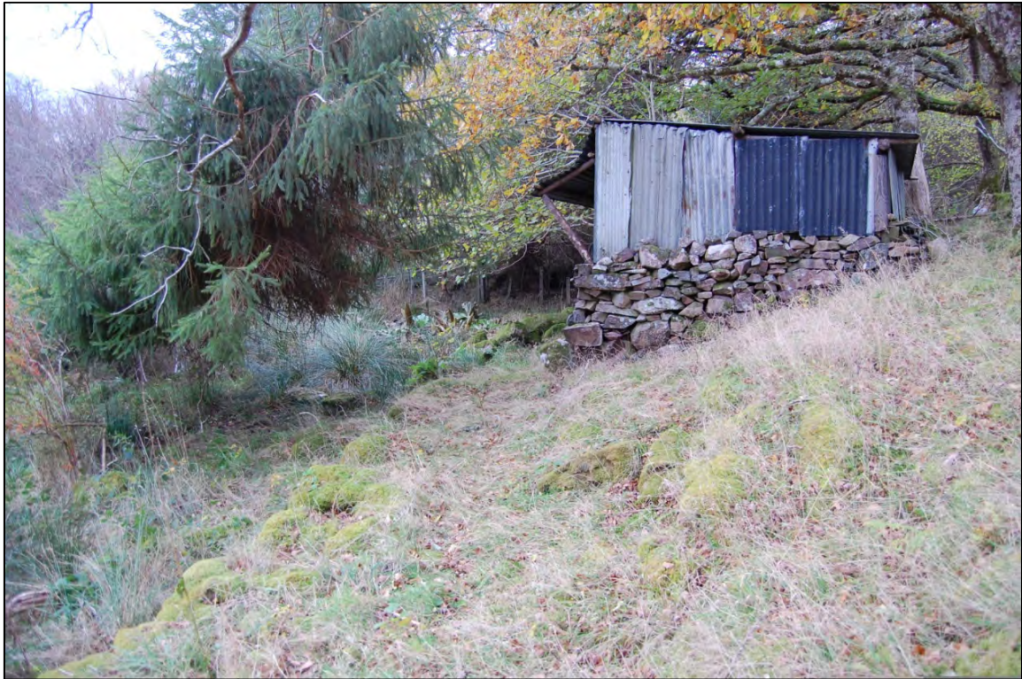
Photo 1 Corrugated shed (F7) to R of path; revetment wall (F1) to L.
