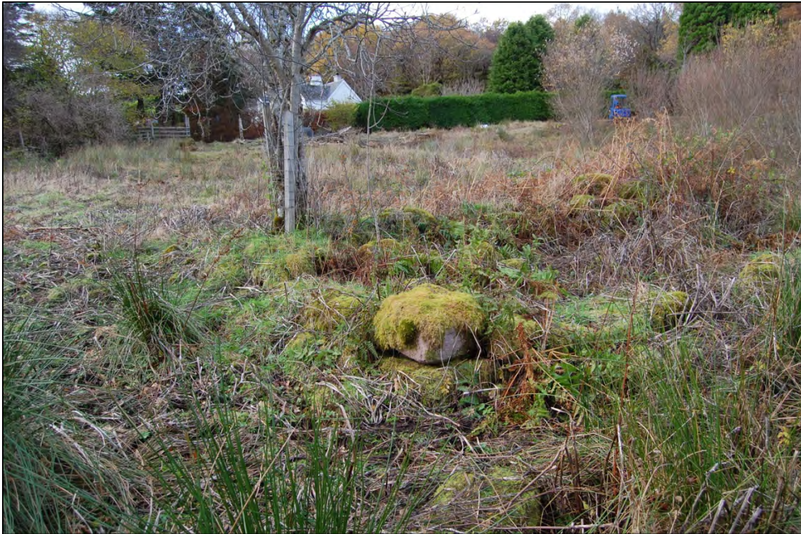
Photo 10 Footings of building F4
