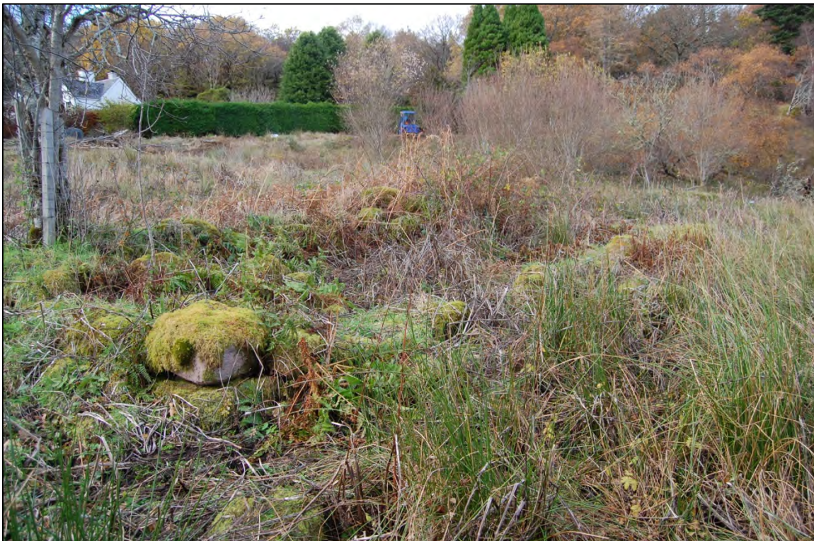
Photo 11 Footings of building F4
