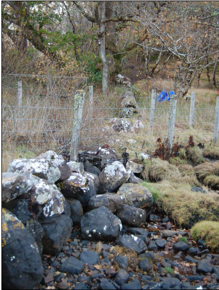
Photo 22 Township dyke F41
