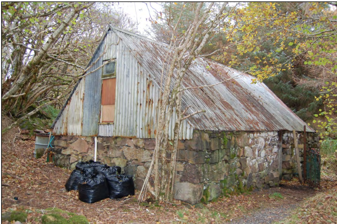
Photo 6 Roofed building F29
