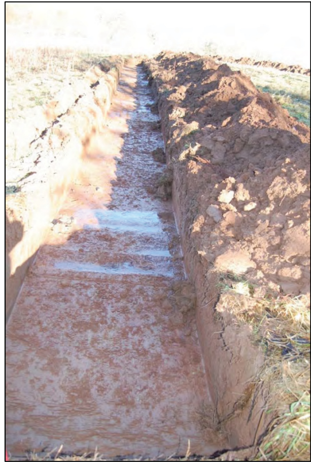
Photo 3 Trench 3 from N
