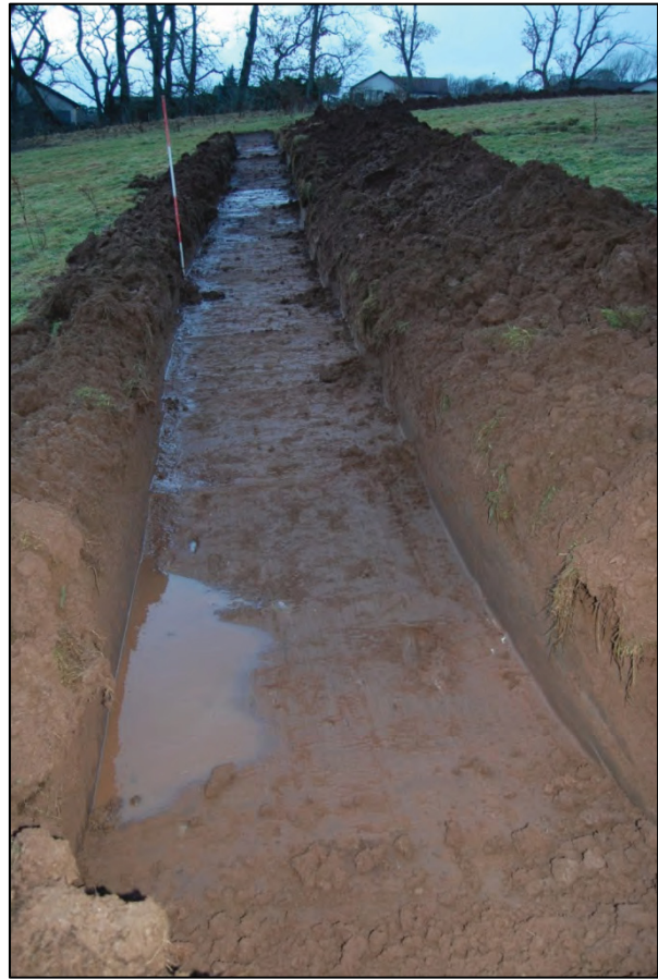
Photo 7 Trench 7, from E
