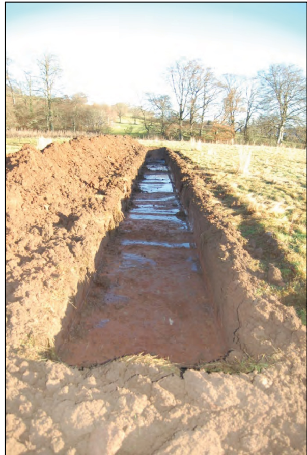
Photo 1 Trench 1 from SW
