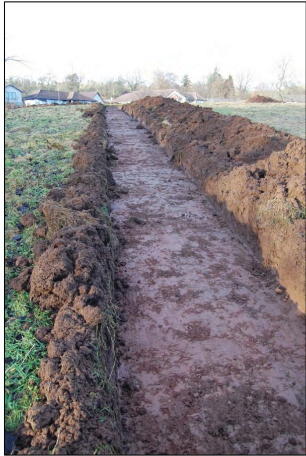
Photo 5 Trench 5 from S
