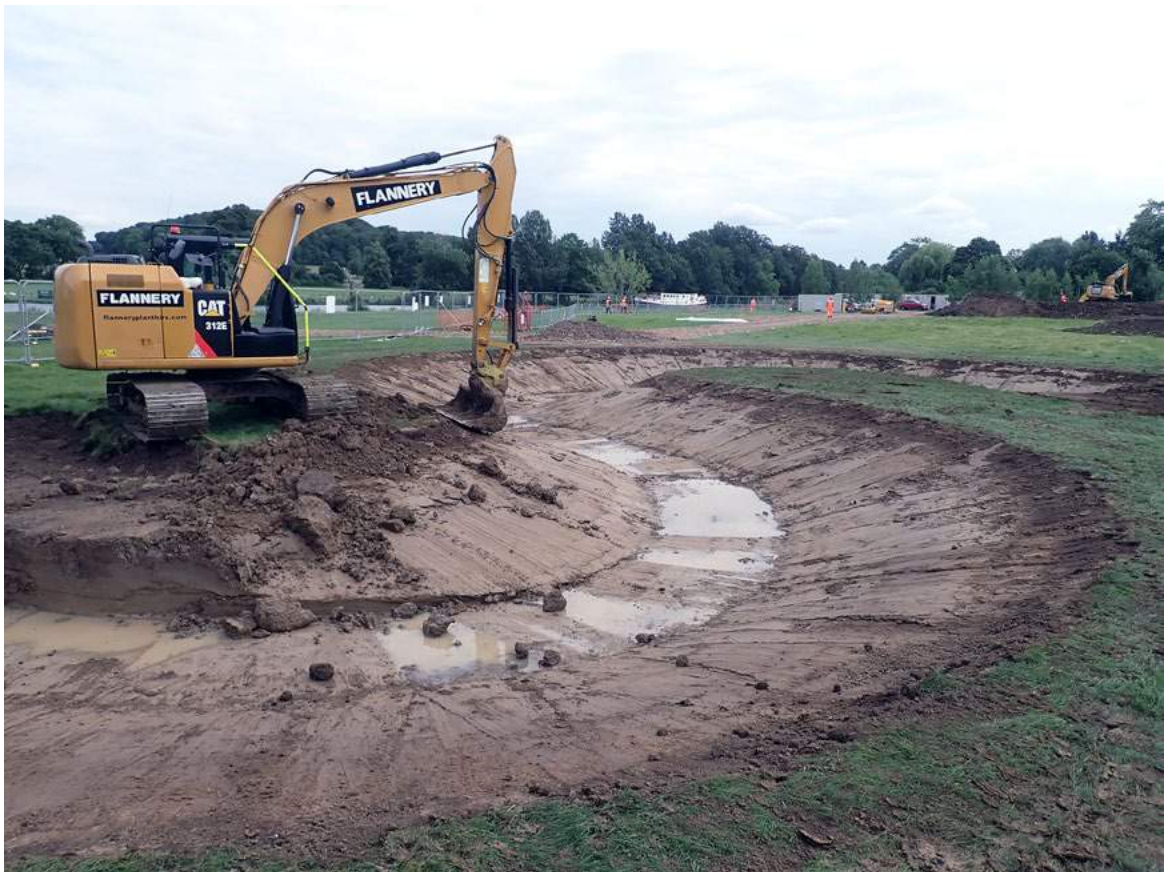
Plate 2: General view of works showing excavation of battered slope
