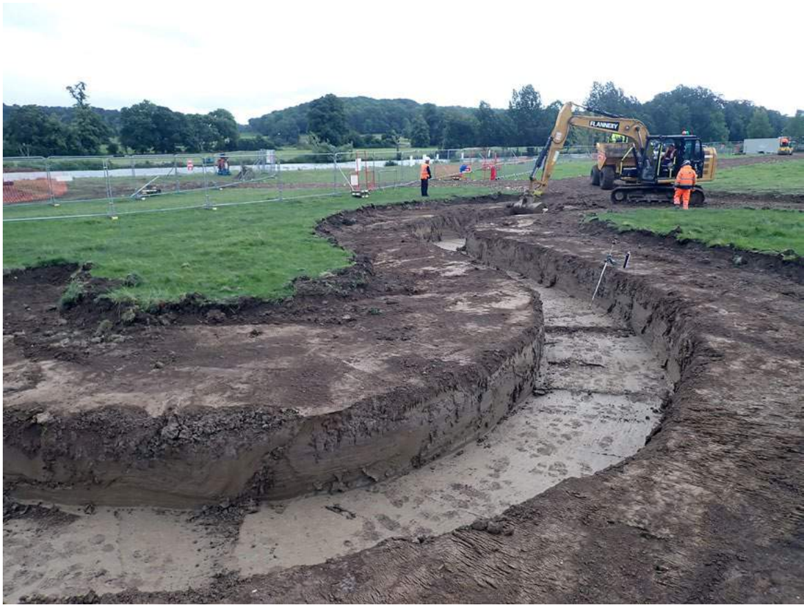
Plate 1: General view of works showing central channel excavation
