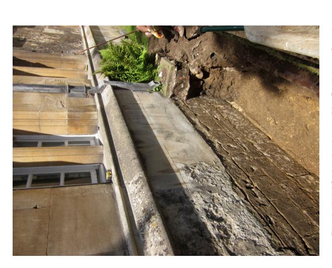
Plate 1: 1675-6 footing showing possible offset in base of trench
