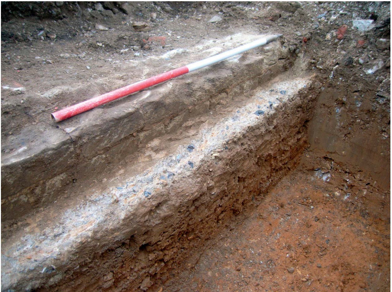
Plate 2: Trench 1, wall 103 and foundation 104
