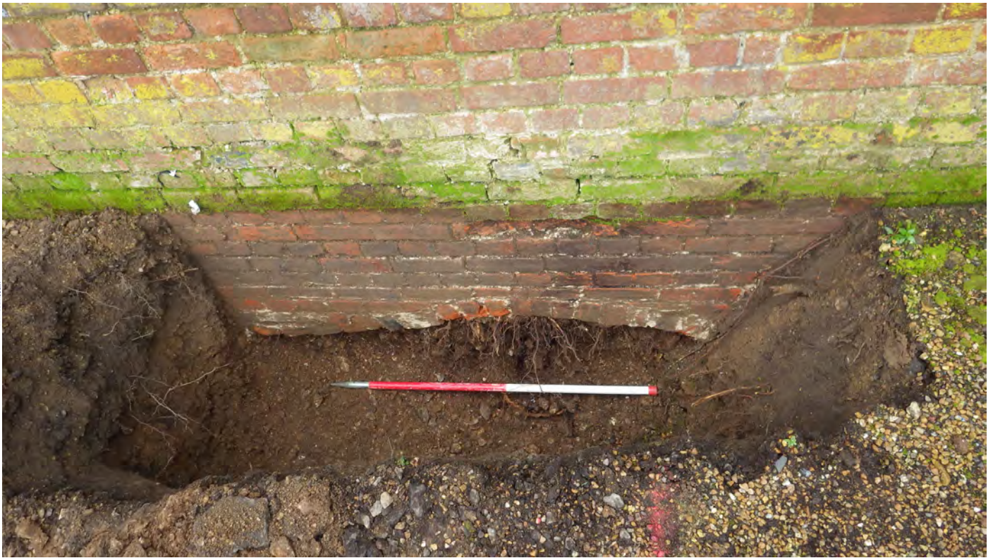
Plate 1: Foundation of boundary wall 6 exposed in Trench 3, showing brick arch
