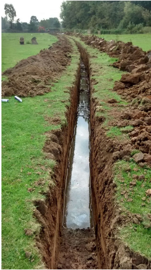
Plate 1: Field 1, general view, looking south
