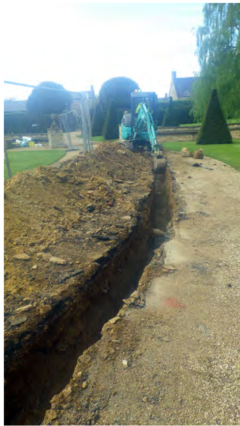
Plate 2: View north along area A.1
