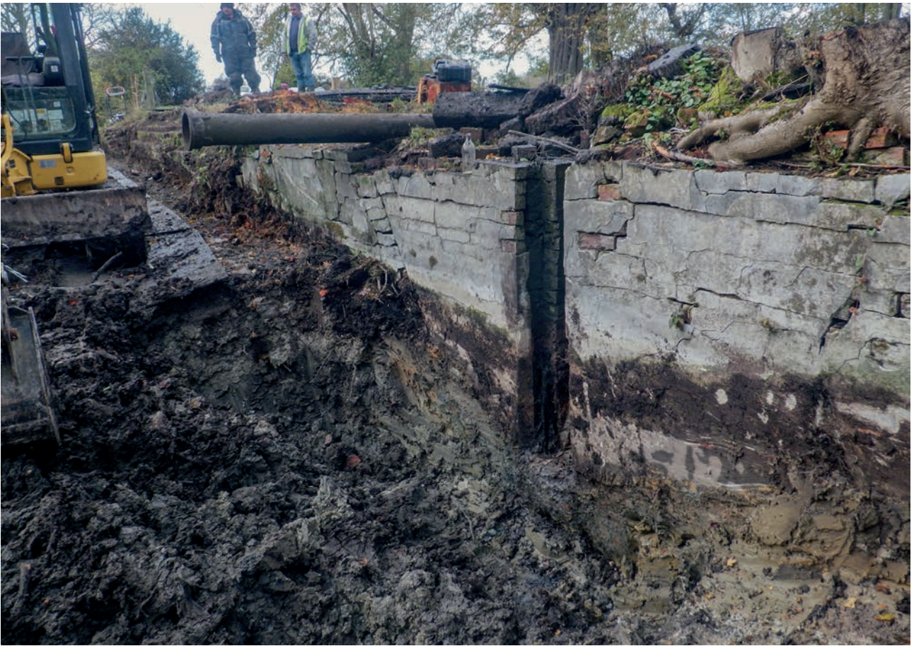
Plate 3: Deposit removed during dredging works
