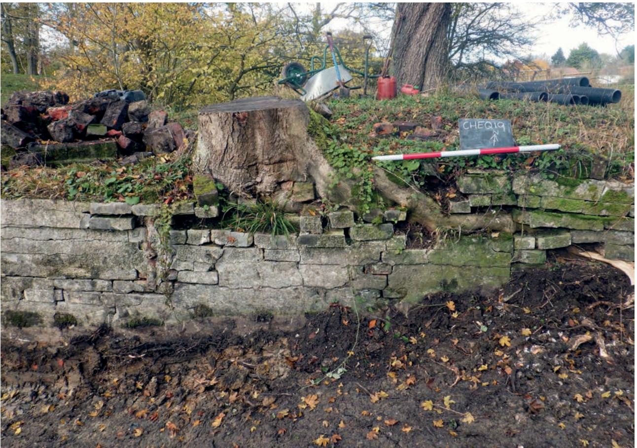
Plate 4: Root disturbance at eastern end of dam wall
