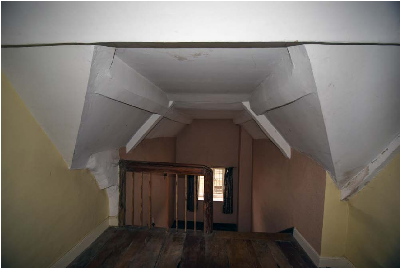
Plate 24: The ceiling of the stair turret, looking west
