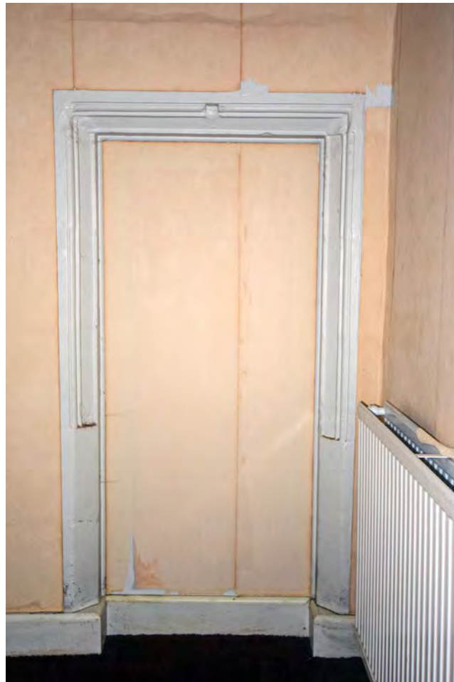
Plate 28: Bedroom 1, looking east
