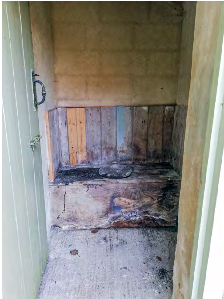
Plate 47: Small outhouse on the north side of the cottage, looking west
