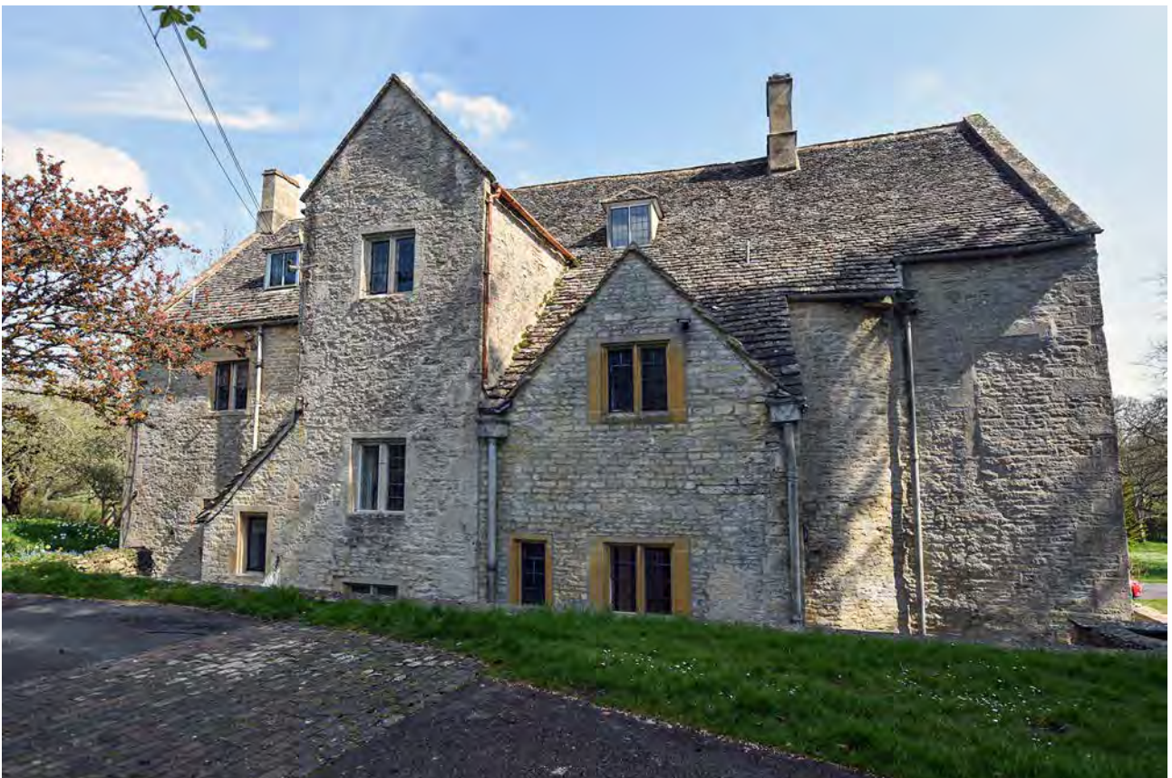
Plate 4: The west elevation of Aldsworth Manor, looking north-east
