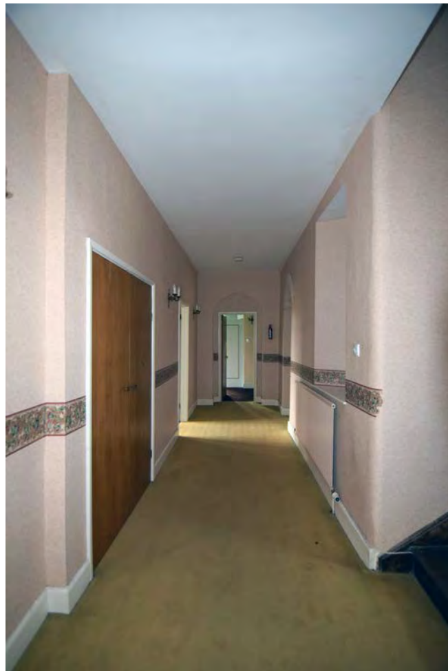
Plate 25: The first floor hallway, looking south
