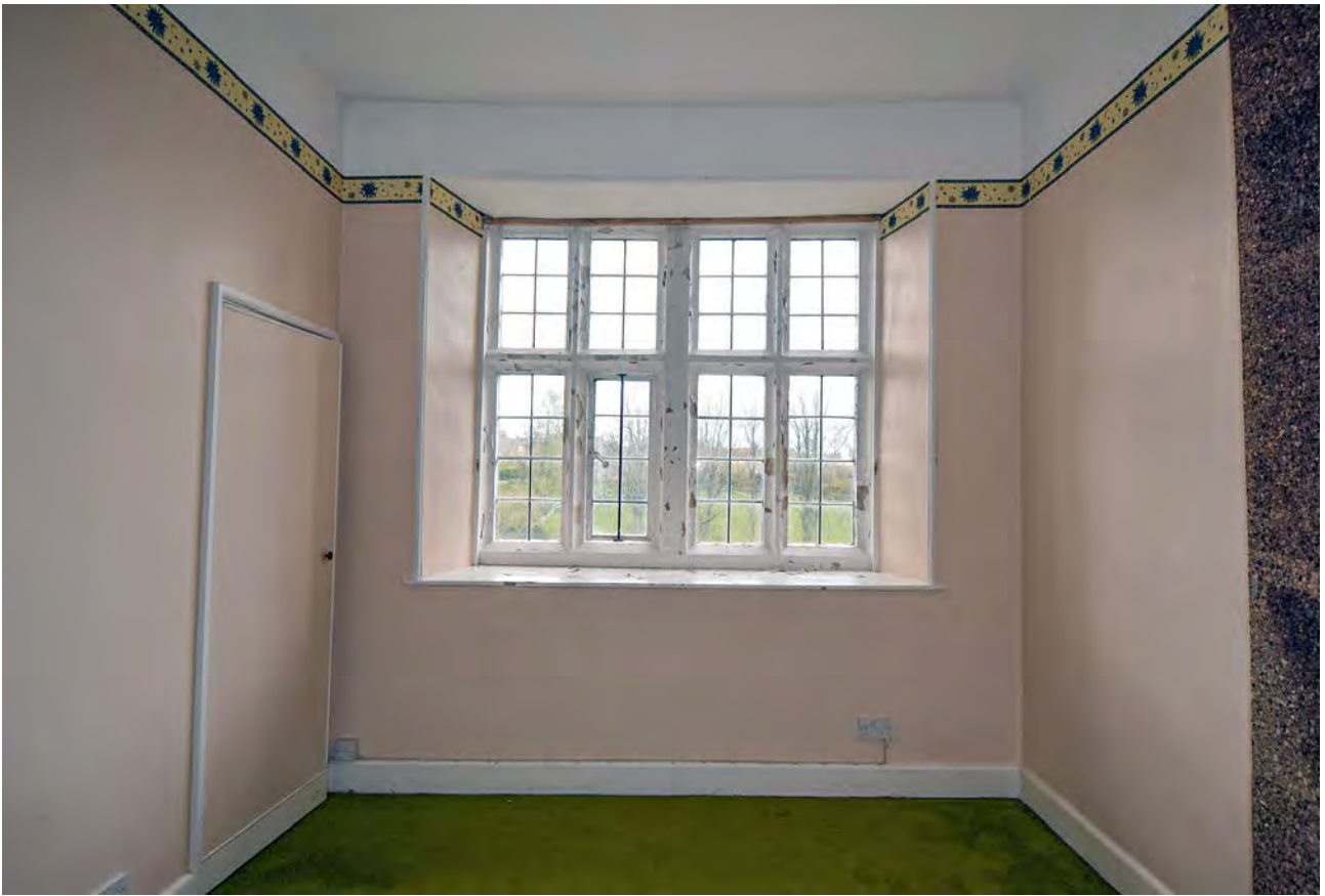
Plate 34: Bedroom 3, looking east
