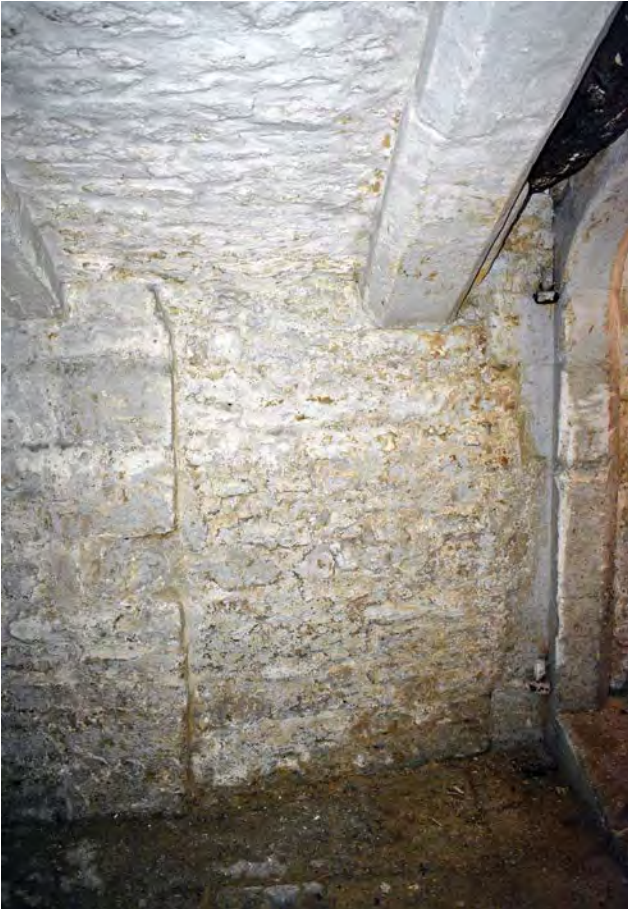
Plate 7: The north chamber of the cellar, looking west
