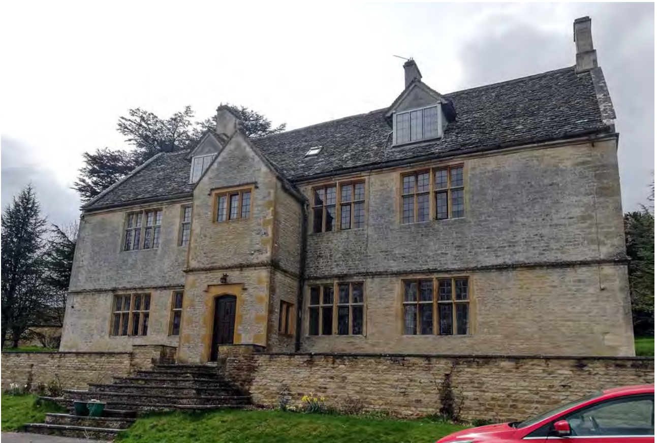
Plate 1: The east elevation of Aldsworth Manor, looking south-west
