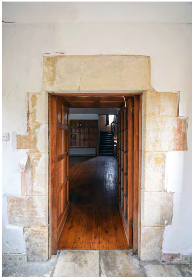
Plate 9: The ground floor of the porch tower, looking west
