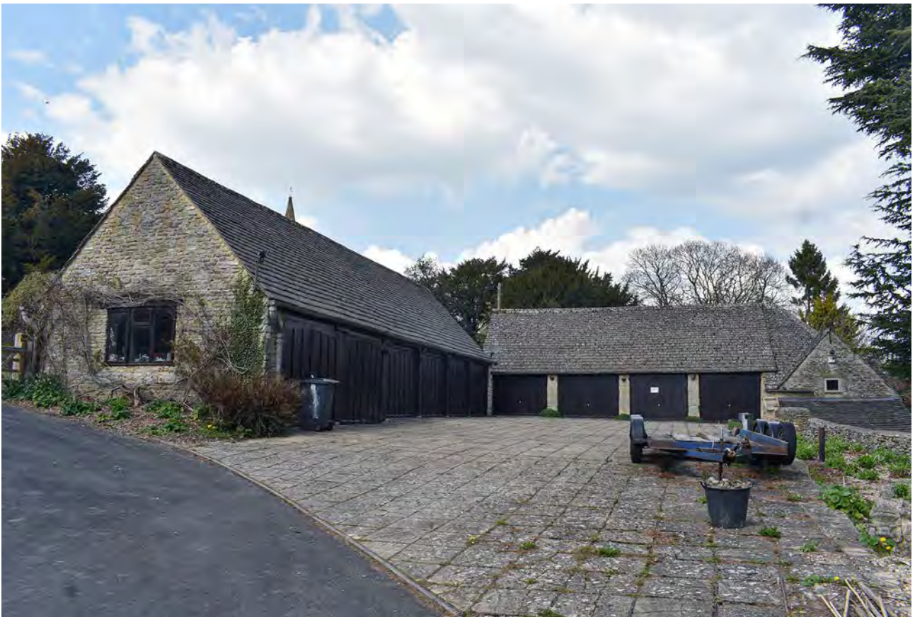
Plate 52: The garages, looking north
