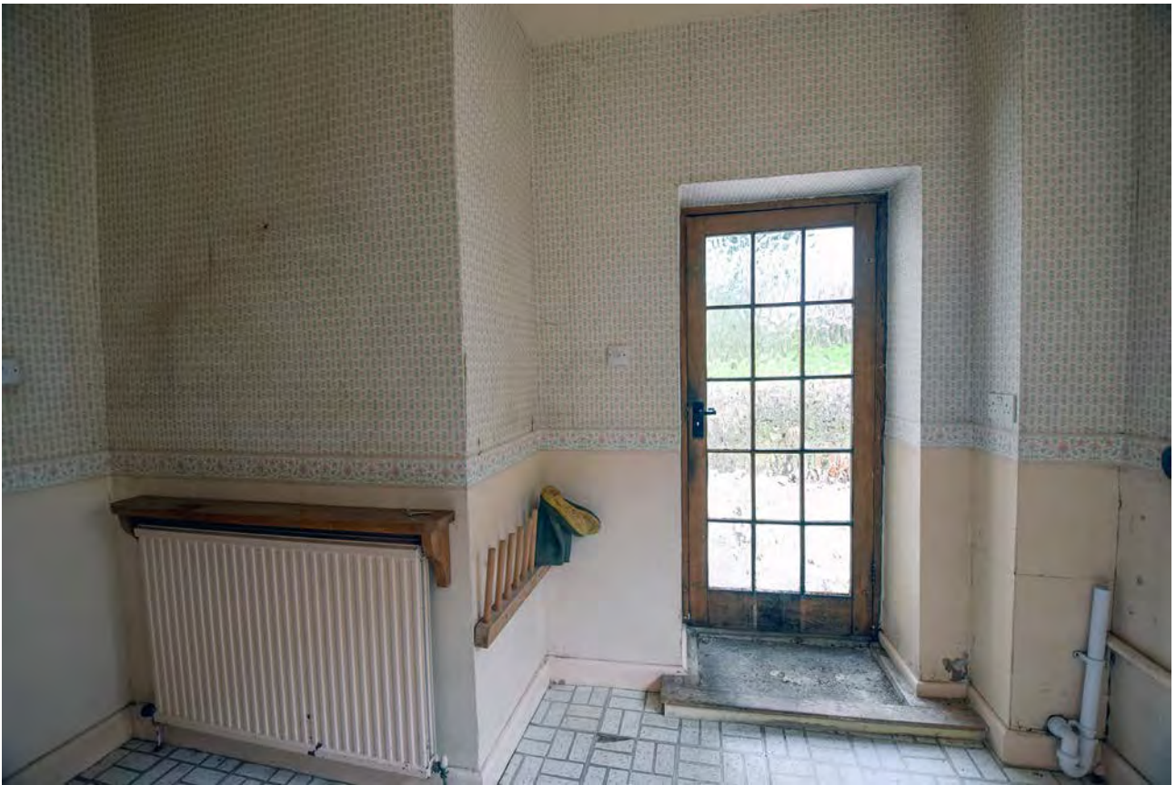
Plate 22: The back hall, looking south
