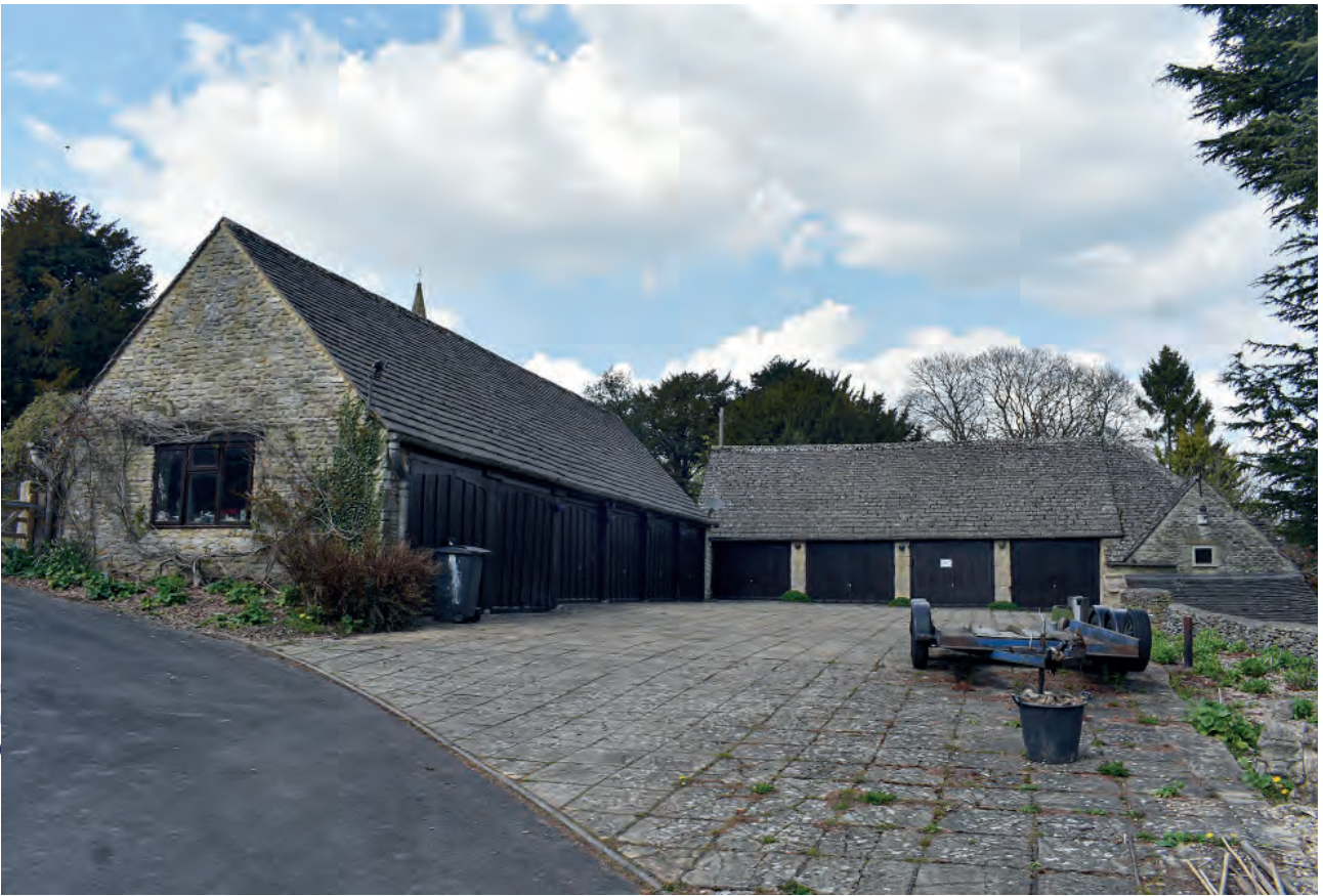
Plate 7: The garages, looking north
