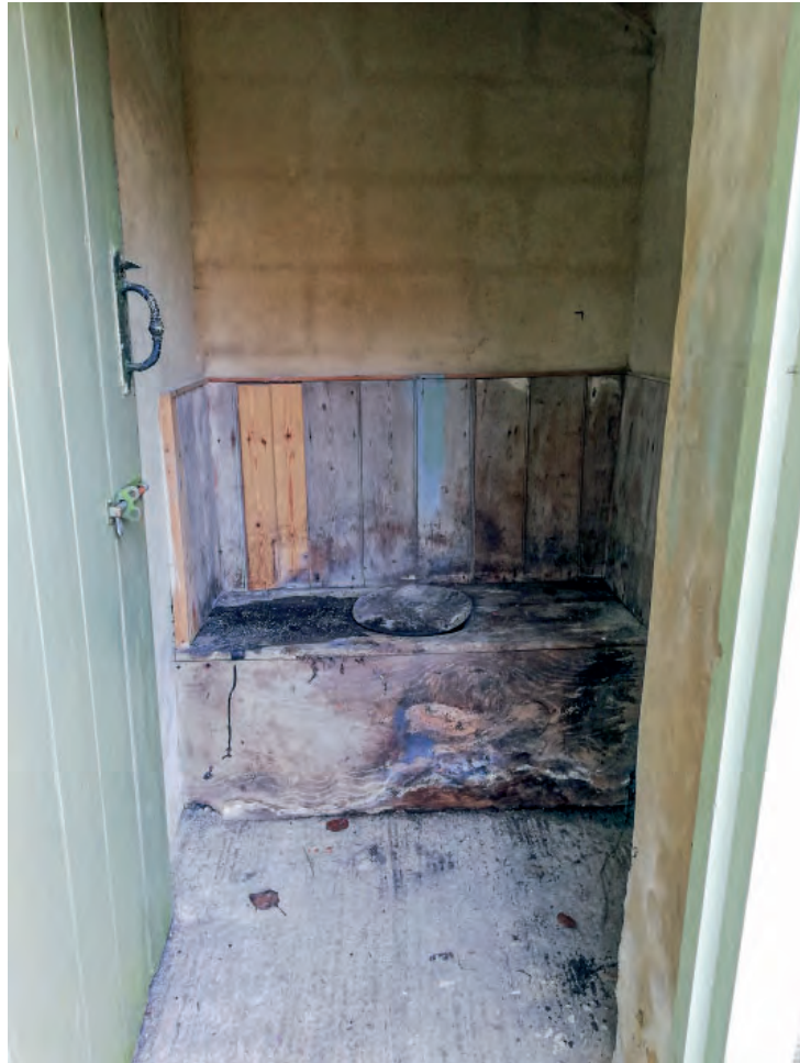
Plate 2: Small outhouse on the north side of the cottage, looking west
