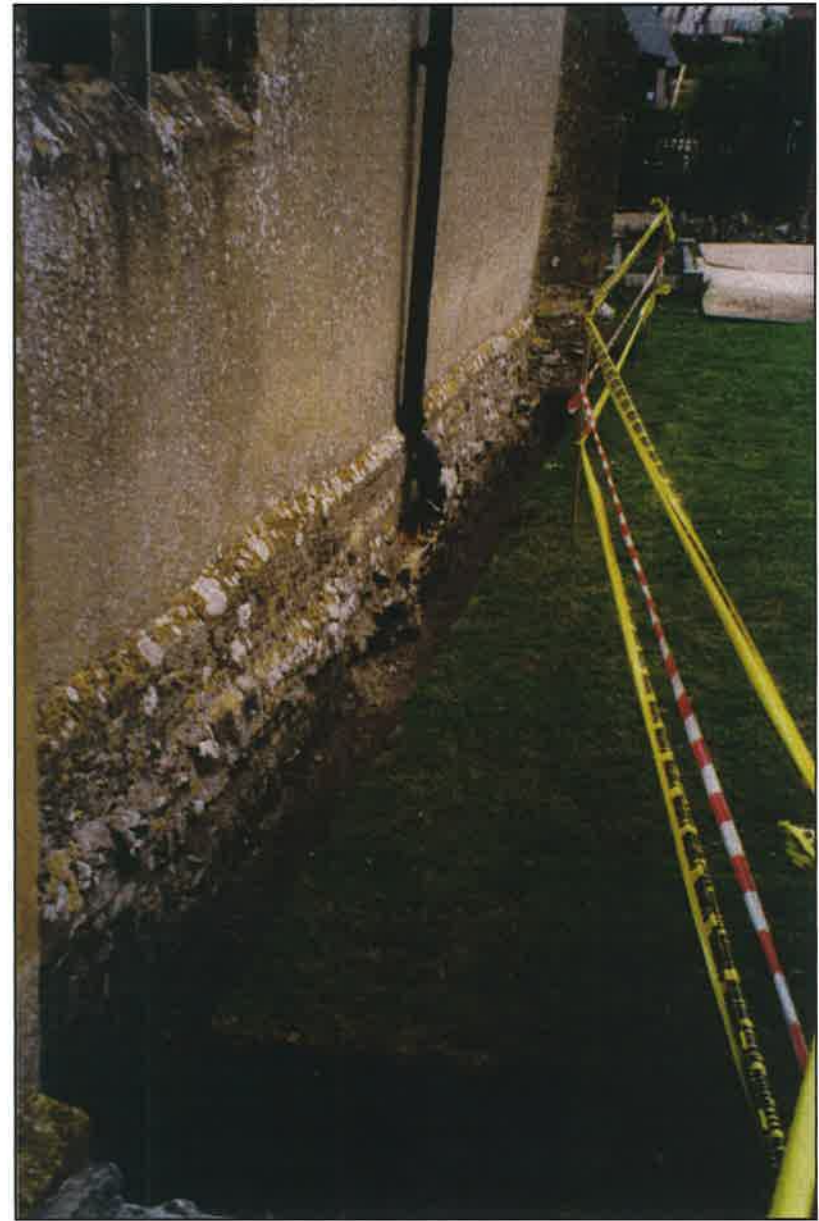
Plate 5: South wall looking east
