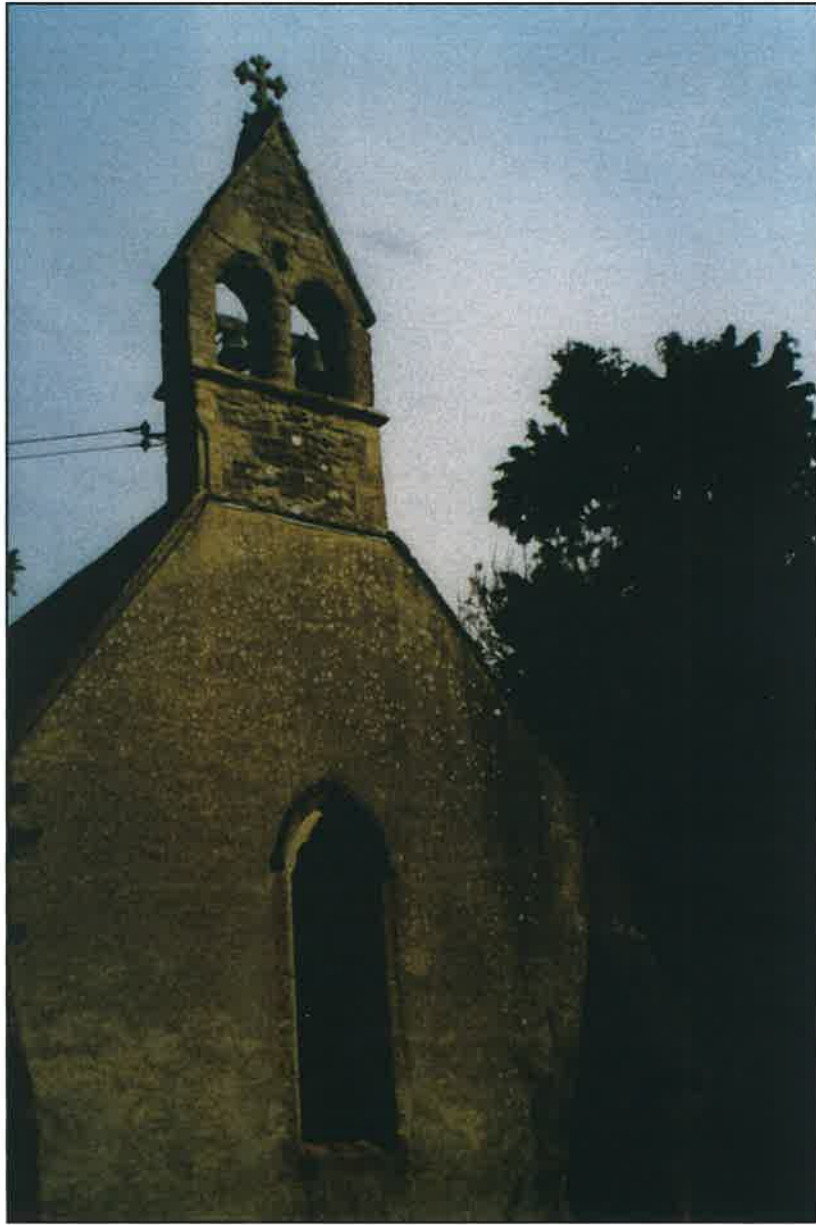
Plate 1: General view of west window and tower
