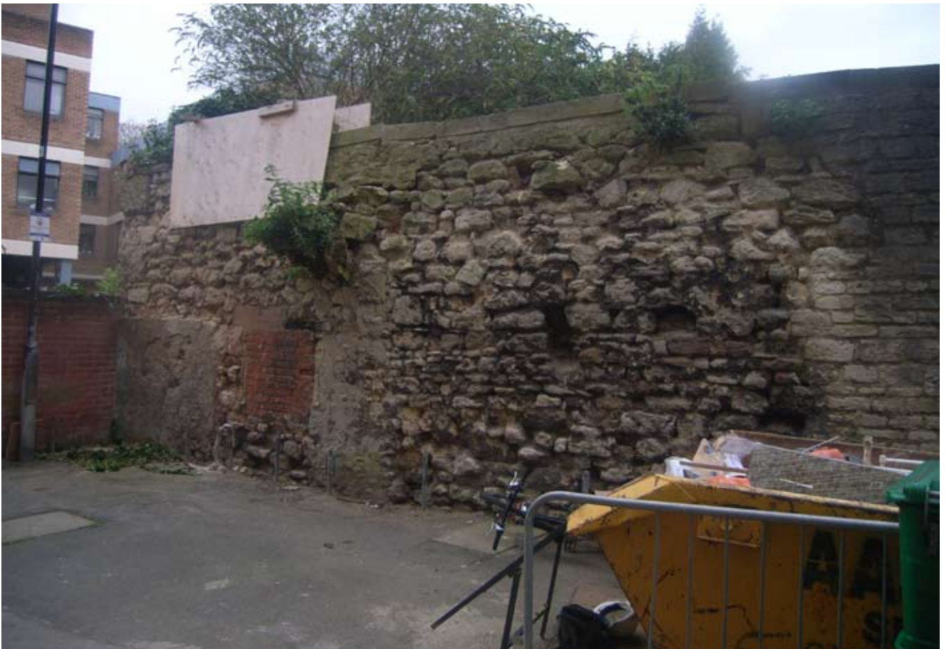
Plate 22: South wall of former malthouse on Rose Place
