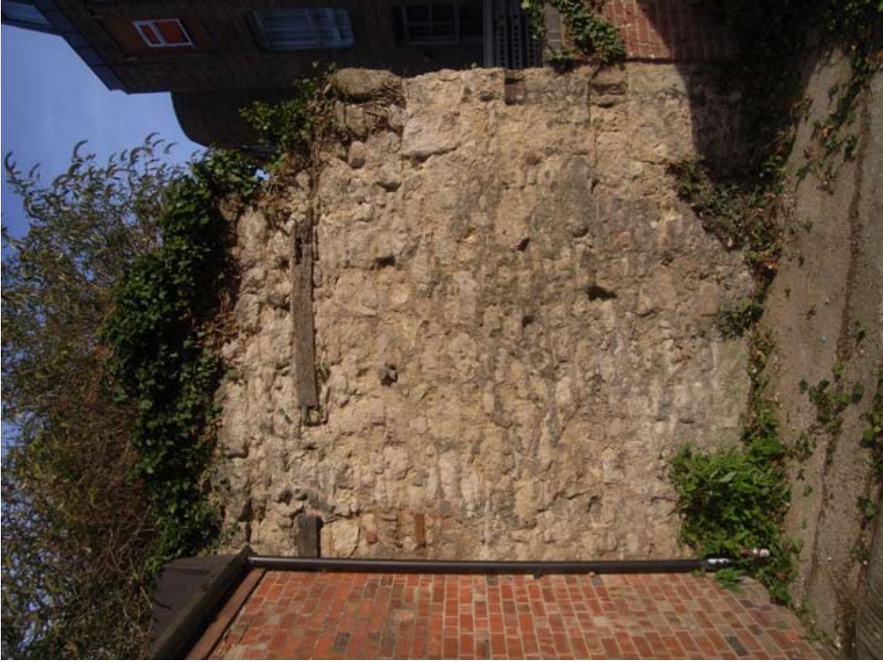
Plate 23: West elevation of former malthouse on Rose Place
