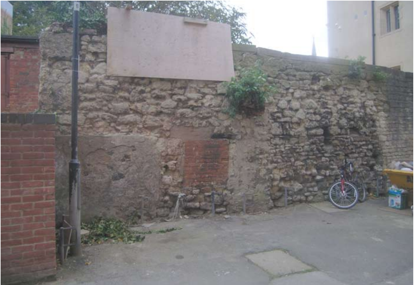
Plate 21: South wall of former malthouse on Rose Place
