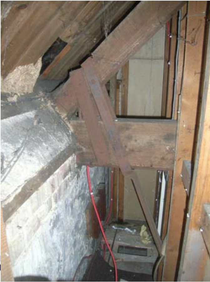
Plate 13: End of tie-beam in 6 Brewer St.
