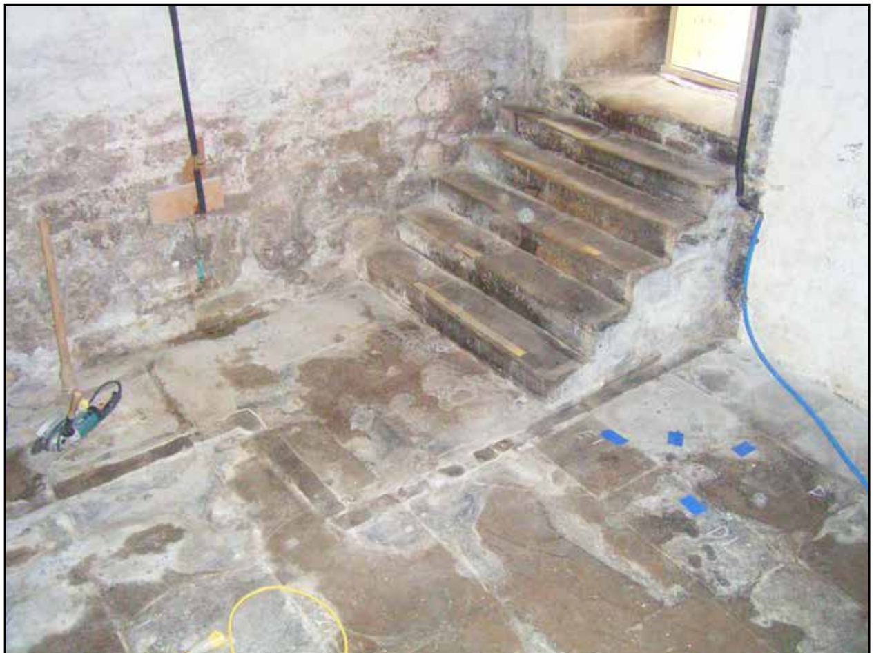
Plate 6. North entrance steps
