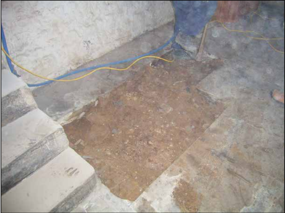
Plate 11. Foundation Pad 2 during excavation
