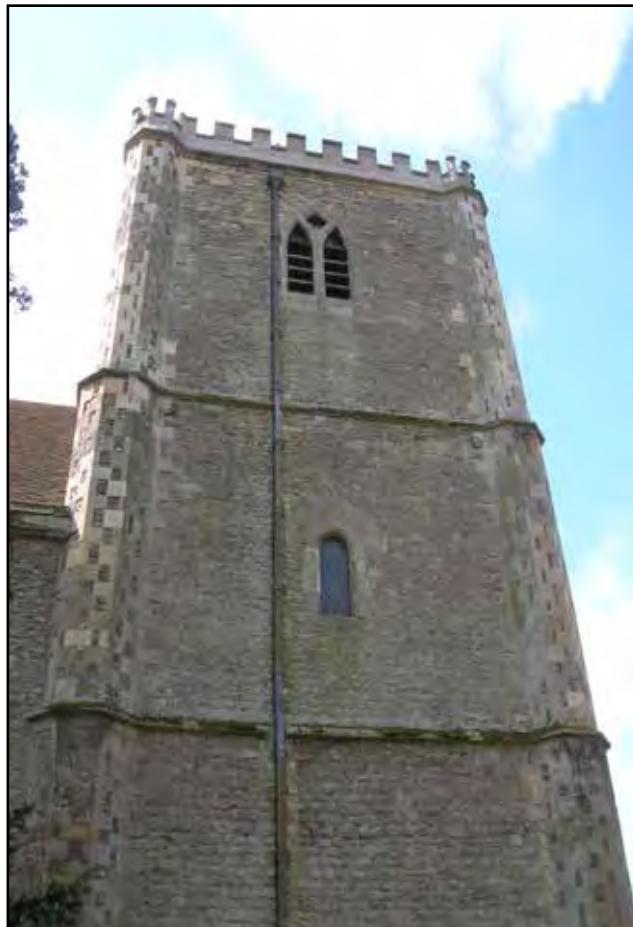
Plate 32. North elevation of outside of Tower, upper view
