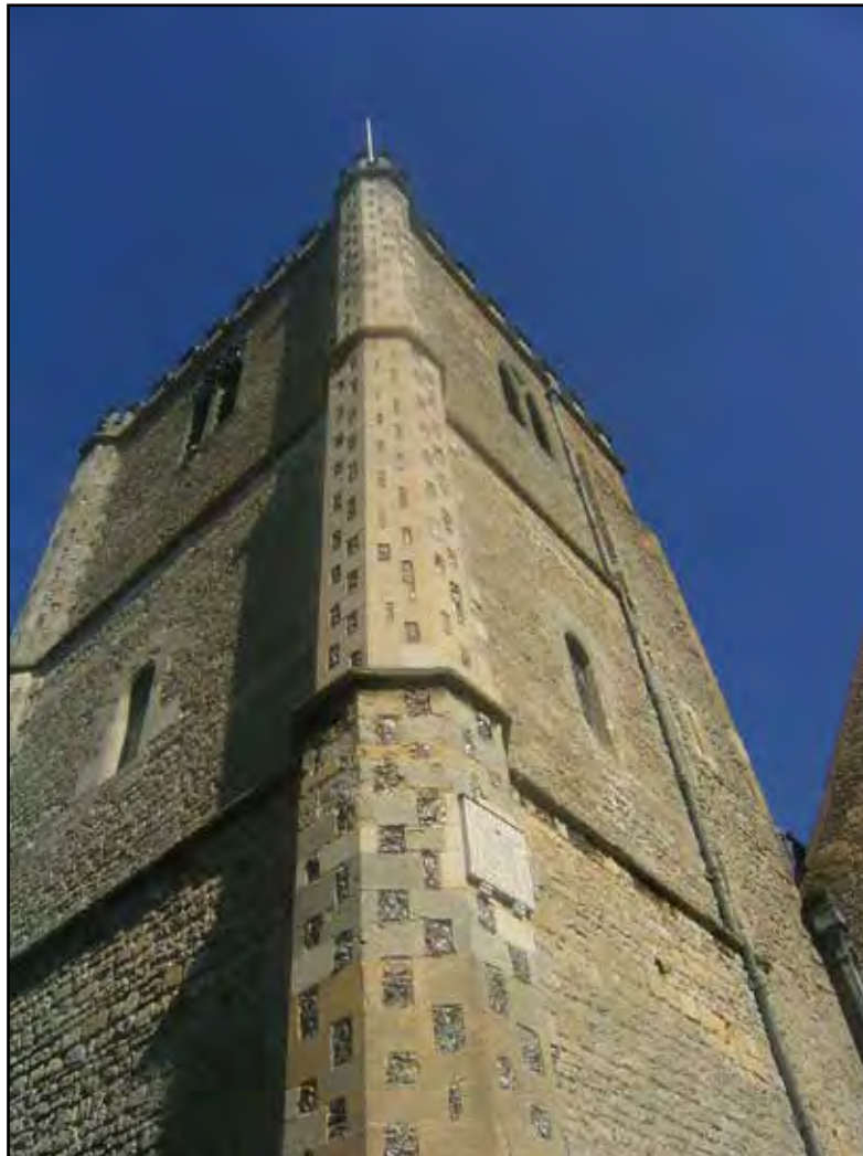
Plate 30. West elevation of outside of Tower, upper view
