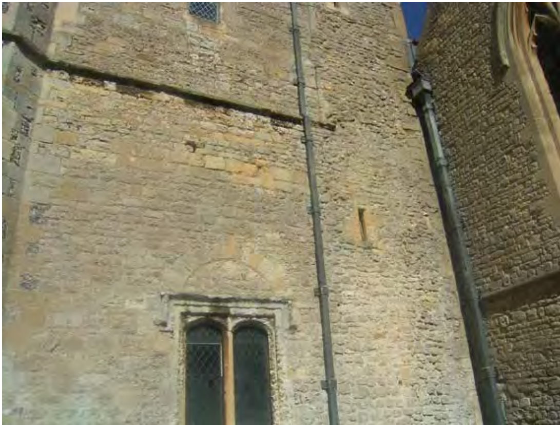
Plate 28. South elevation of outside of tower, upper view
