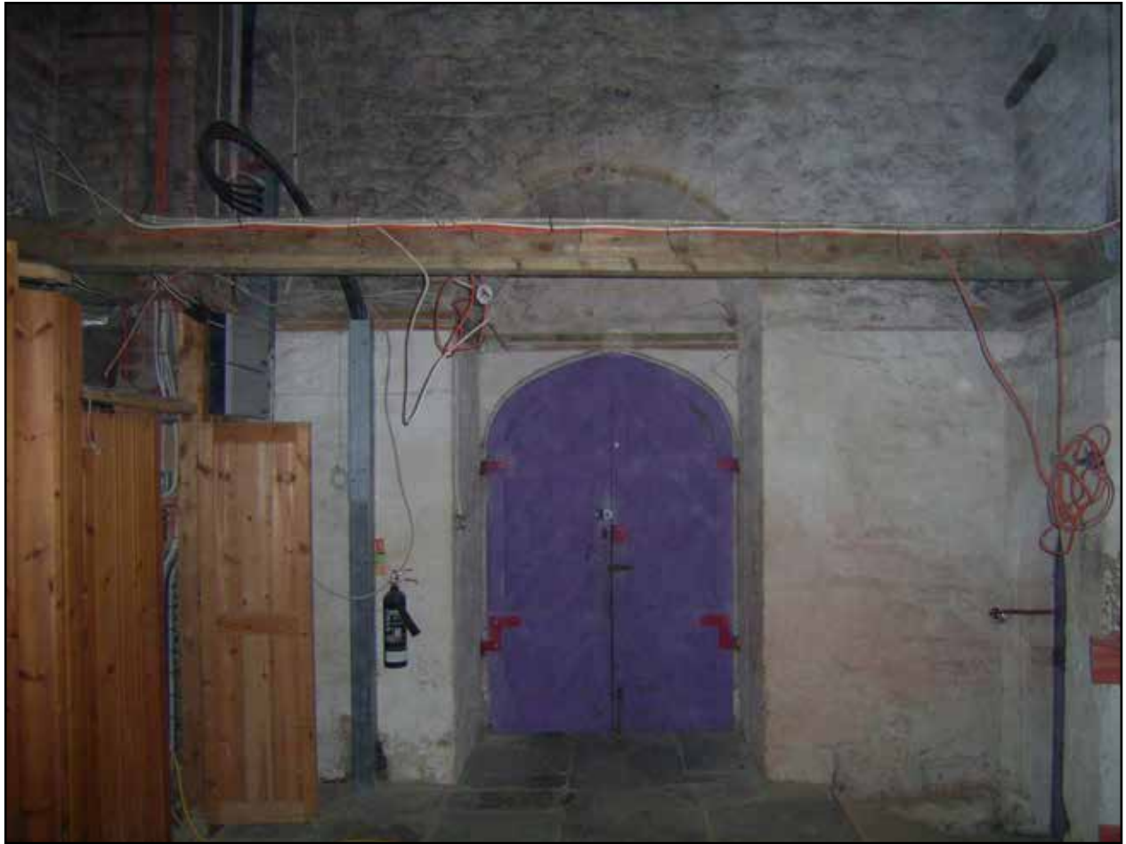
Plate 1. East Elevation of Tower
