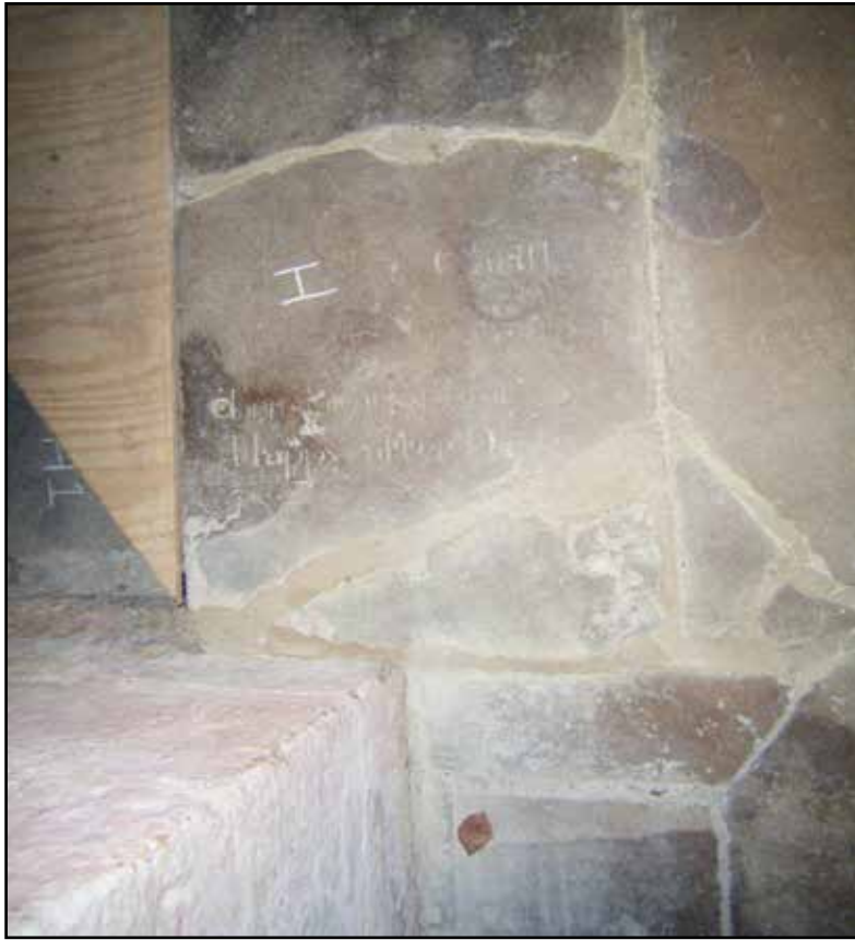
Plate 21. Grave slab flagstone in Foundation Pad 6
