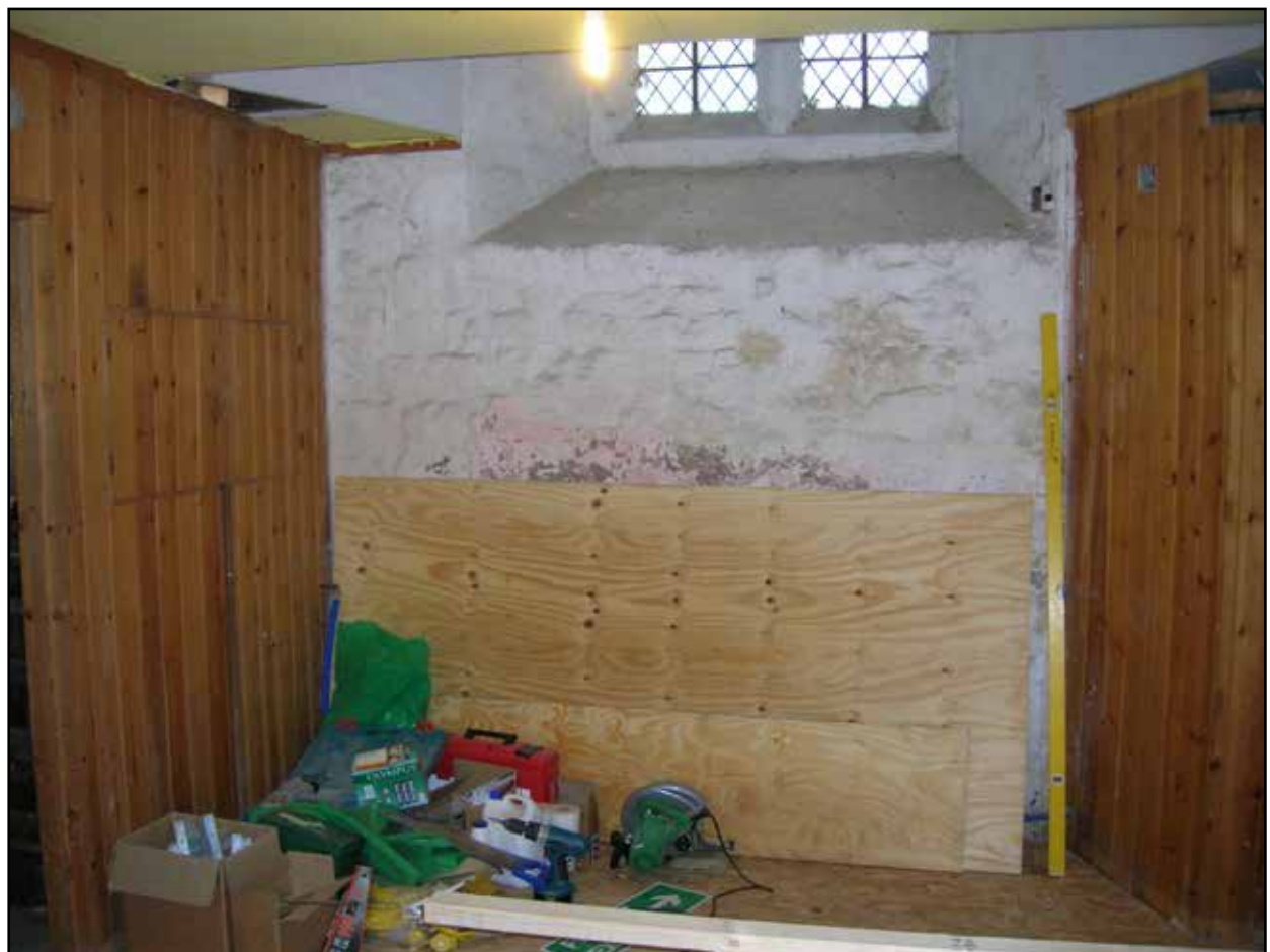
Plate 4. North Elevation of Tower
