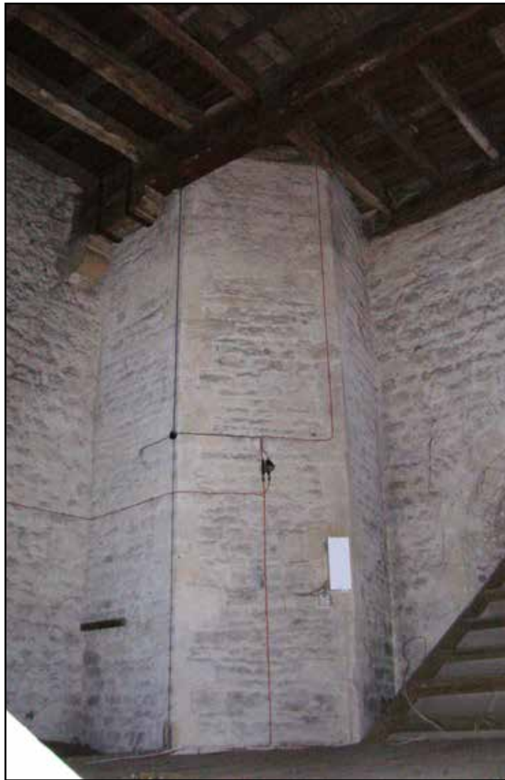
Plate 7. Timber ceiling before erection of new floors
