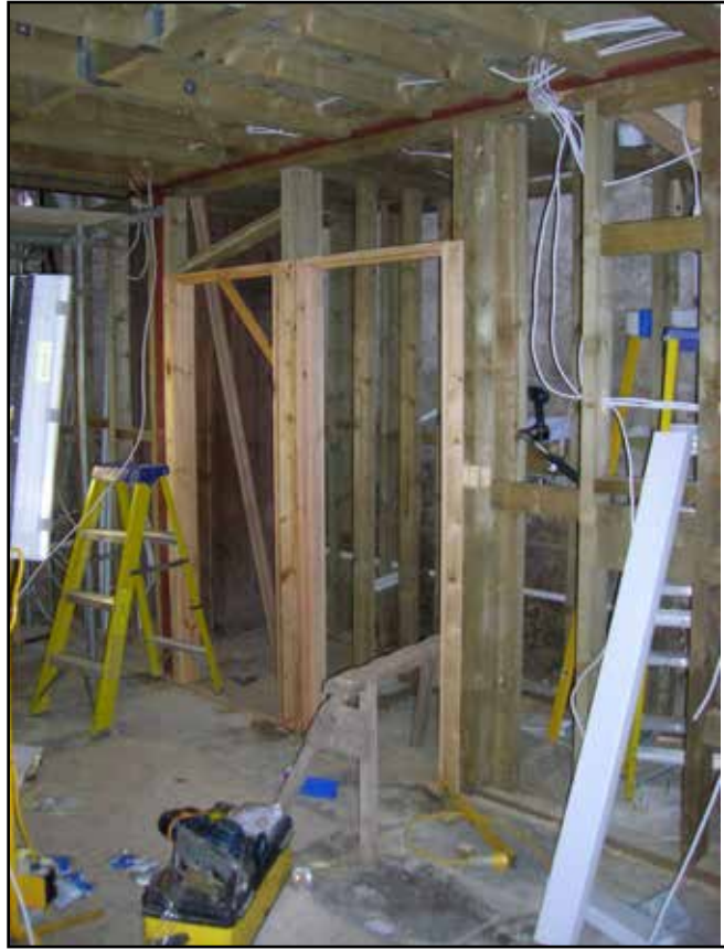
Plate 23. Erection of new interior
