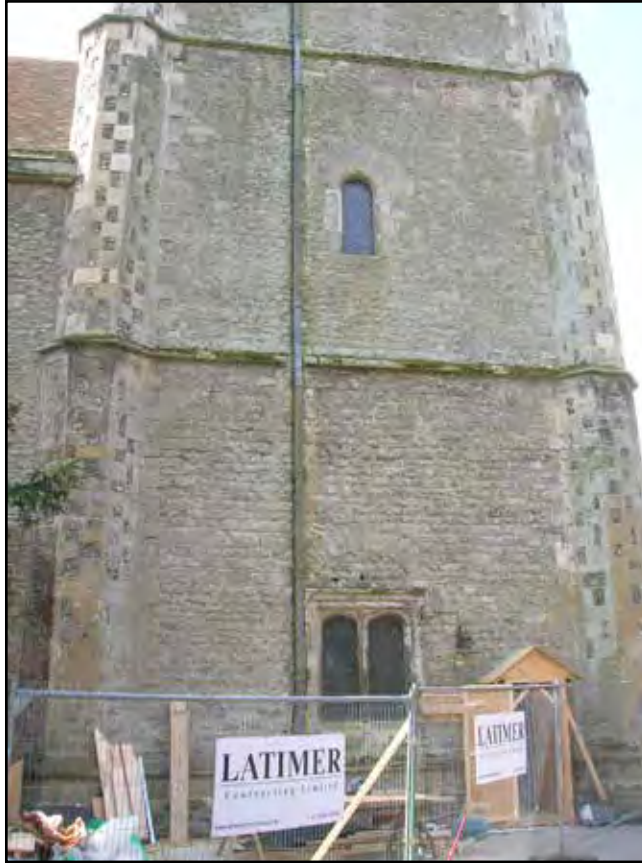
Plate 31. North elevation of outside of Tower, lower view
