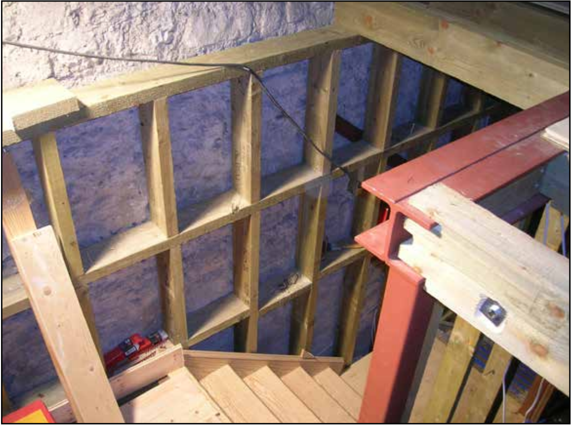
Plate 25. Staircase to new floors
