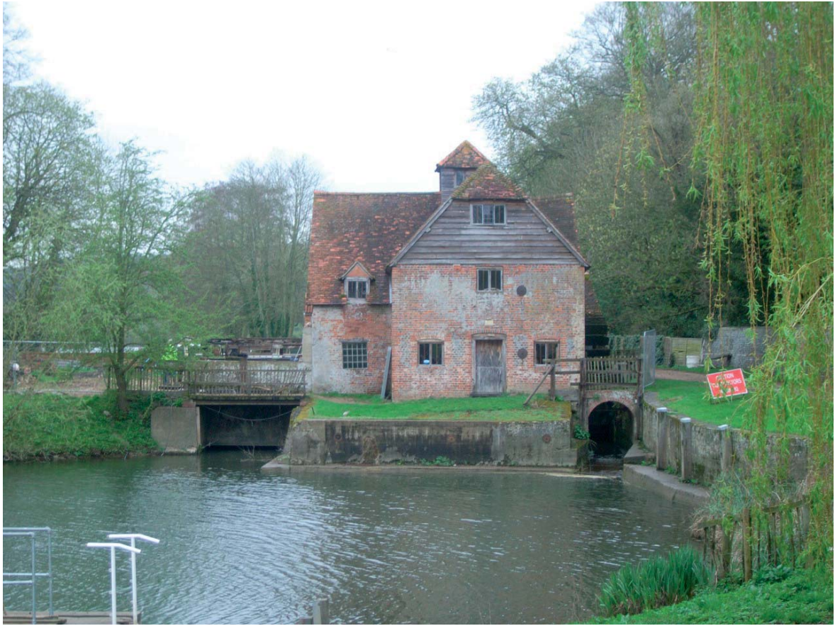
Plate 1: South-east elevation of Mapledurham Mill, with the southern turbine chamber and mill race to the left
