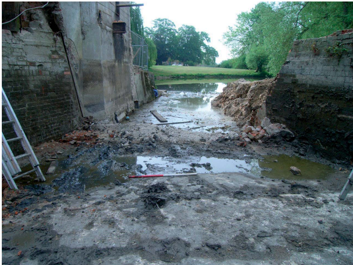
Plate 4: Southern mill rail following demolition of 1922 turbine
