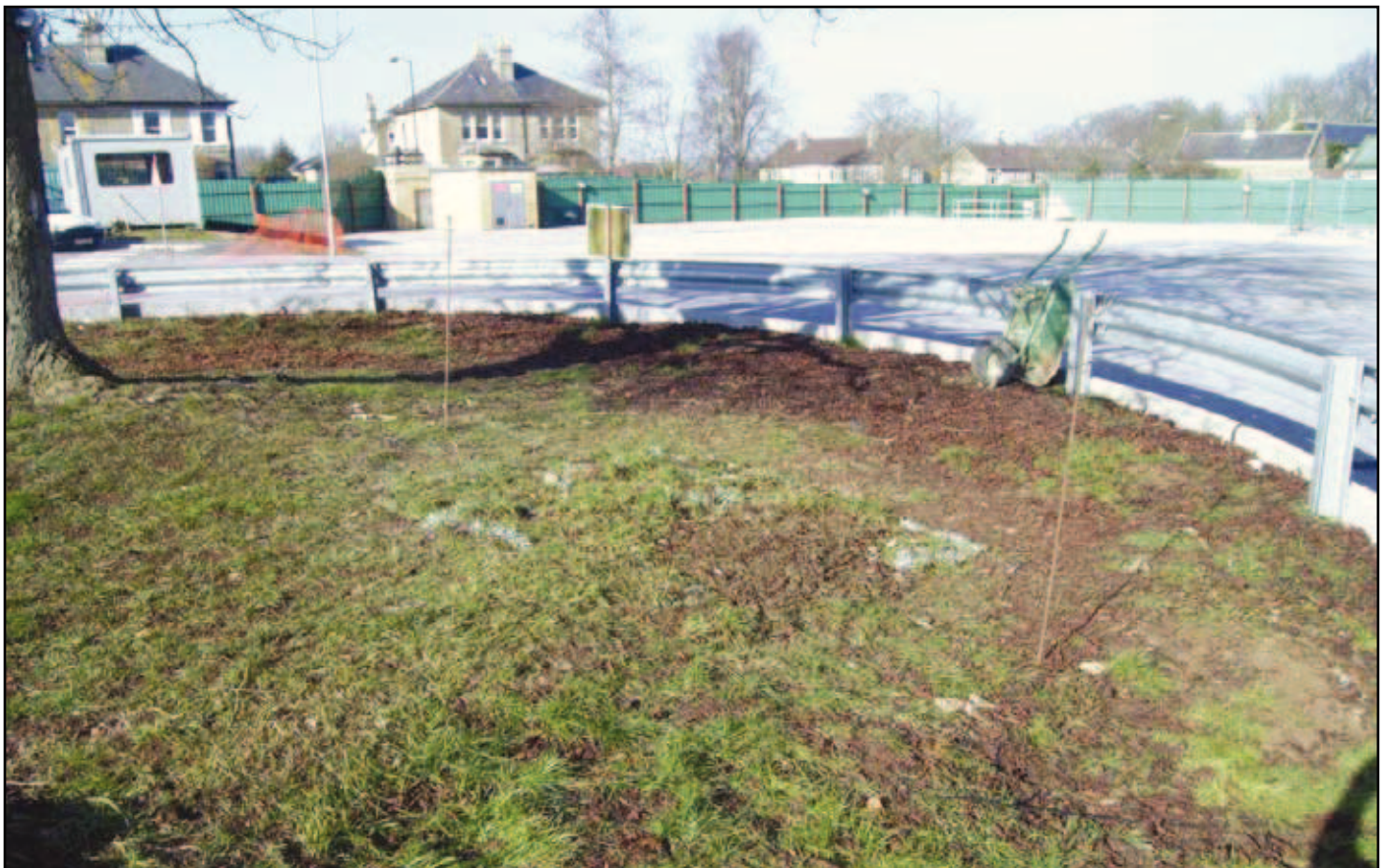
Plate 4: Trial pit 2. (After reinstatement) showing current disposition of the site
