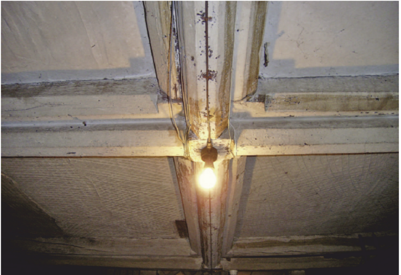
Plate 14: Applied mouldings in roof structure of Area 2, facing west
