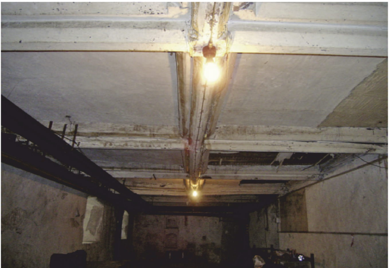
Plate 12: Roof Structure in Area 2, facing west
