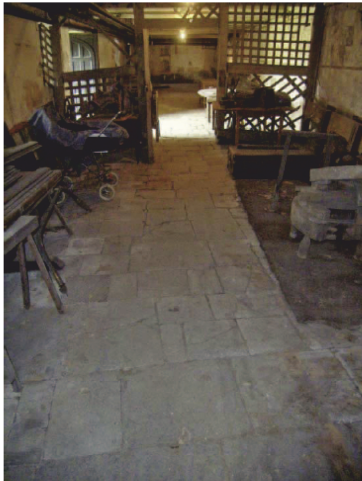
Plate 26: Flagstone floor in Area 3, facing east
