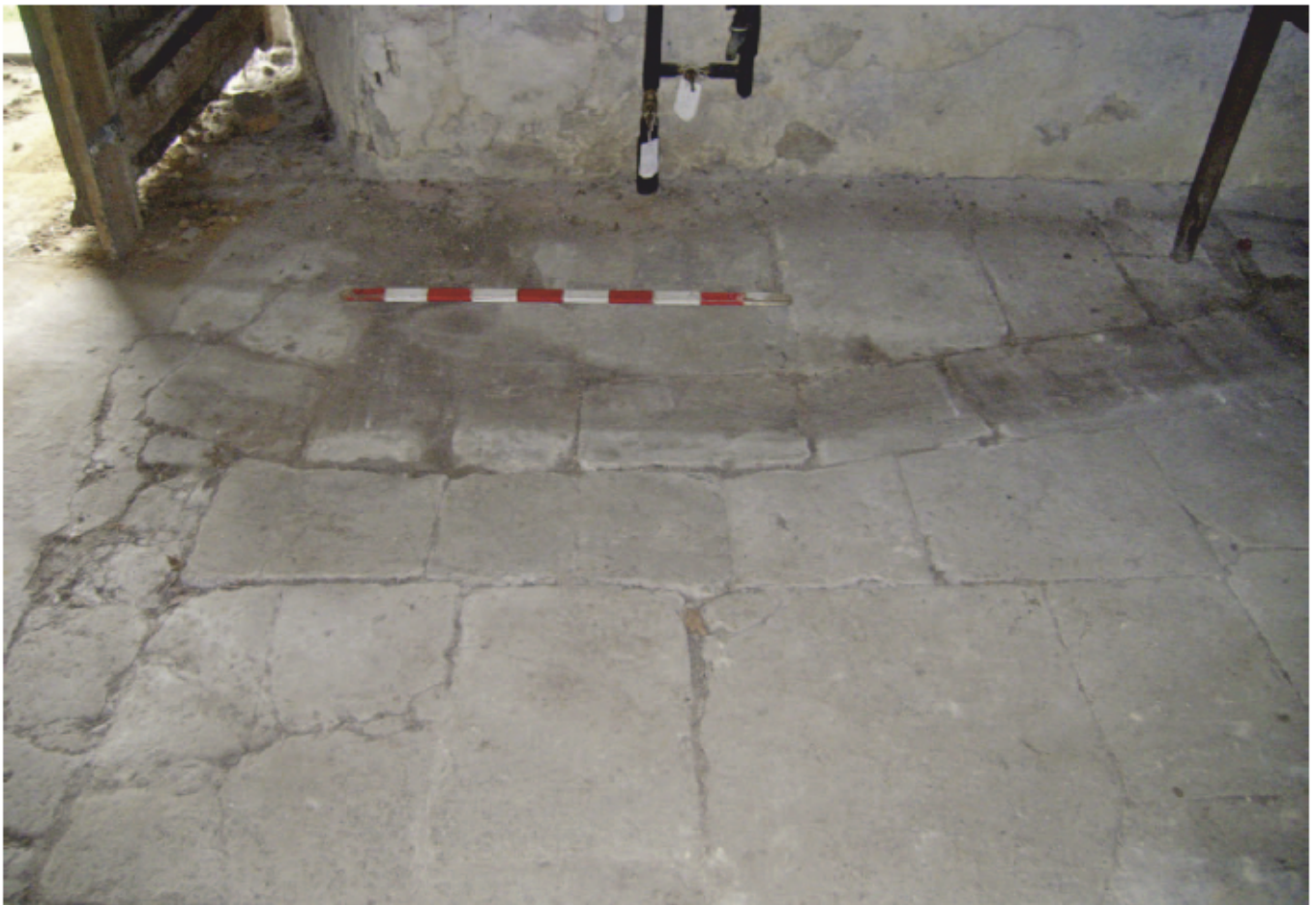
Plate 11: Drain in north side of floor in Area 2, facing north
