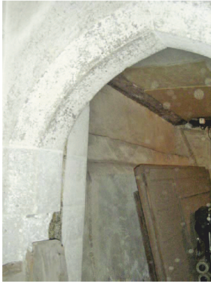
Plate 33: Chamfer on dooray in east wall of Area 4, facing south west
