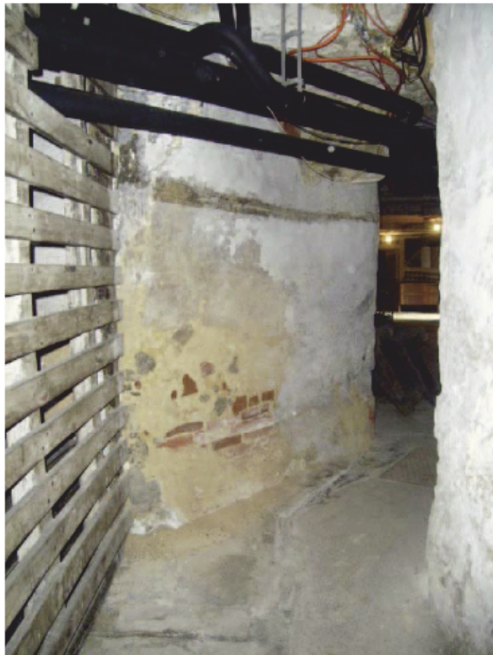
Plate 4: Passage leading from Area 1 to Area 2, facing west
