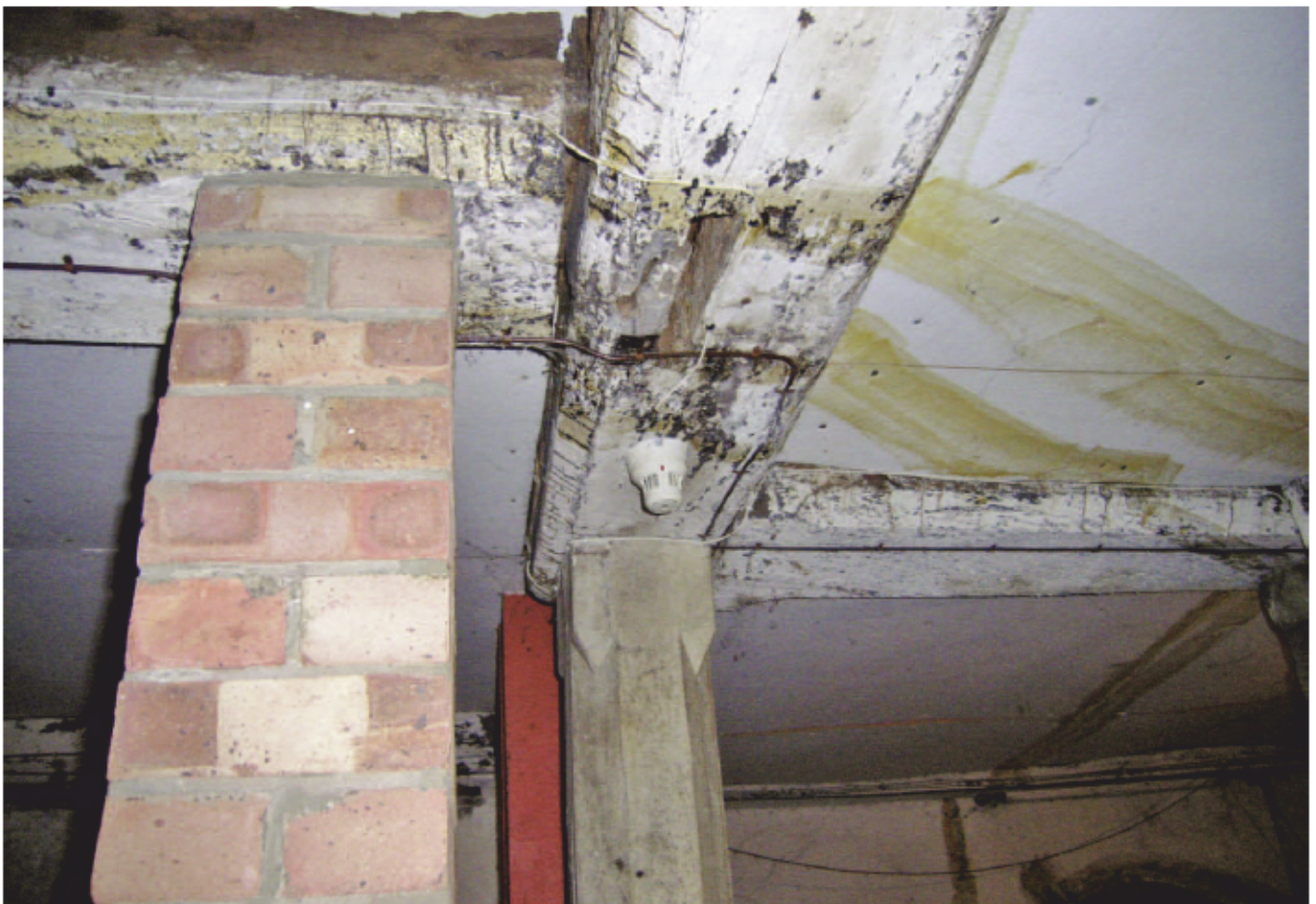
Plate 28: Brick and wood supports for roof structure in Bay 12 of Area 3
