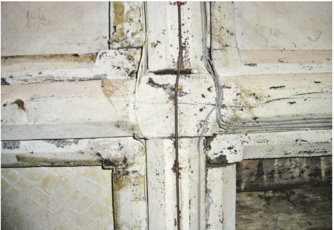
Plate 15: Applied mouldings in roof structure of Area 2
