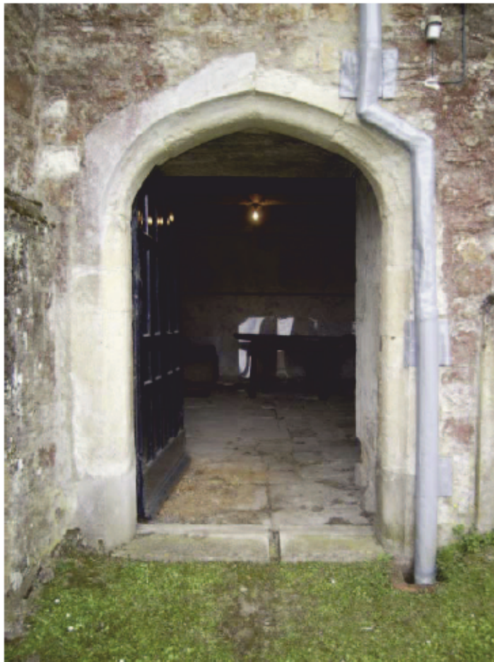
Plate 8: Doorway leading from Queen's Court to Area 2 of Cellars
