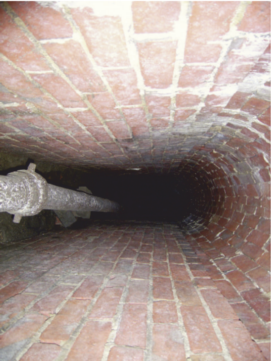
Plate 35: Drain running from east side of Area 4 under Stone Court
