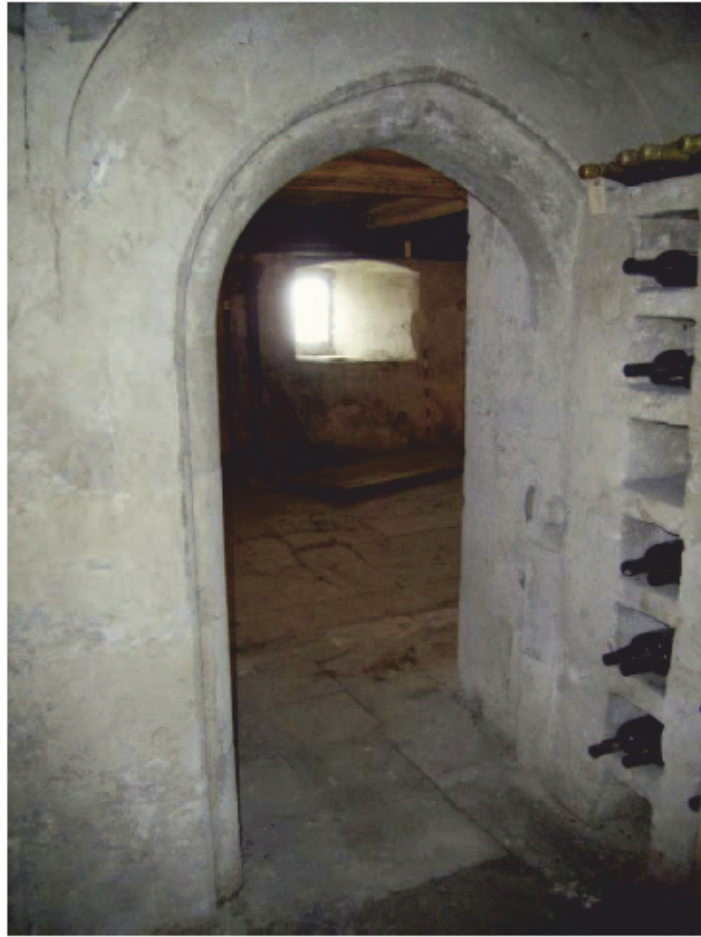
Plate 21: Doorway of Wine Cellar, facing north
