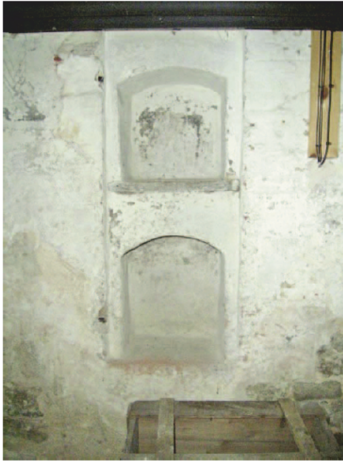
Plate 7: Cupboards in east wall of Area 2
