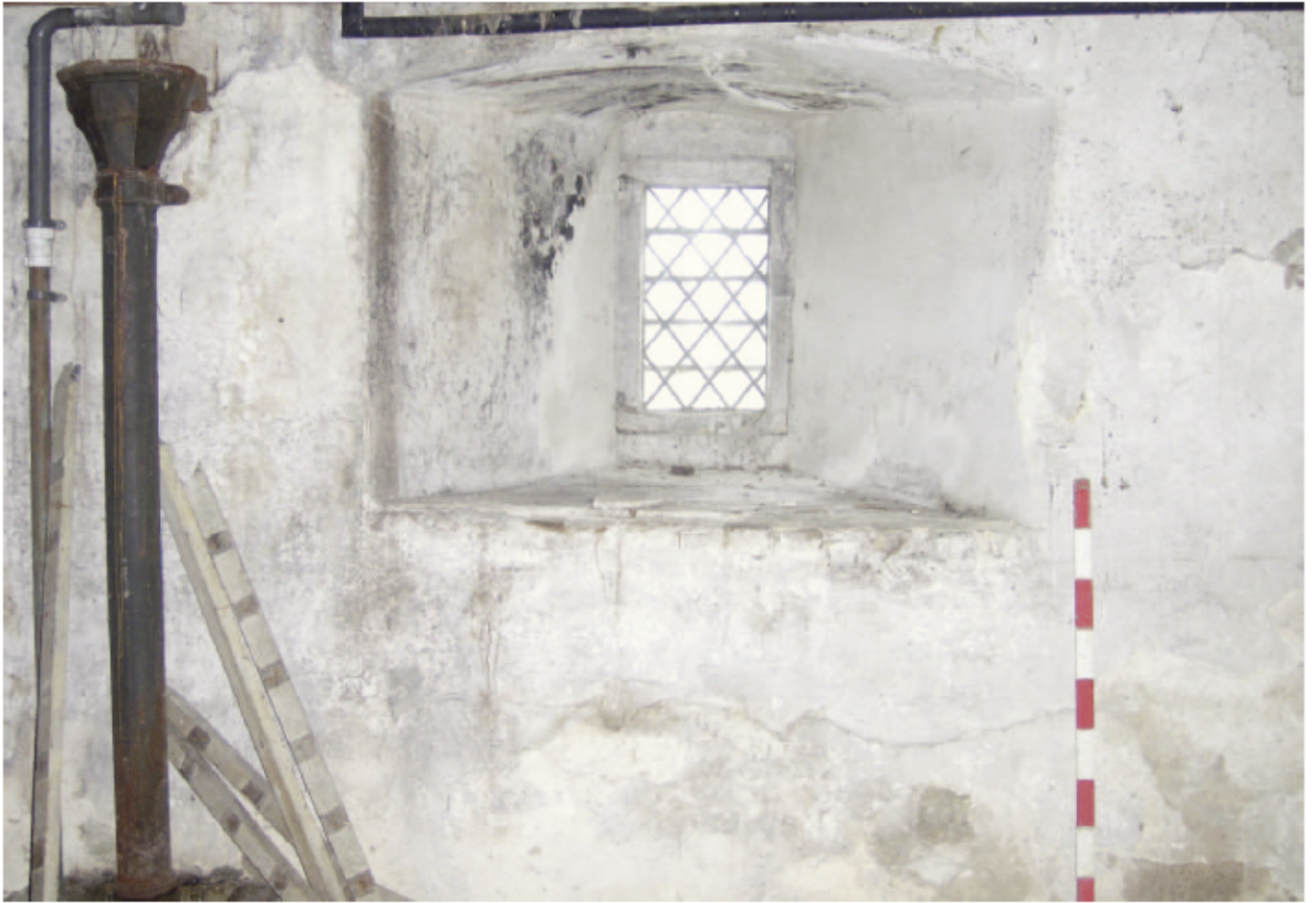
Plate 9: Window in North wall of Area 2
