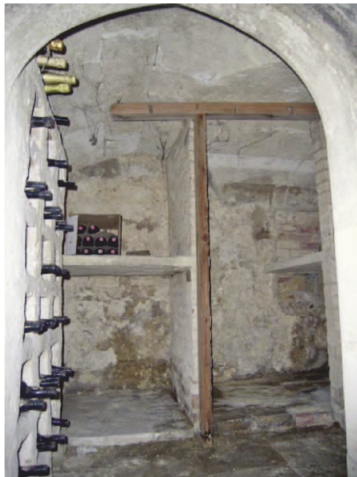
Plate 18: Doorway and south wall of Wine Cellar, facing south
