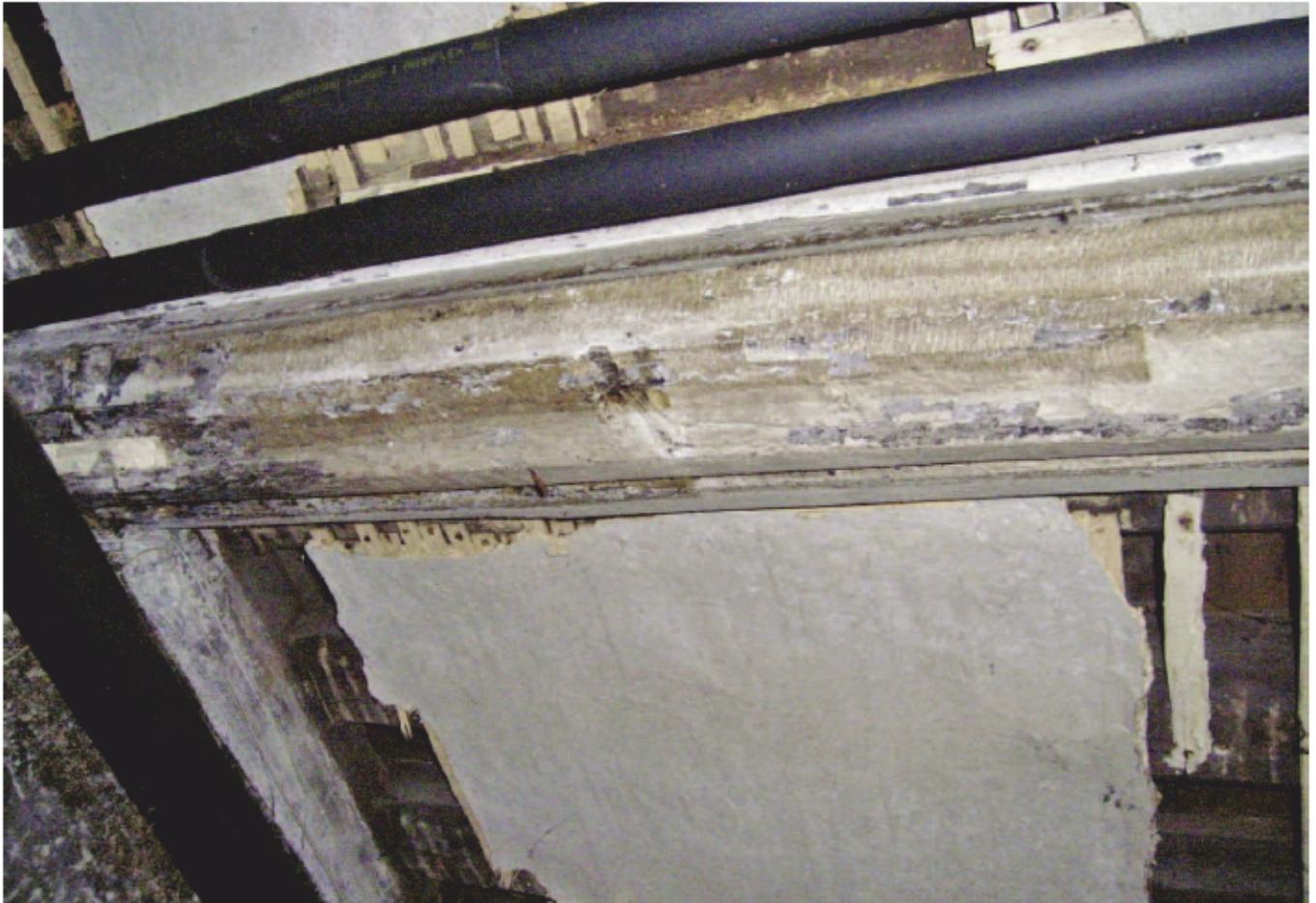
Plate 17: Transverse Beam 1 in Bay 1 of Area 2
