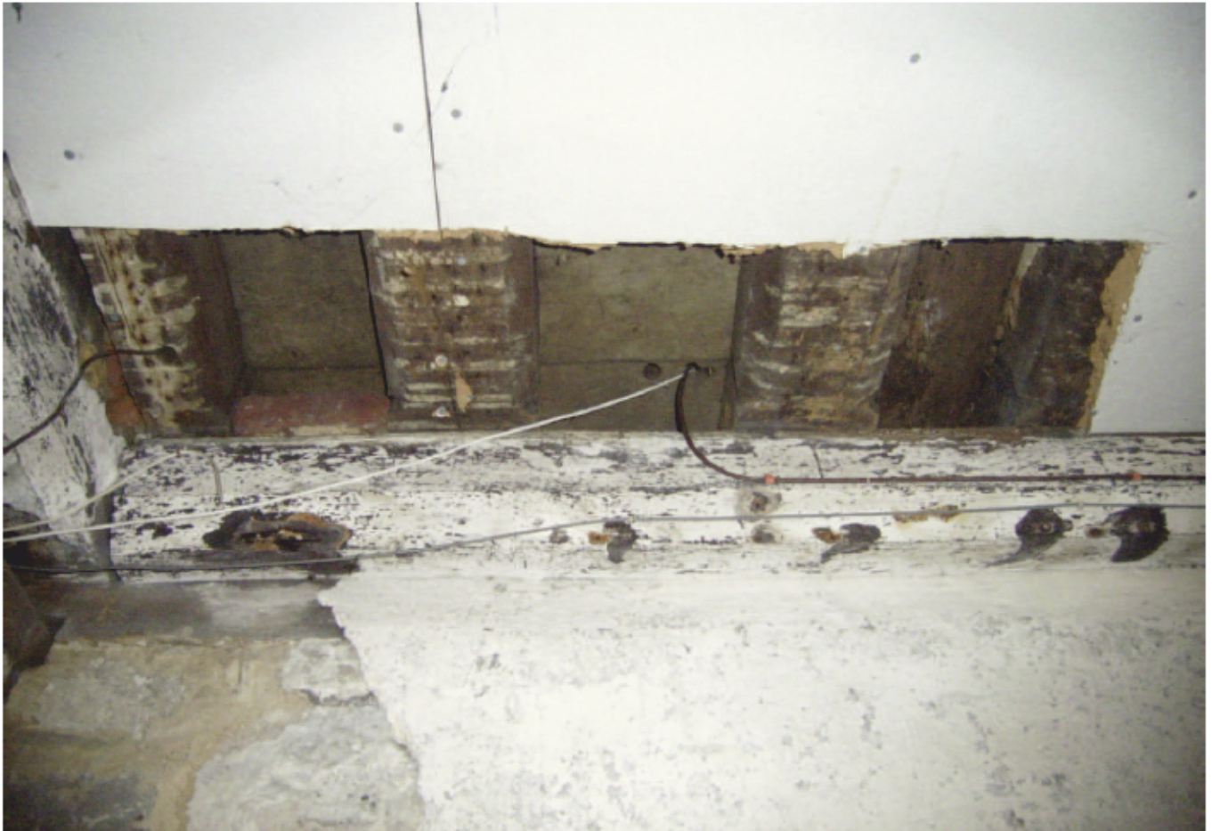
Plate 16: Chamfered common joists in Area 2, facing south
