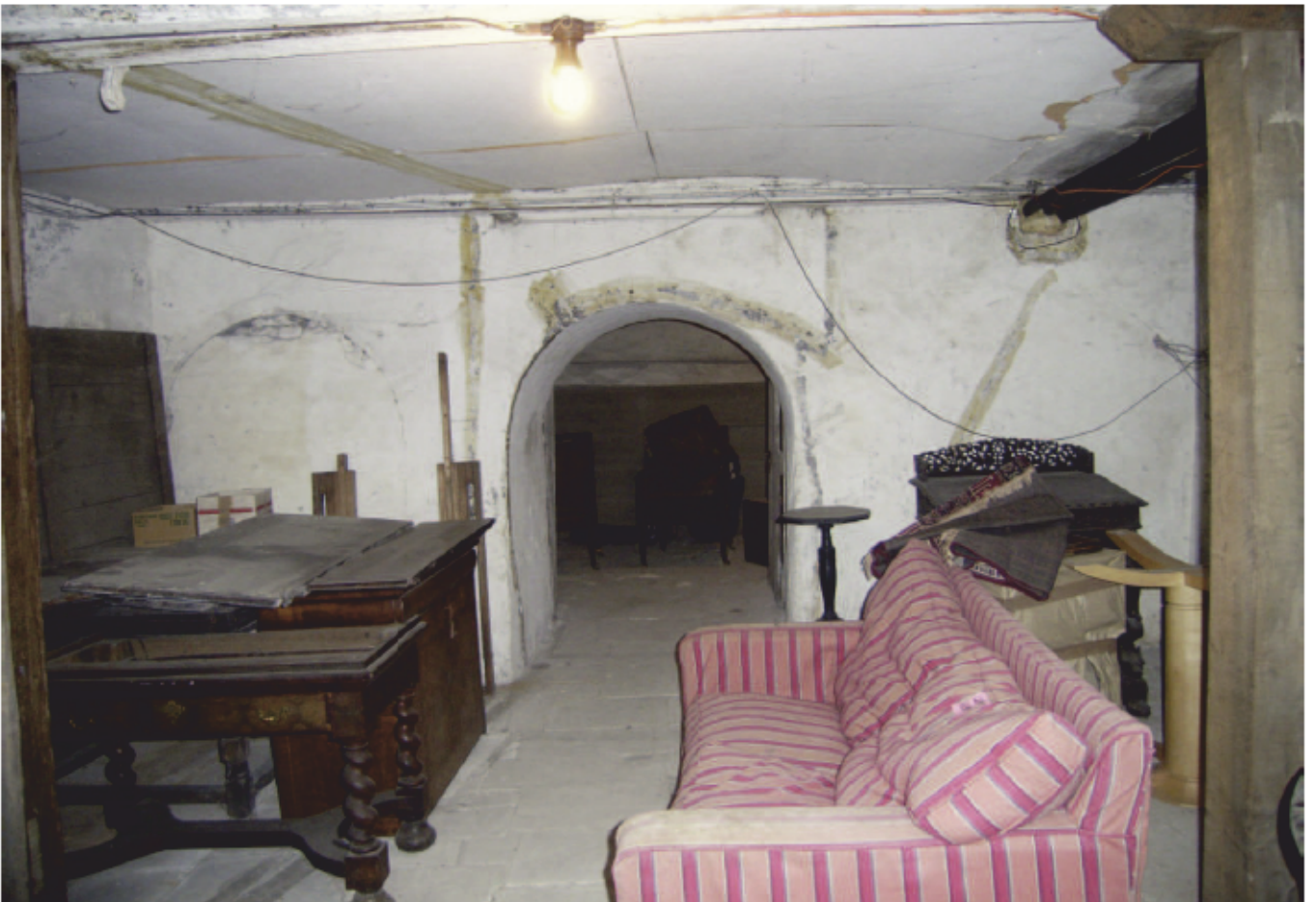
Plate 30: Support arches in wall dividing Areas 3 and 4, facing south
