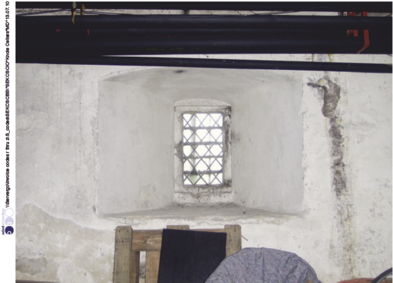
Plate 25: Window in north wall of Area 3
