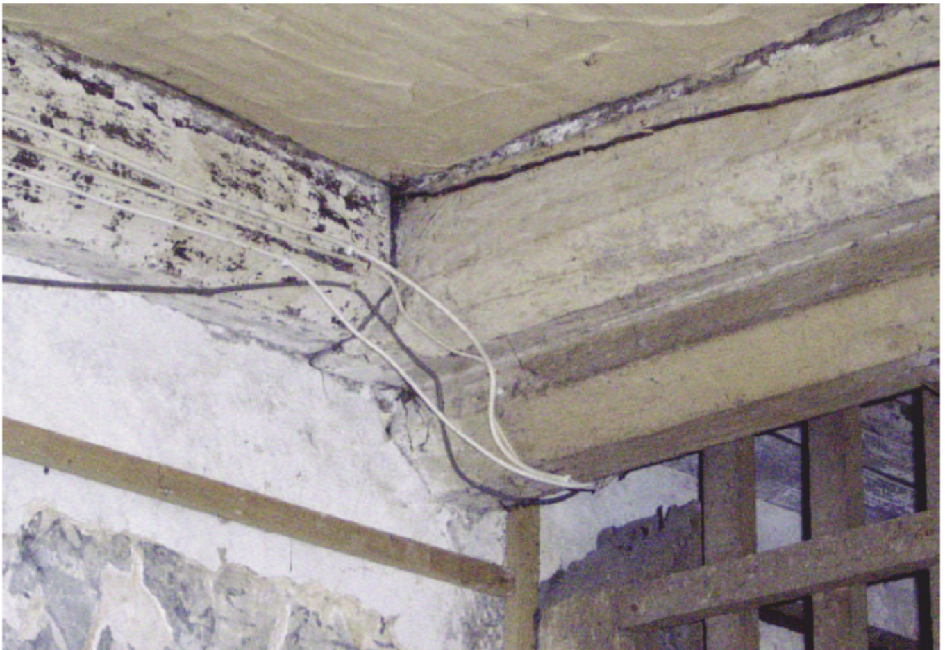
Plate 13: Transverse beam and wall plate in Area 2, facing south west
