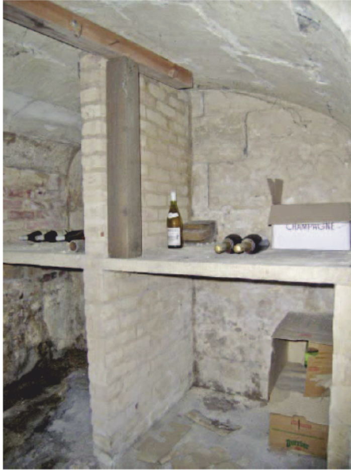
Plate 19: West wall of Wine Cellar, facing south west
