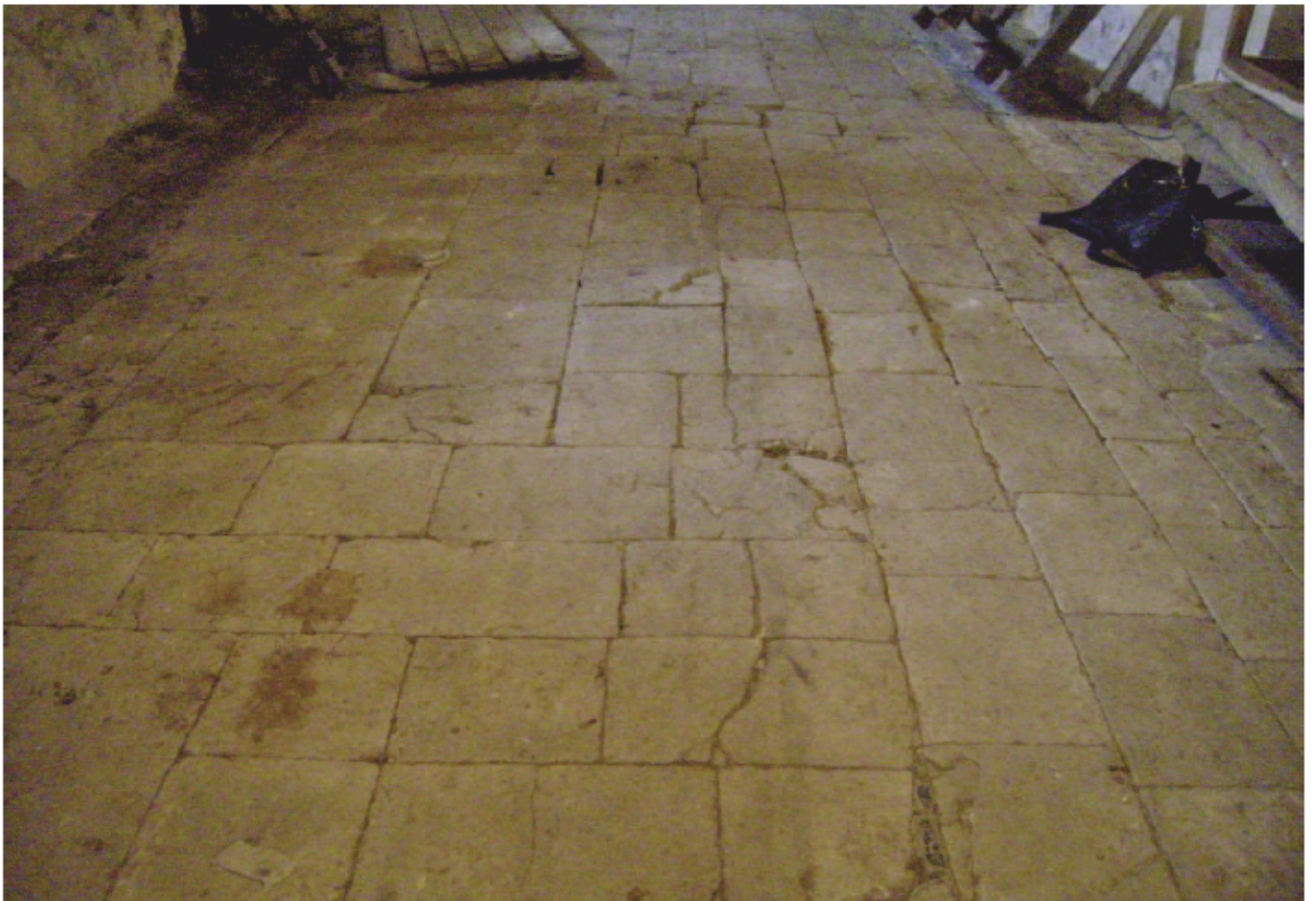
Plate 10: Flagstone floor in Area 2, facing east
