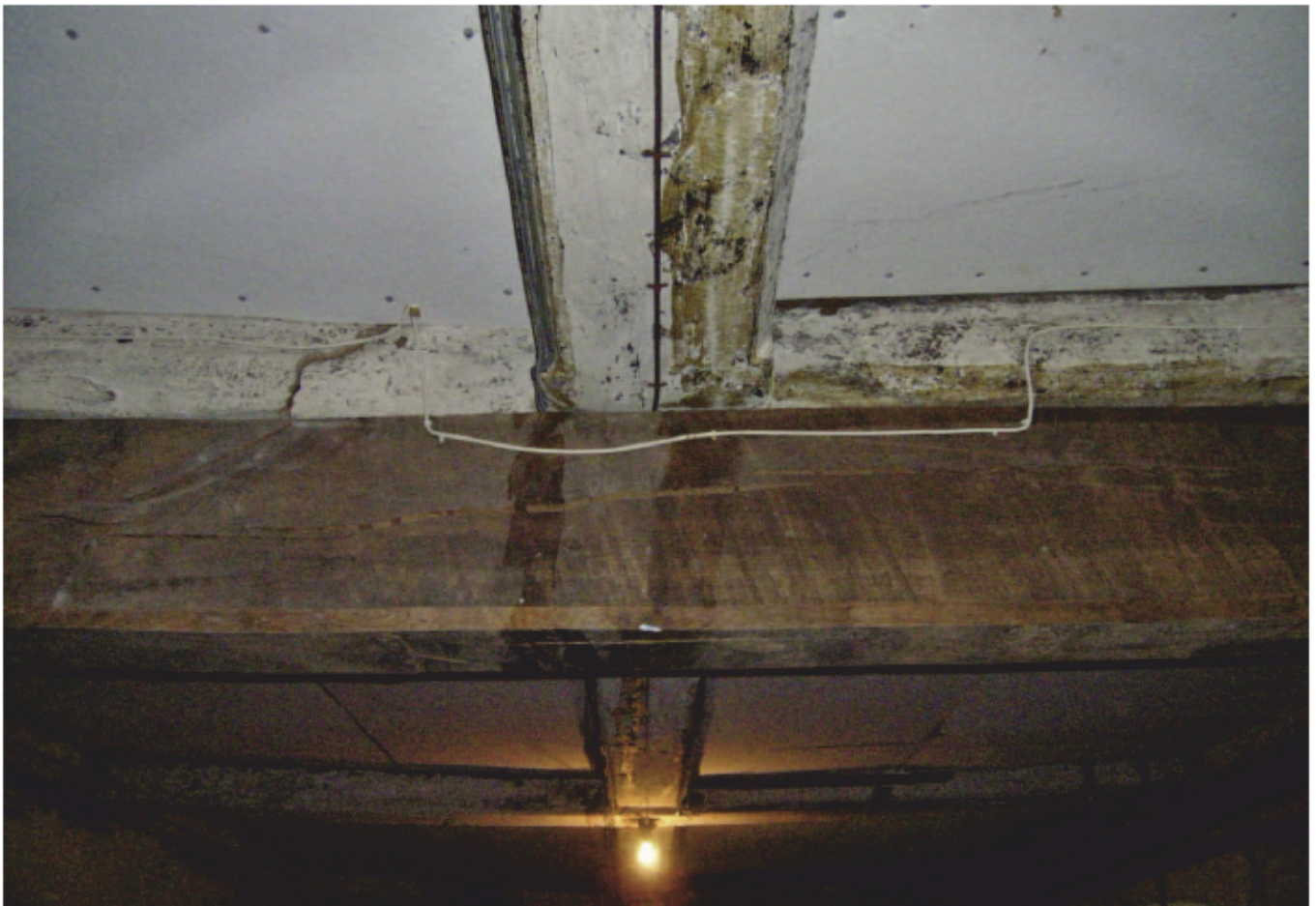
Plate 27: Oak beam support in roof of Area 3, facing west
