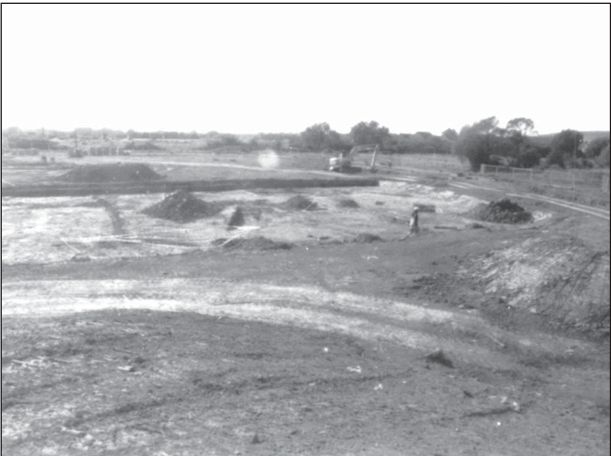
Plate 2: Working shot of the site
