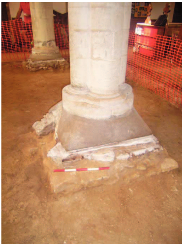
Plate 8: Base of north east cluster column, facing west
