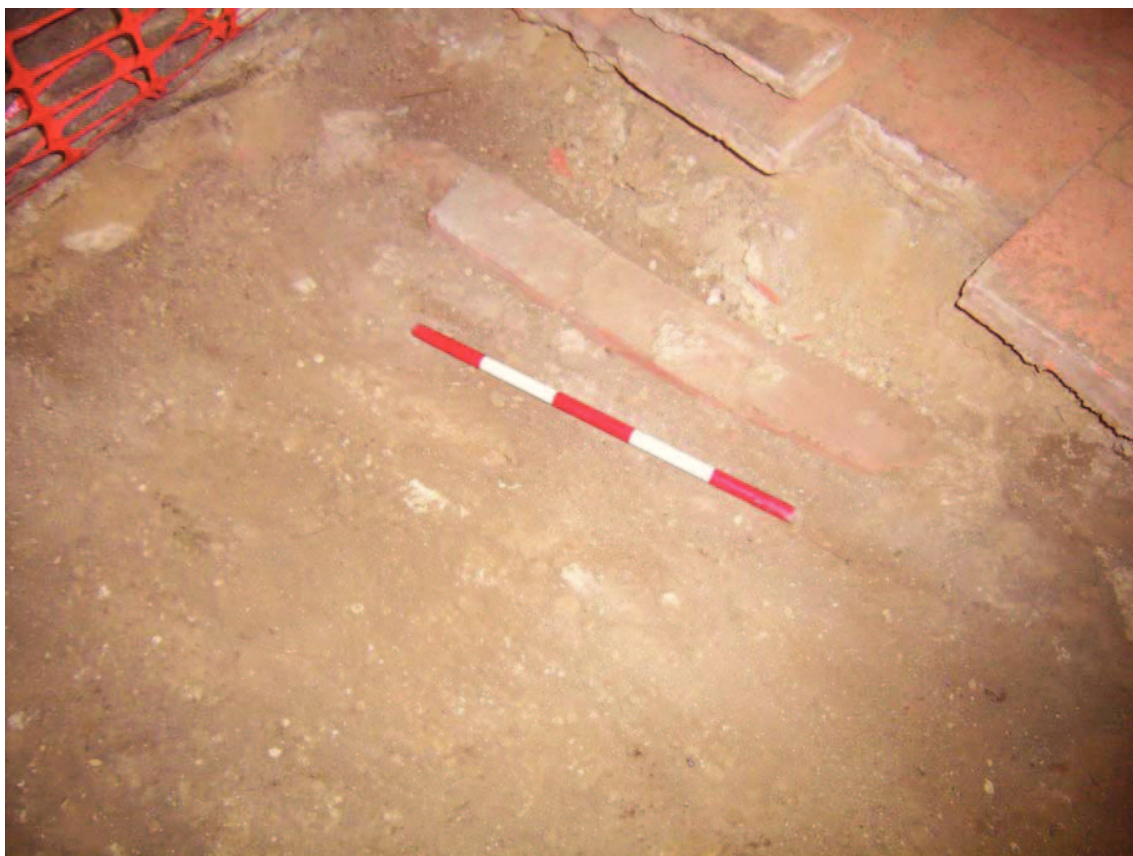
Plate 6: Exposed edge of brick vault in south east corner of nave, facing south east
