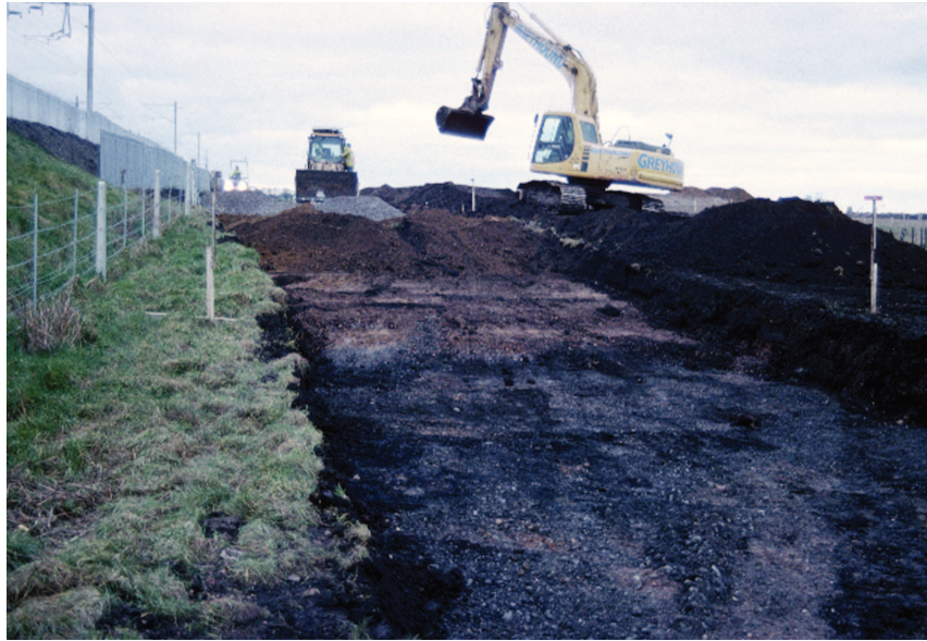
Plate 1: Topsoil stripping, haul road 5
