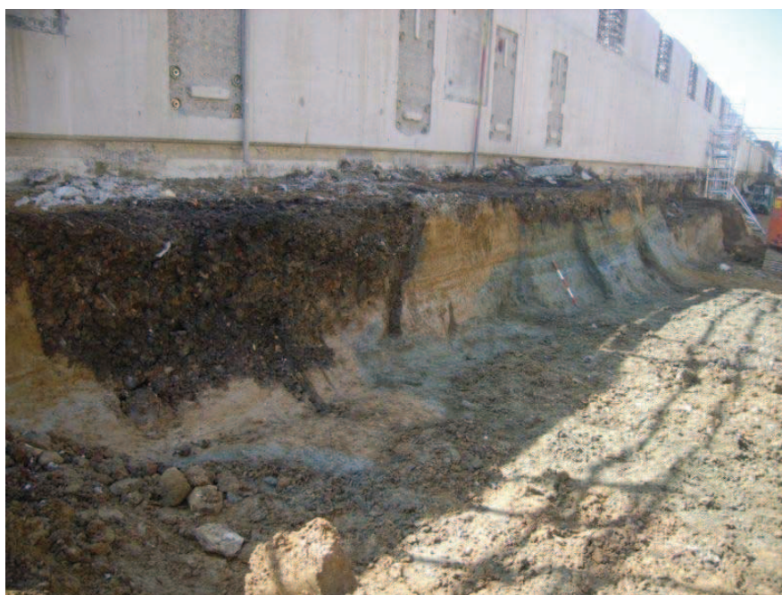
Plate 7: Blue-grey clay of the former river channel, and a 19th-century railway related feature in the foreground, looking south-west
