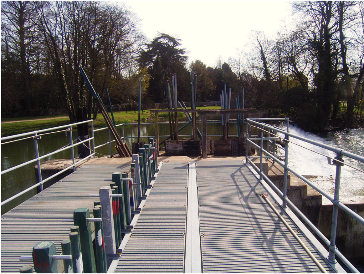
Plate 13: Mapledurham Weir, walkway facing east
