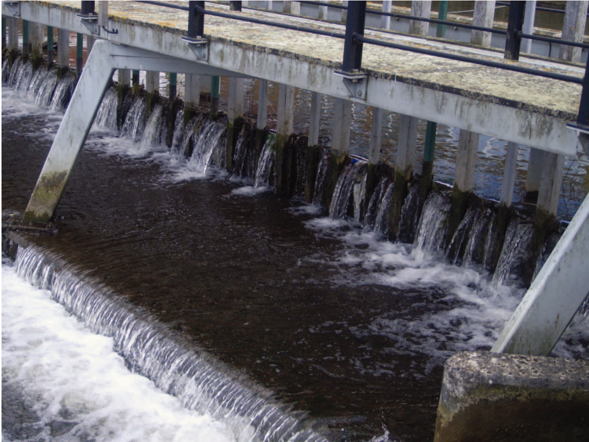
Plate 16: Blakes Weir, facing south east
