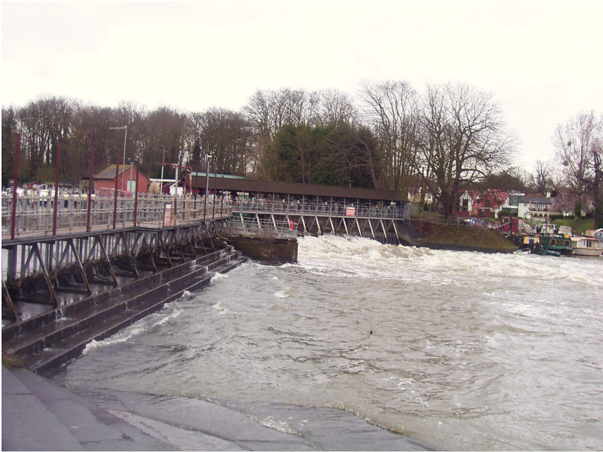
Plate 19: Molesey Weir, facing north west
