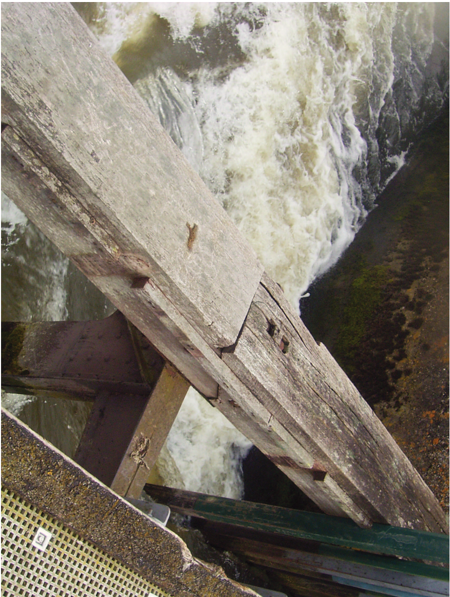
Plate 3: Radcot Weir, scarfed beam for rymer
