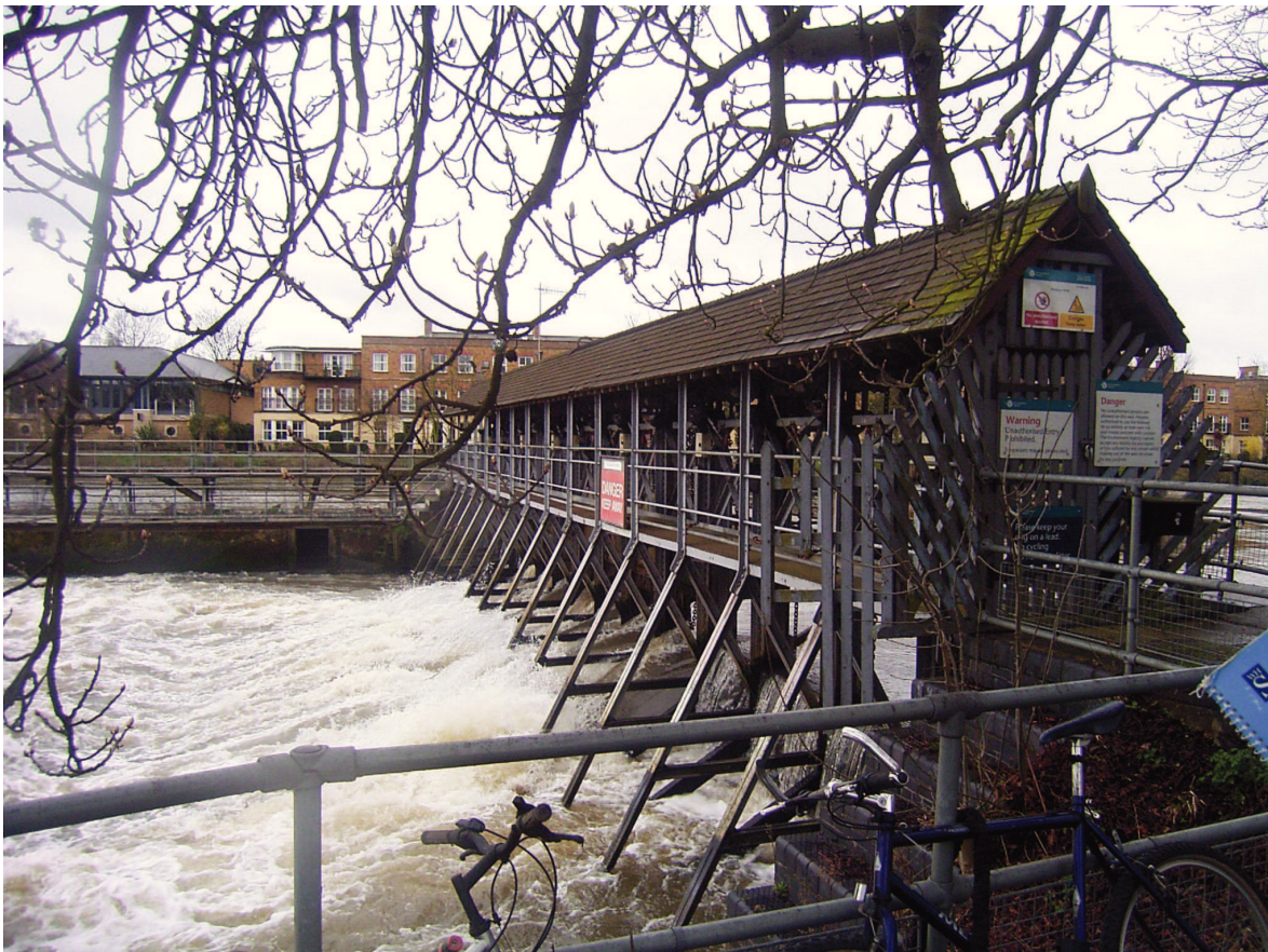
Plate 20: Molesey Weir, radial gate weir facing south
