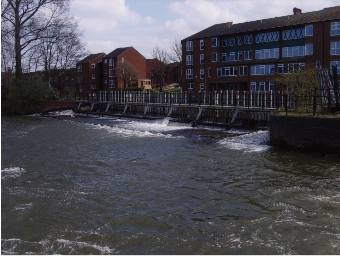
Plate 15: Blakes Weir, facing south east
