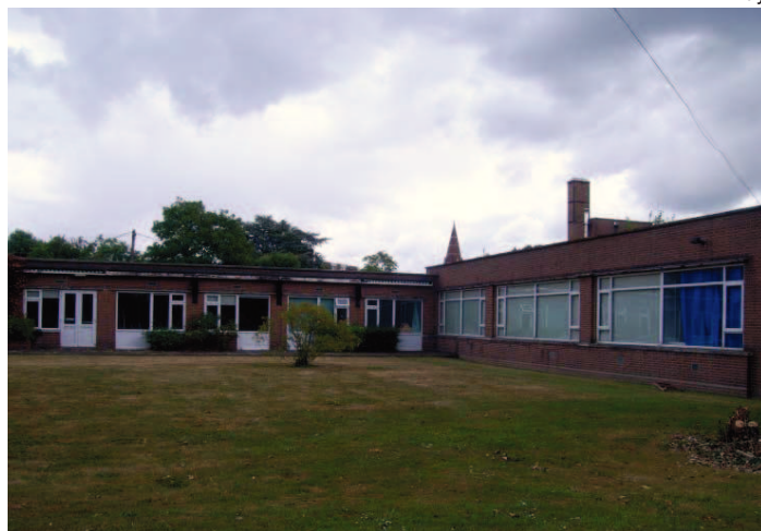
Plate 4: South west wing of the hospital, viewed from the west grounds
