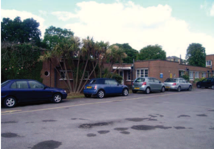
Plate 25: North east elevation of south west wing, facing west
