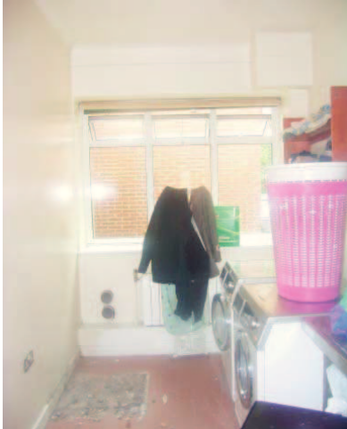
Plate 91: Ground floor utility room, facing north west
