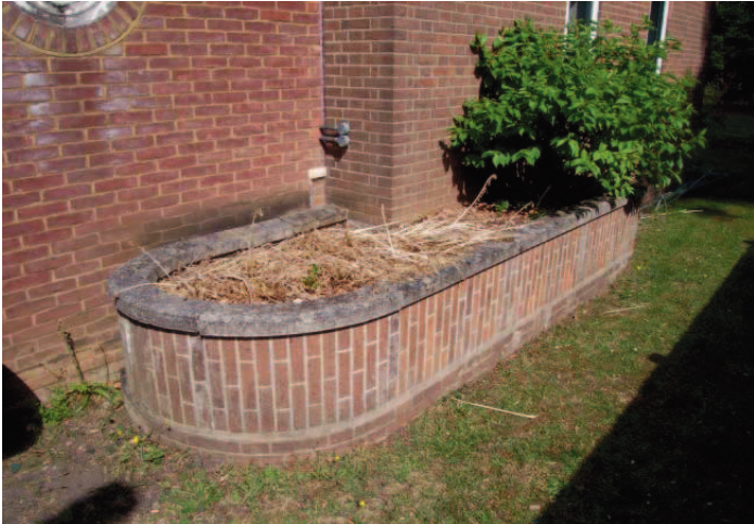
Plate 9: Rounded brick plant box on exterior of south west wing
