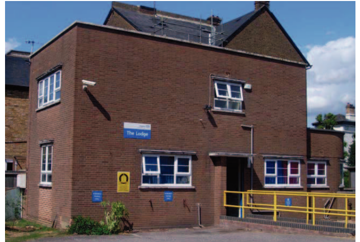
Plate 70: South elevation of the Lodge, facing north
