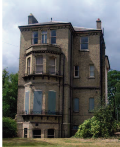
Plate 112: No. 1 Oak Hill, facing west
