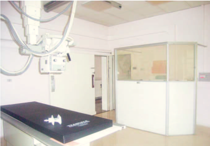
Plate 61: X-ray room, facing west
