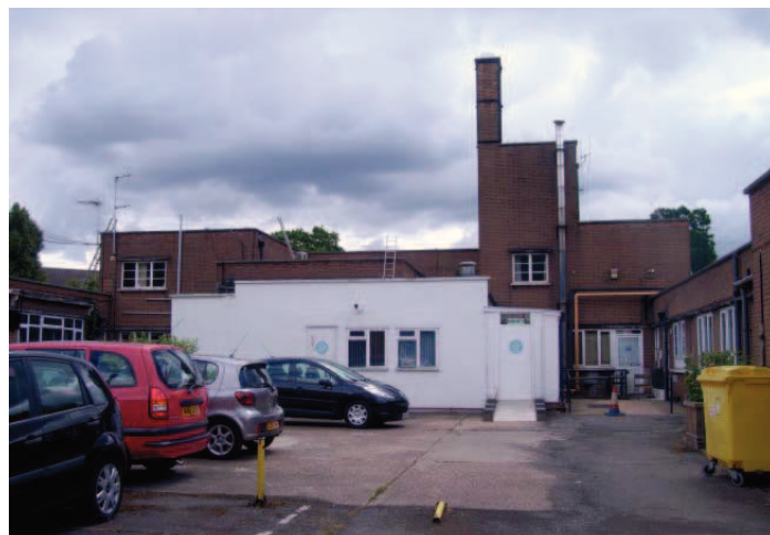
Plate 18: North west/rear of main hospital
