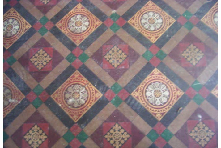
Plate 114: Original mosaic floor in the entrance hall of No. 1 Oak Hill
