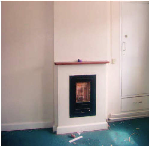
Plate 41: Original fireplace on first floor of main axis
