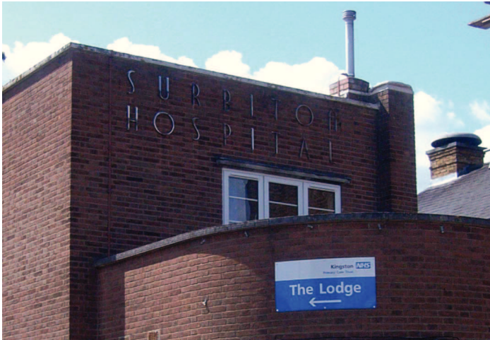
Plate 69: Detail of stainless steel lettering on facade of the Lodge
