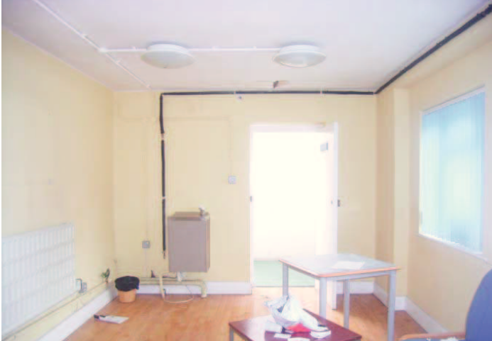
Plate 37: Small day room in extension of kitchen block, facing south west
