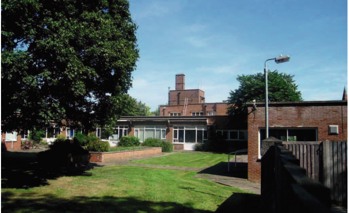
Plate 5: South west wing of the hospital, viewed from the south west grounds
