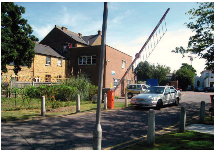
Plate 71: The Lodge, viewed from hospital grounds, facing north east
