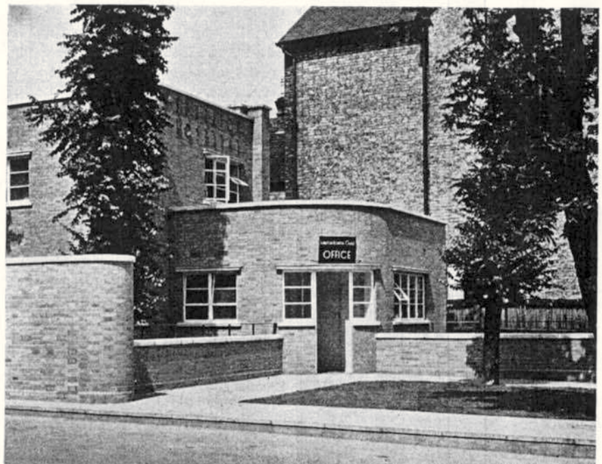
The entrance lodge, which, like the main building, is in light-toned bricks.
