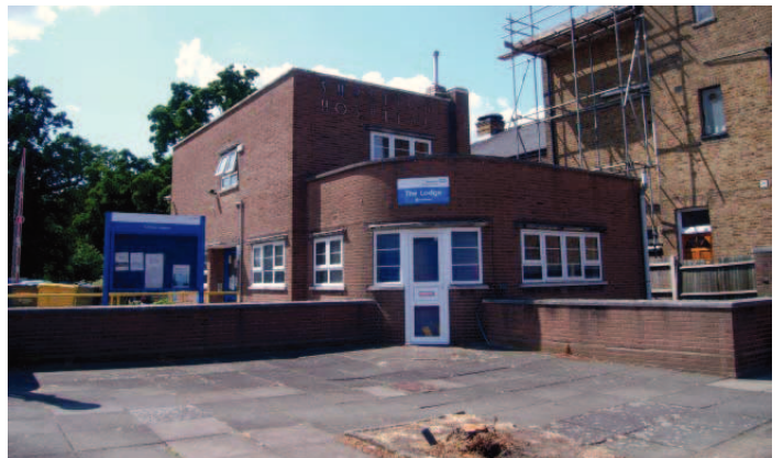
Plate 68: East facade of the Lodge, facing north west
