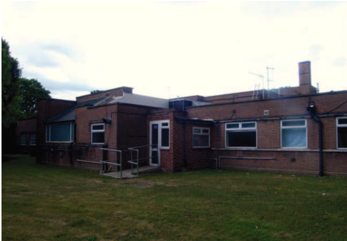
Plate 27: North east elevation of north east wing, facing south
