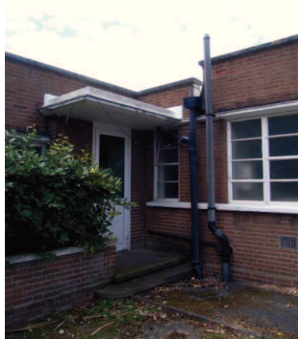
Plate 10: Cantilevered concrete porch on north east side of south west wing
