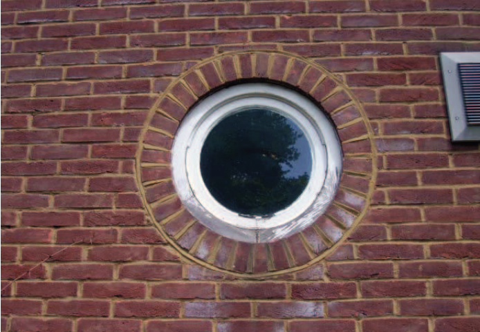
Plate 13: Primary porthole window on south west wing
