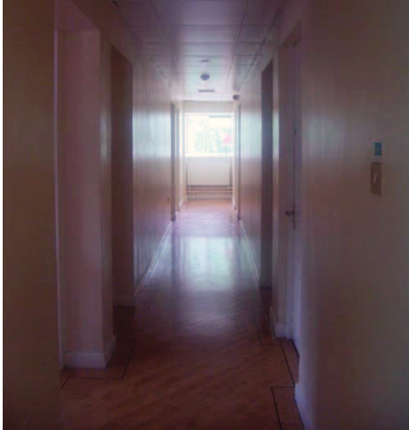
Plate 101: First floor corridor, facing north east
