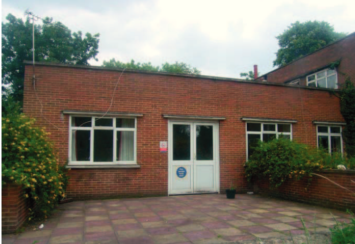
Plate 89: South west elevation of extensions
