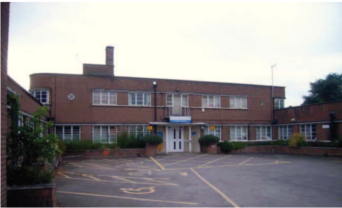
Plate 15: South east front/facade of main hospital
