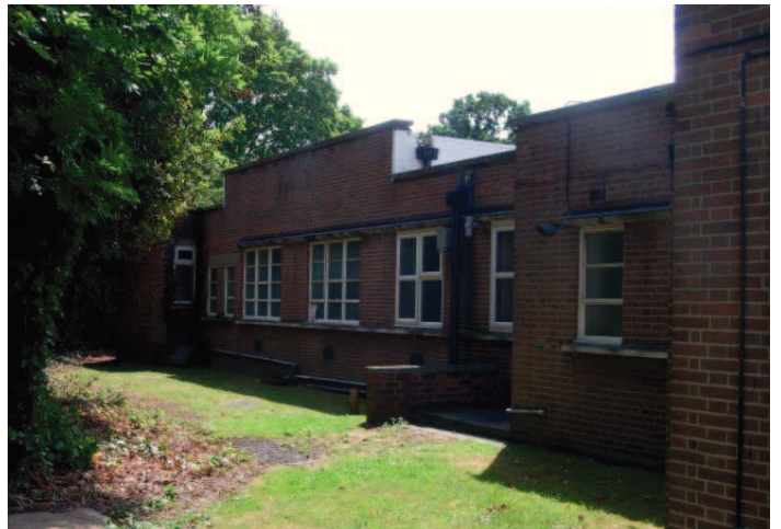
Plate 28: North east elevation of north east wing, facing south
