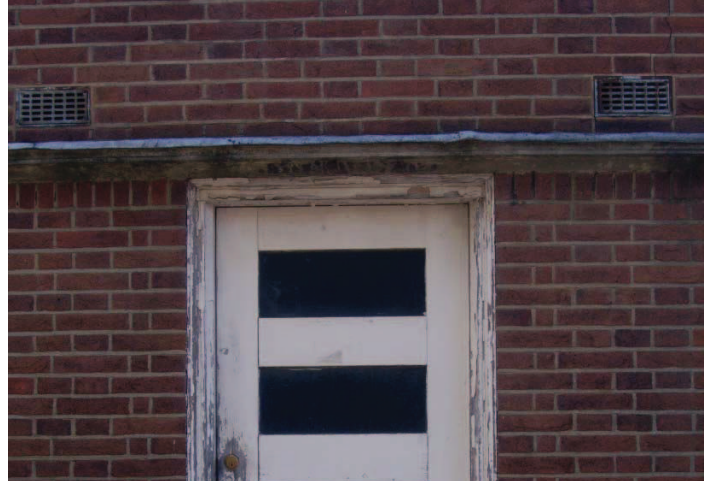
Plate 14: Primary wooden panelled door with moulded wooden architrave on Mortuary unit
