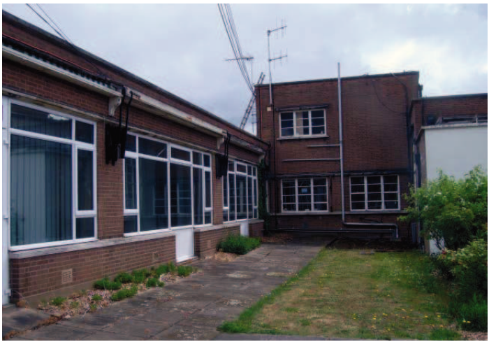
Plate 31: South west elevation of north east wing, facing east
