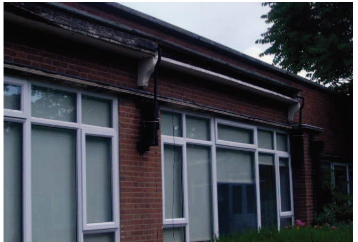
Plate 24: Awning fixture on south west elevation of south west wing
