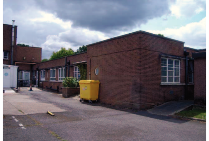
Plate 26: North east elevation of south west wing, facing south
