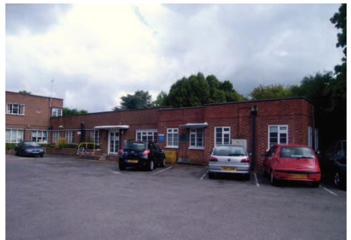
Plate 32: South west elevation of north east wing showing 1948 extension
