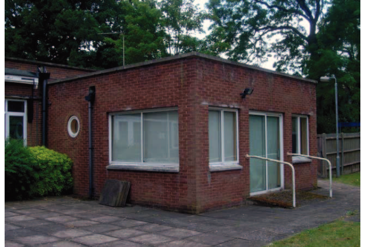
Plate 22: Later extension on linear ward of south west wing, facing south
