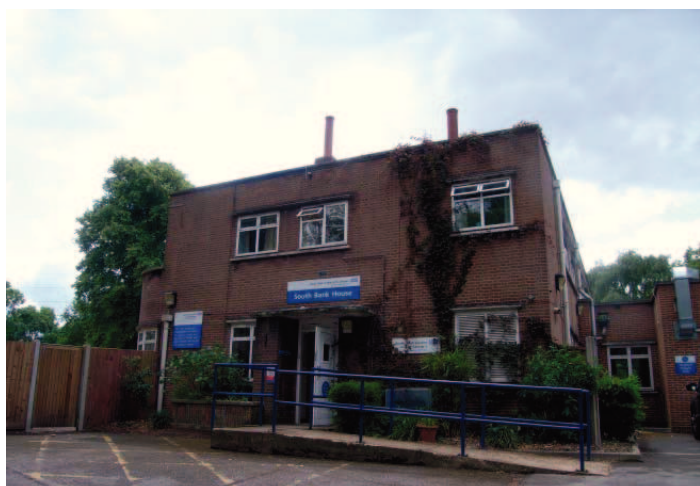
Plate 83: North east front of South Bank House
