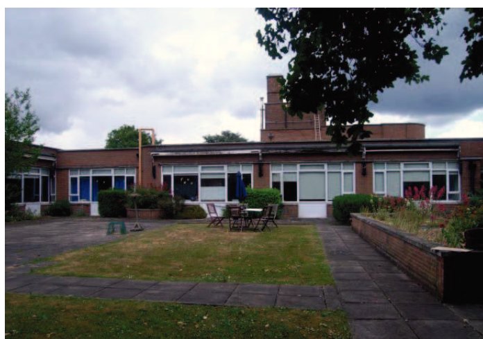
Plate 20: South west face of south west wing, facing north east
