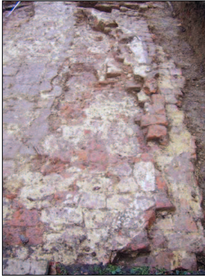
Plate 15: Trench 3, view of footing of north bay window built out from wall 320, showing mortar traces revealing position of window structure
