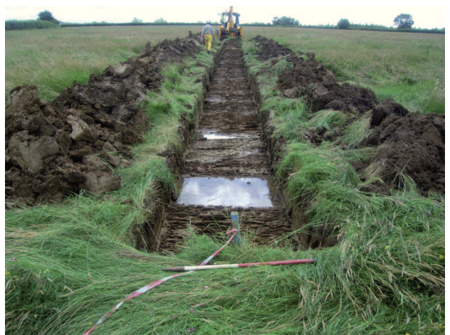
South-West facing photograph of Trench 6
