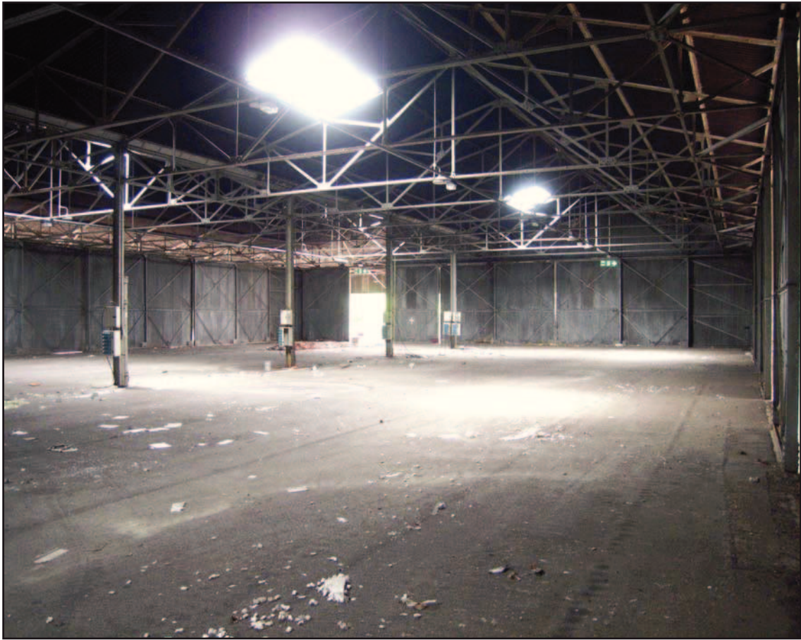
Plate 9: Internal view at south end of south shed
