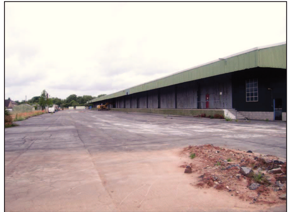
Plate 4: General view of west side of north shed
