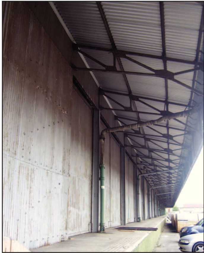
Plate 6: Covered platform on west side of north shed
