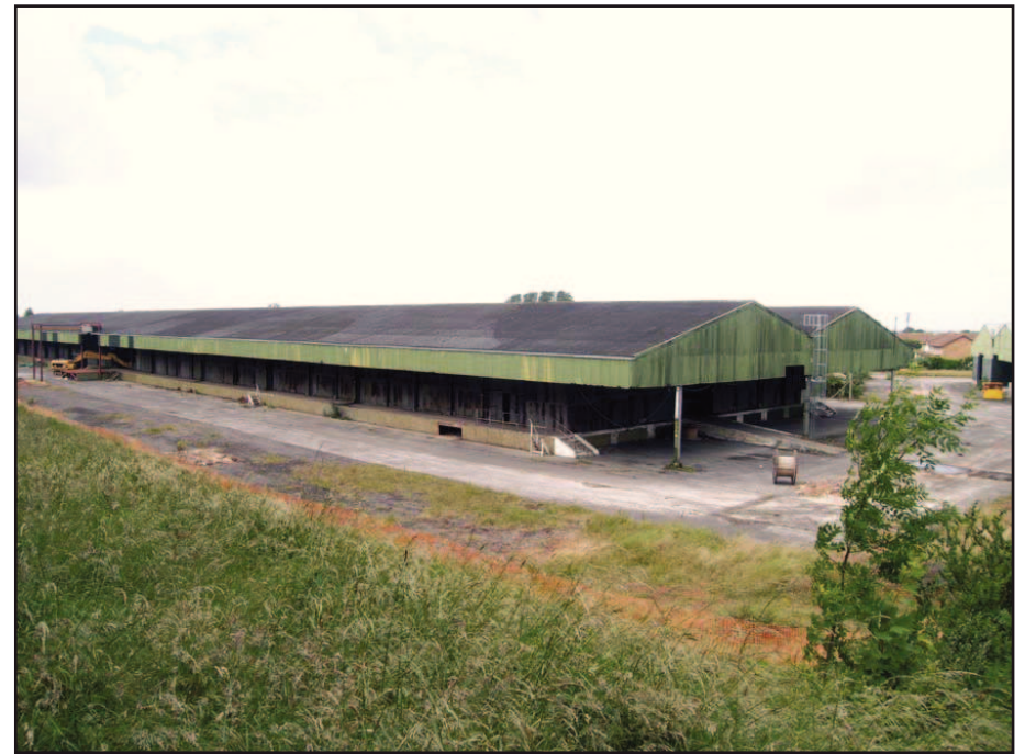
Plate 2: General view of south shed
