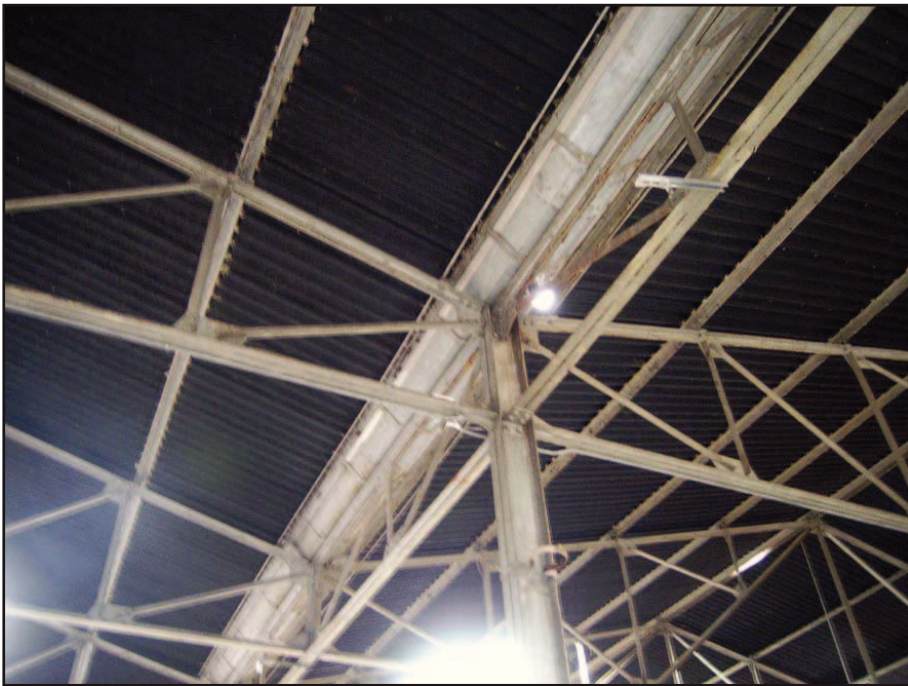
Plate 19: Truss detail at valley
