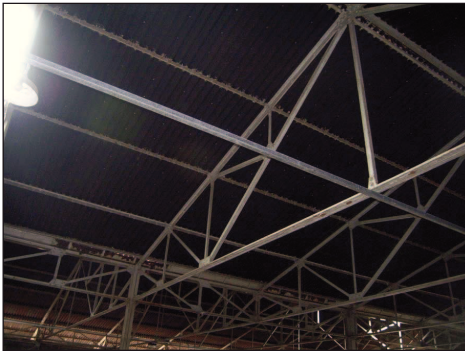
Plate 11: Roof trusses in south shed
