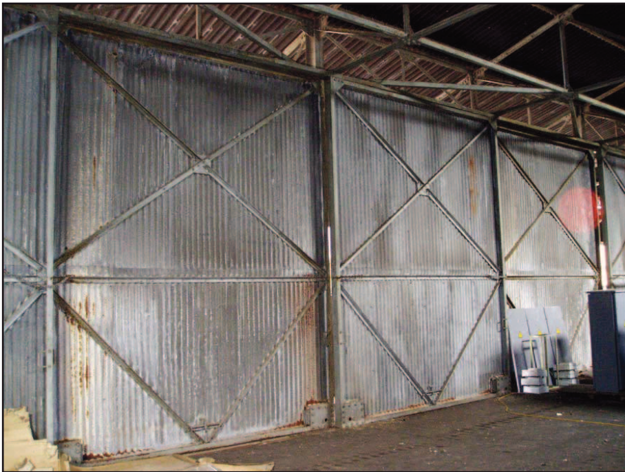
Plate 7: Wall frame in south shed
