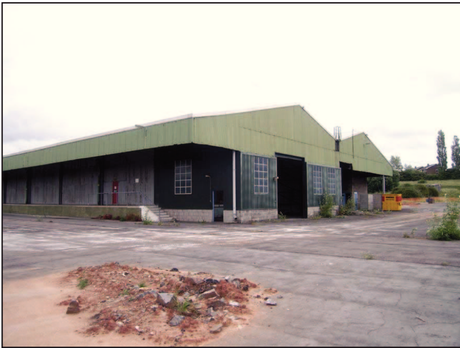
Plate 5: South end of north shed
