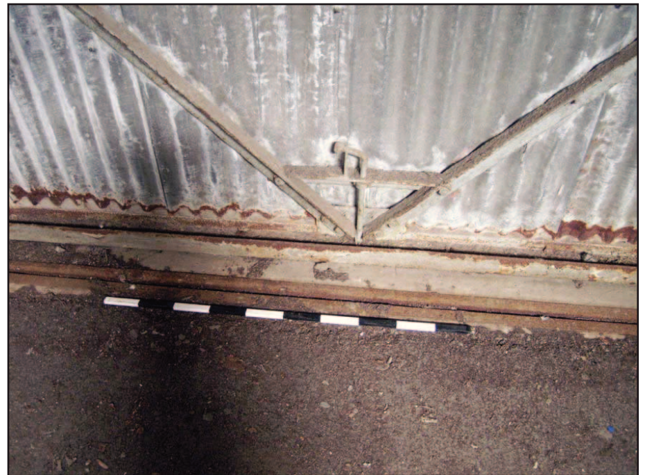
Plate 14: Detail of wall in south shed
