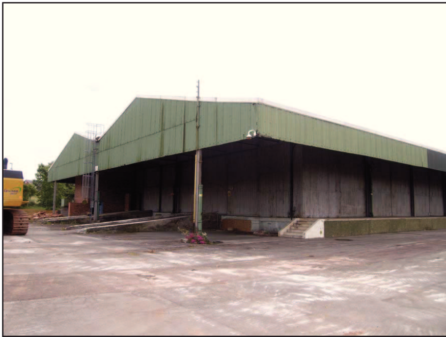
Plate 1: North end of north shed
