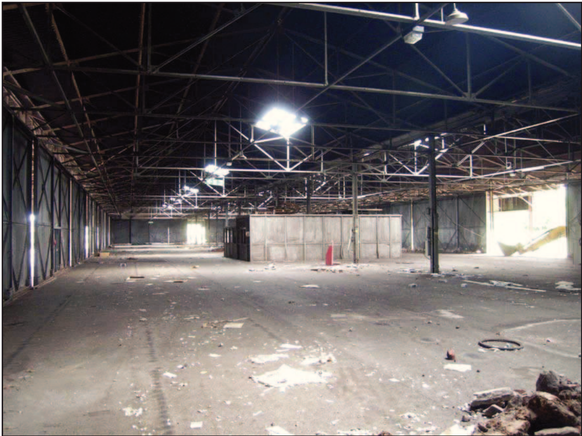
Plate 10: South shed interior looking north
