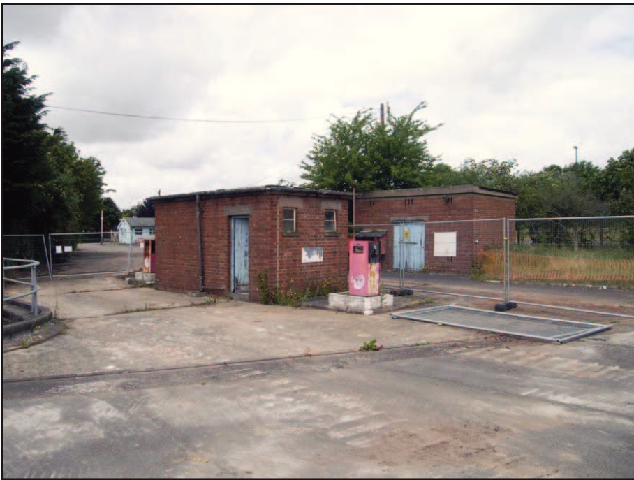
Plate 23: Electrical substation and lodge at entrance
