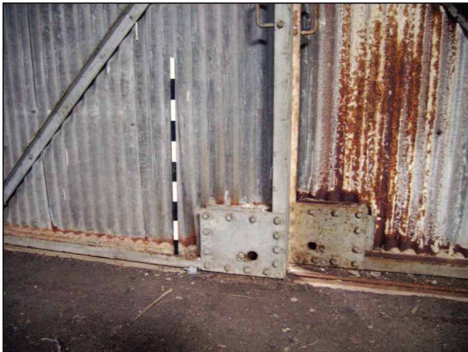
Plate 13: Detail of wall in south shed
