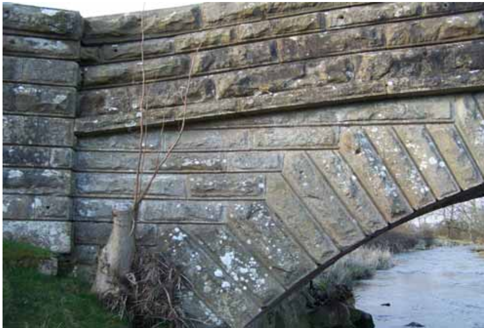
Plate 15: Low Bridge from the south, showing the mid-nineteenth century masonry on this side of the arch
