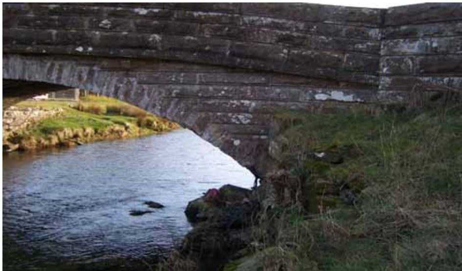
Plate 14: Low Bridge from the north, showing possible seventeenth-century masonry in this side of the arch
