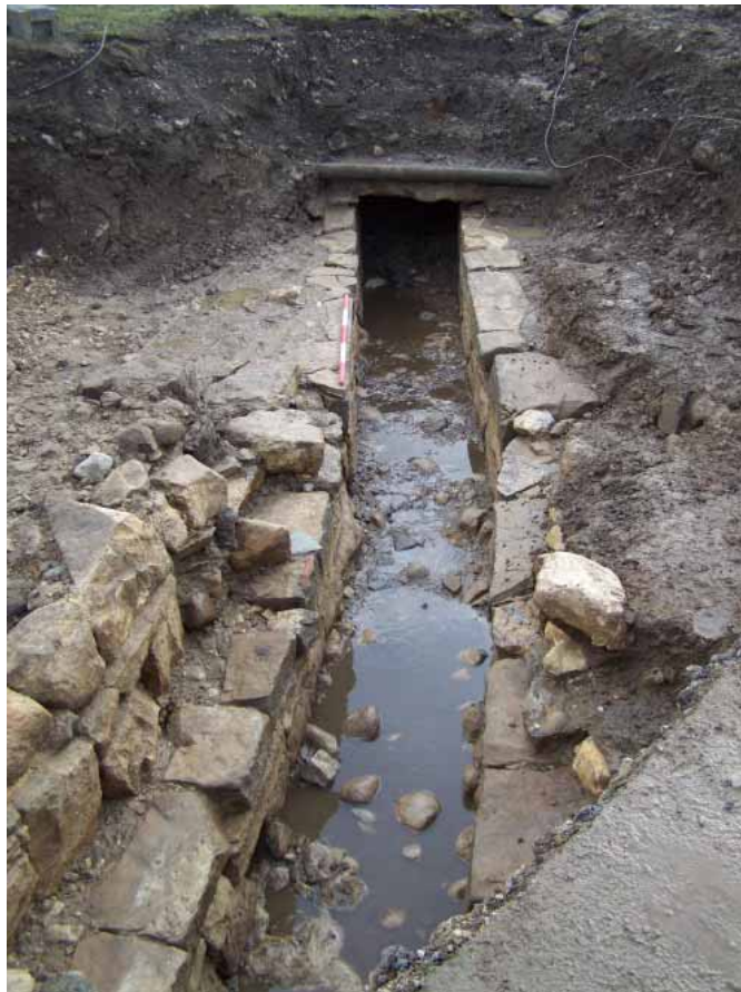
Plate 6: The tail-race for the former corn and saw mill (SG 168), looking south-east, with capping stones removed, showing stone lining 170/171
