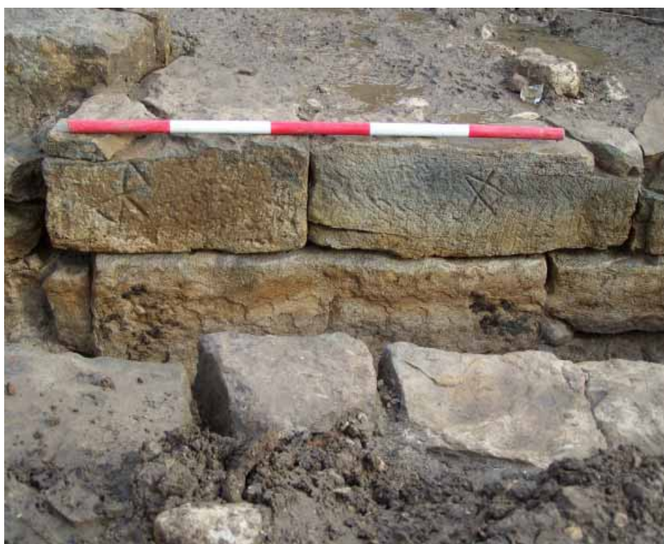
Plate 8: Masons' marks on stonework ( 170 ) in the eastern side of the tail-race channel (SG 168 )
