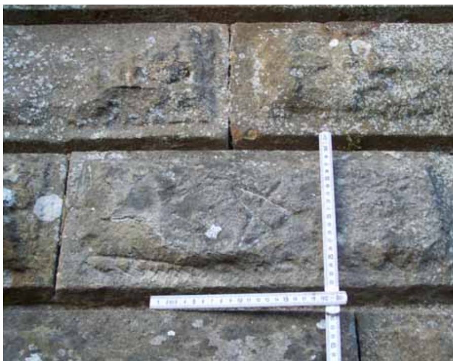
Plate 19: Low Bridge: another mason's mark on mid-nineteenth-century masonry on the south side of the bridge
