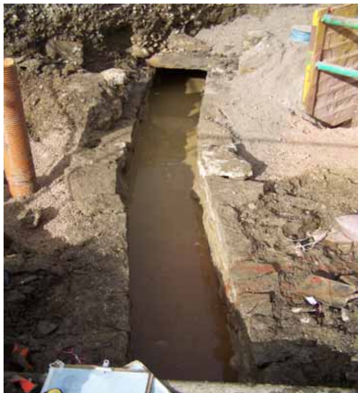
Plate 12: The stone lining (170/171) of tail-race channel SG 168 rebuilt following insertion of pipe
