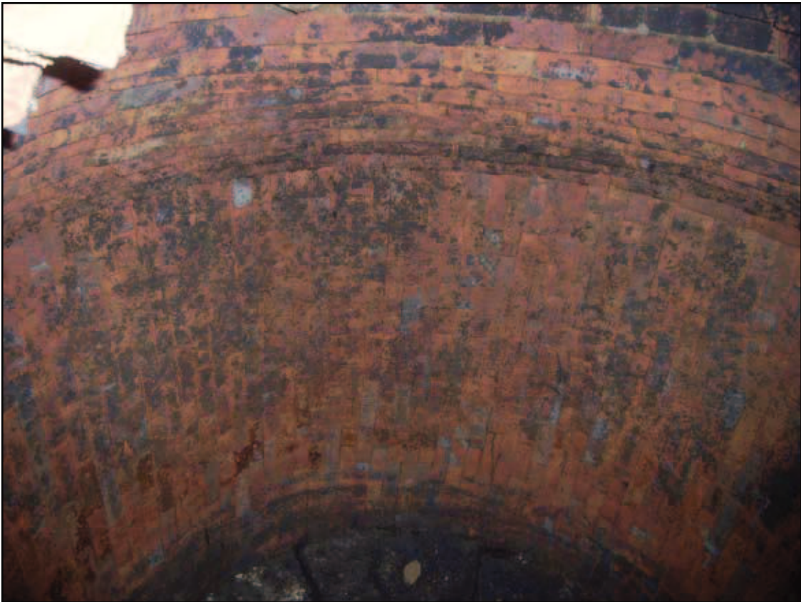
Plate 2: Well 24 showing interior brick lining
