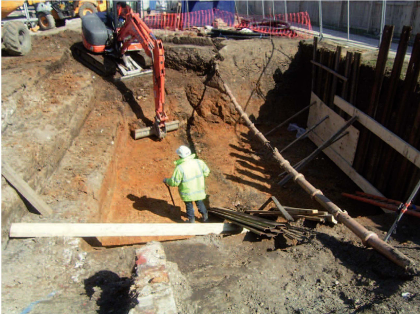
Plate 29: Trench 11, working shot, looking east
