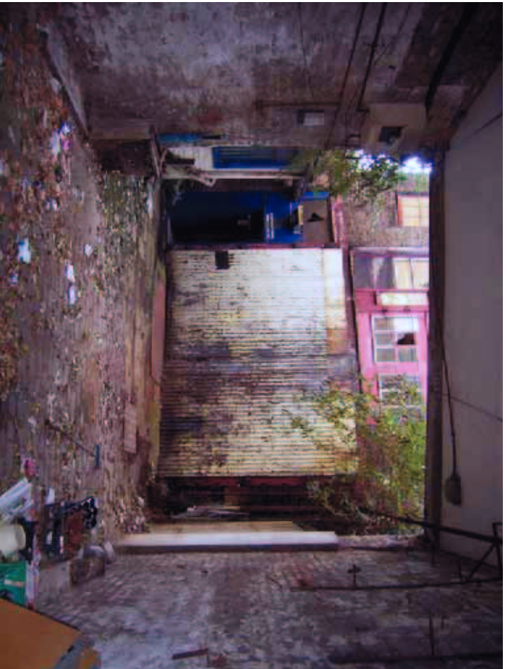
Entrance in north elevation
