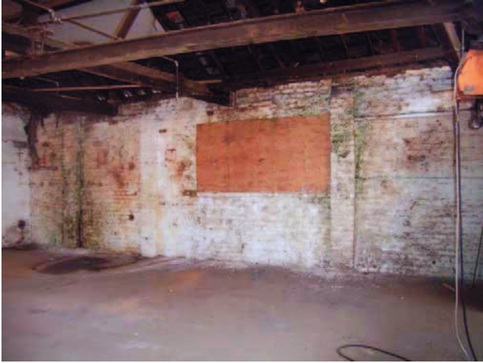
West elevation of north room on first floor
