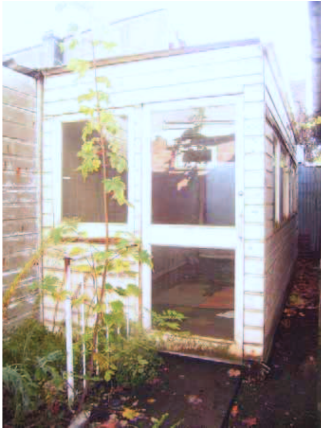
Prefabricated office outside south end of metal works, facing south
