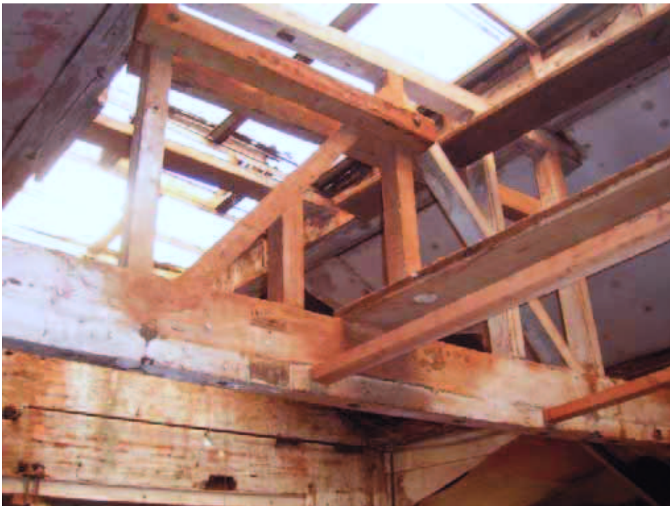
Roof structure of south room on first floor, facing north-east
