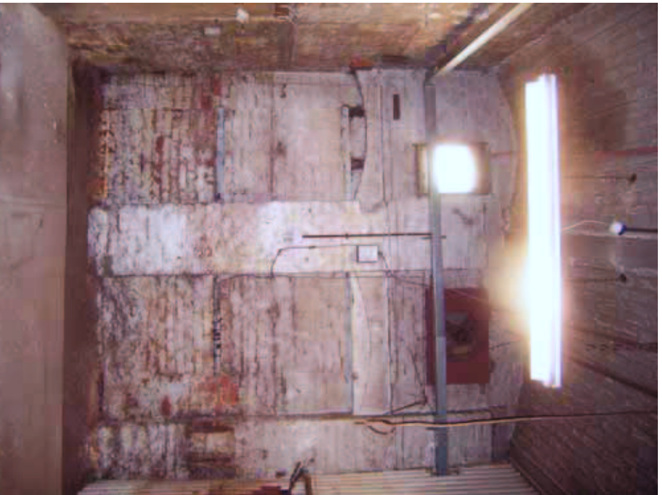
Detail of south interior elevation
