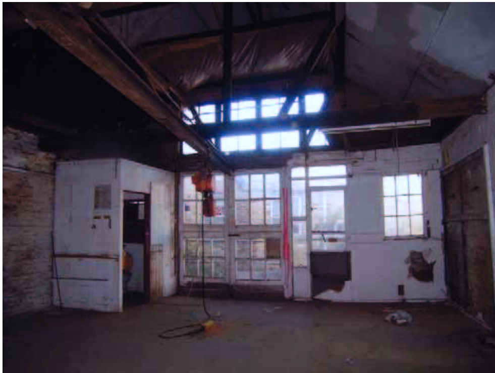
North elevation of north room on first floor
