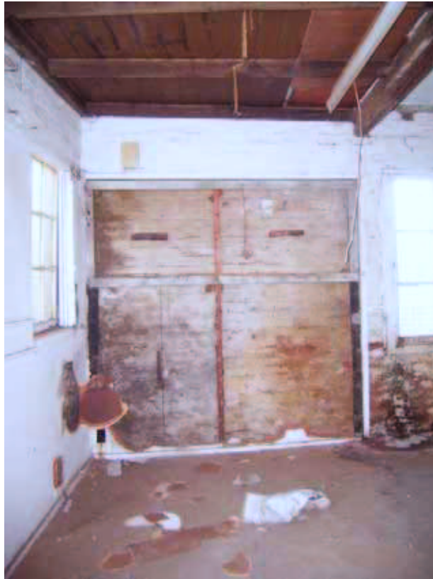
Detail in east elevation of north room on first floor
