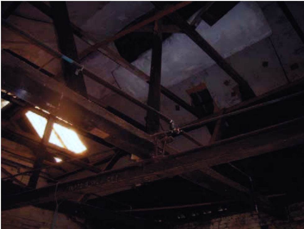
Roof structure in north room on first floor, facing south-west
