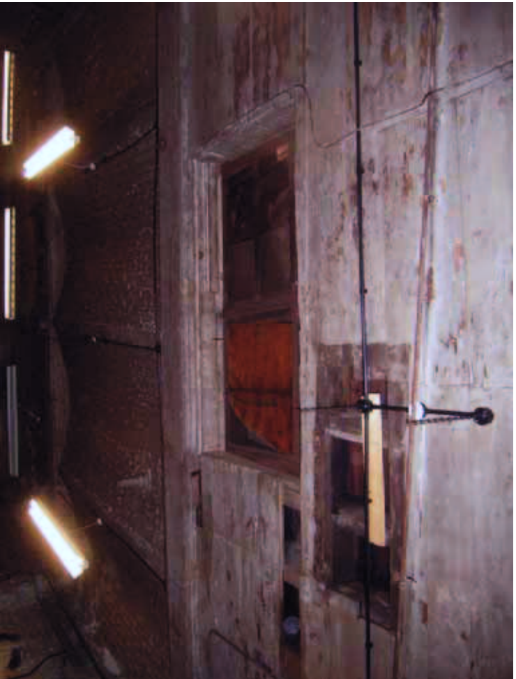
Ceiling detail, facing south
