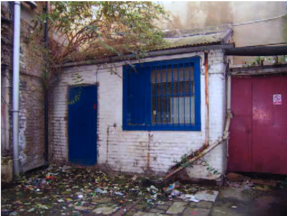
Lean-to outside north end of metal works, facing east
