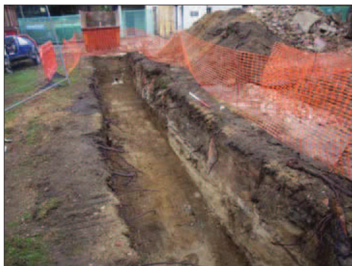
Plate 3: Trench 3 showing modern drains, looking NNE
