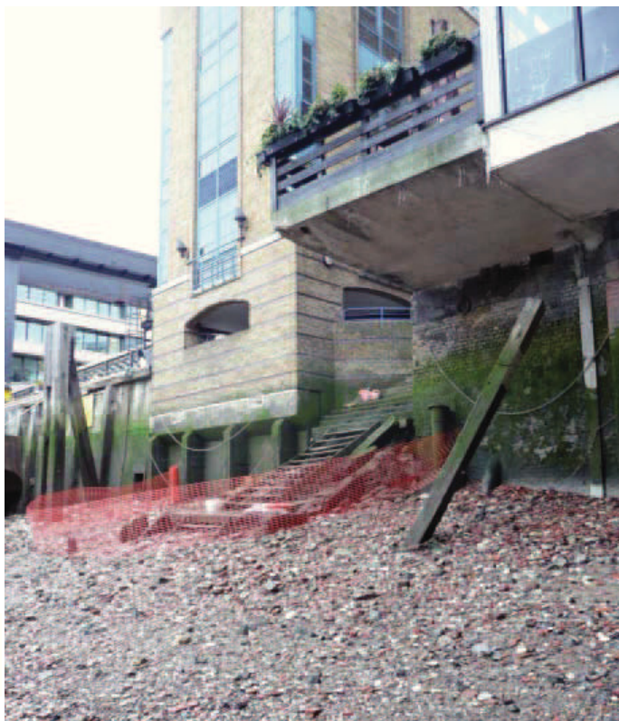
Plate 1: Site viewed from the south-east
