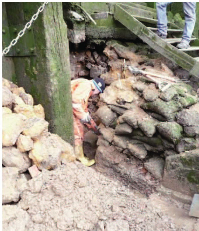
Plate 2: Working in TP01
