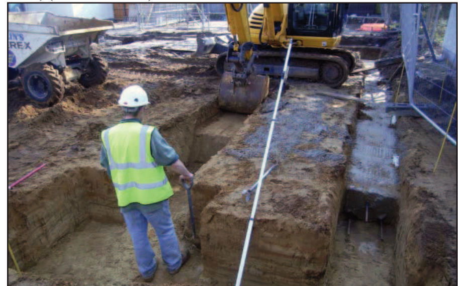
Plate 4 Working shot, excavation of Building A footing trenches (view east)
