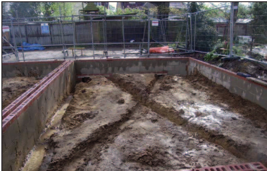
Plate 7 Sewage and water service trenches in Building A (view east)
