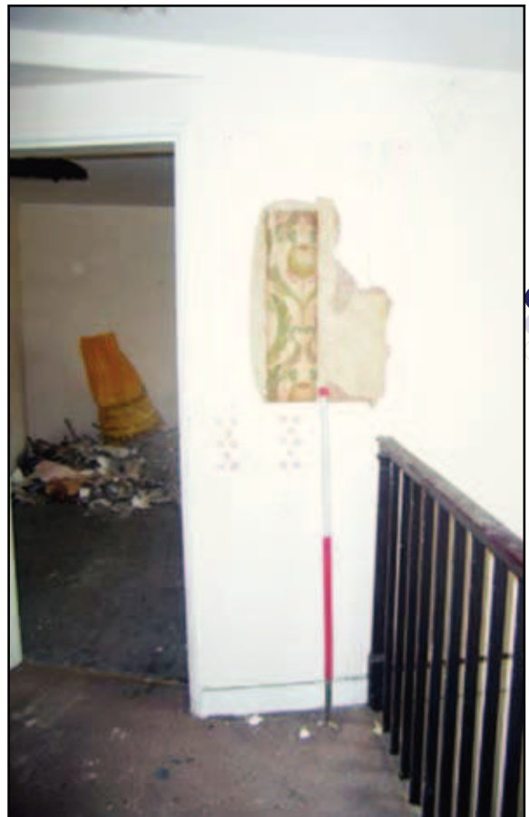
Plate 30: 27 Holywell, second floor detail of wallpaper
