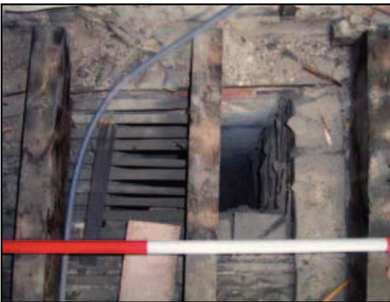
Plate 29: 27 Holywell, first floor void within extension following removal of boards
