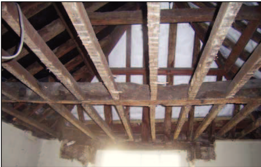
Plate 33: 27 Holywell, exposed roof timber frame
