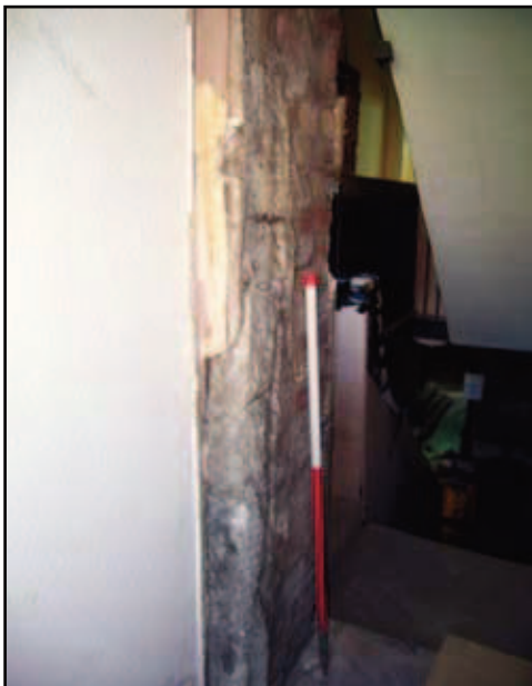
Plate 23: 27 Holywell, detail of first floor extension door reveal
