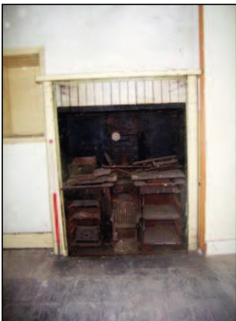
Plate 25: 27 Holywell, ground floor early 20th century range oven
