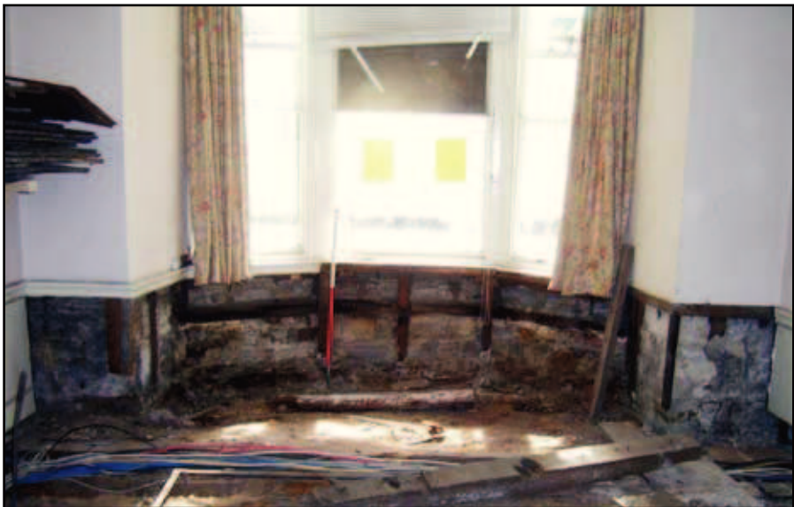
Plate 17: 27 Holywell, ground floor bay window
