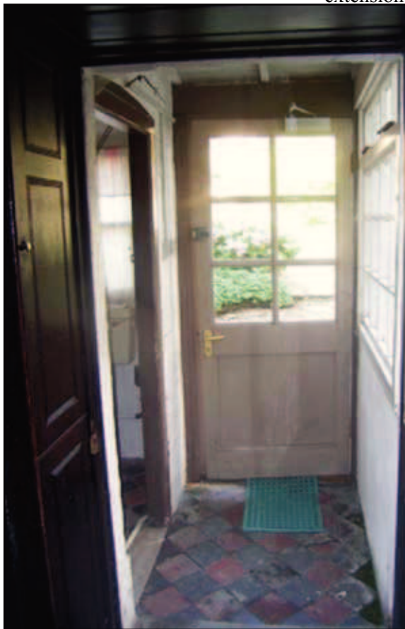
Plate 5: 27 Holywell, ground floor rear entrance
