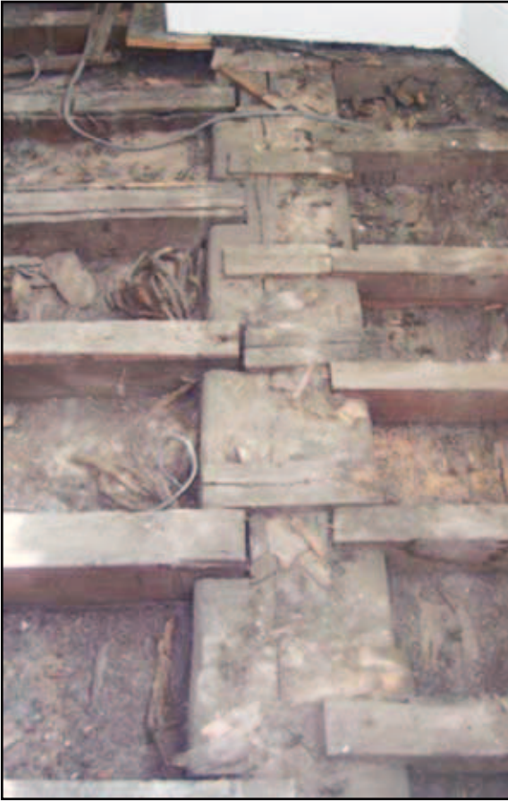
Plate 27: 7 Holywell, second floor reception room following removal of boards
