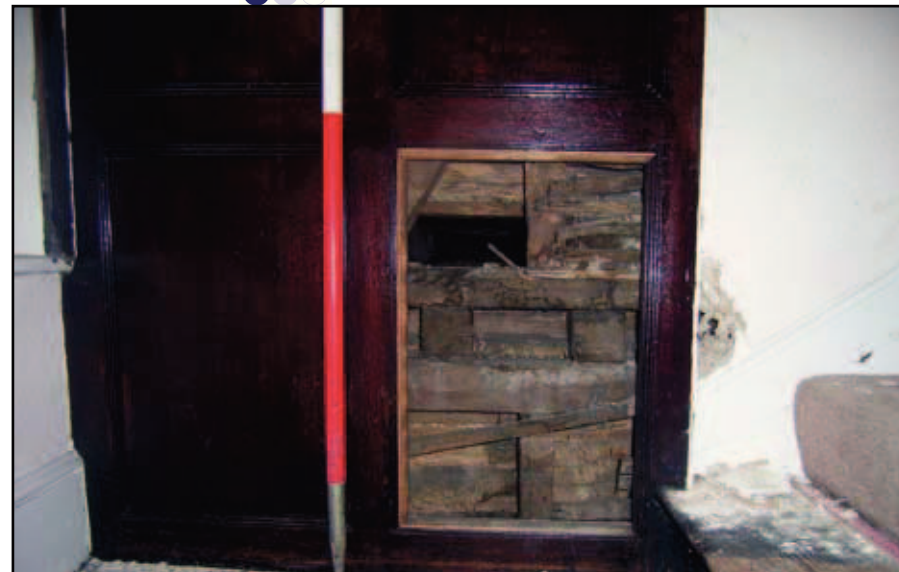
Plate 24: 27 Holywell, detail of floor construction of first floor
