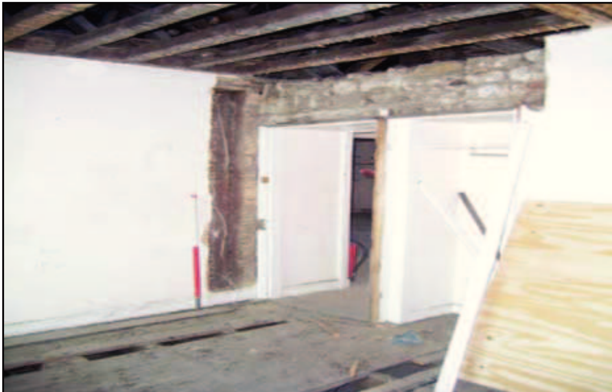
Plate 31: 27 Holywell, second floor detail of partition walling
