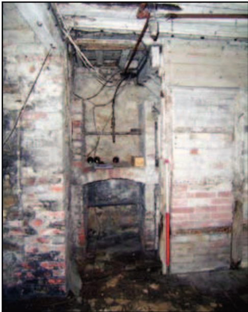
Plate 15: 27 Holywell, cellar view of storage shelves
