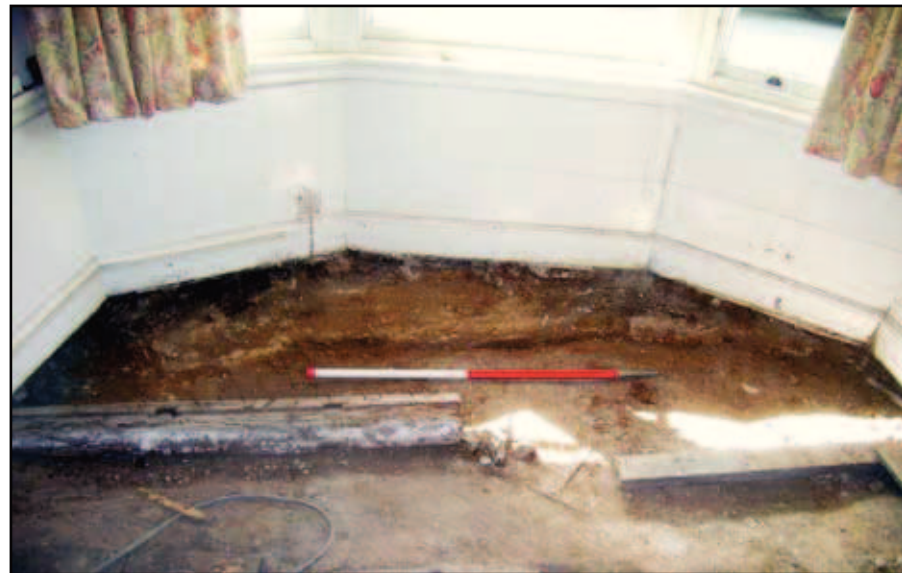
Plate 18: 27 Holywell, ground floor detail of early footing
