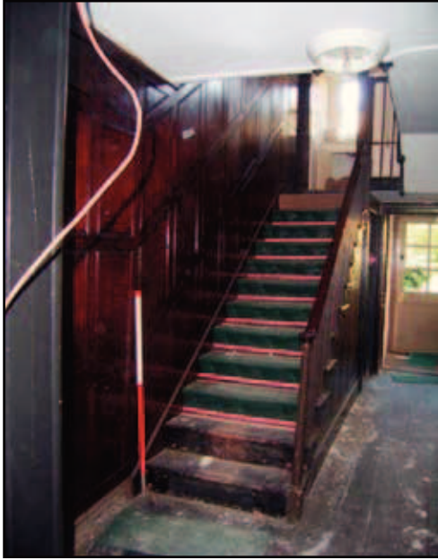
Plate 7: 27 Holywell, ground floor stairs
