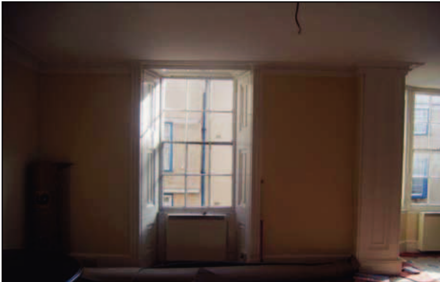
Plate 9: 27 Holywell, first floor reception room windows
