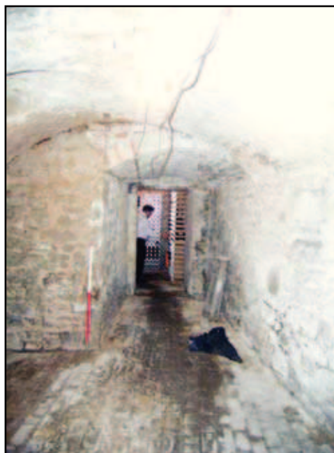
Plate 14: 27 Holywell, cellar general view
