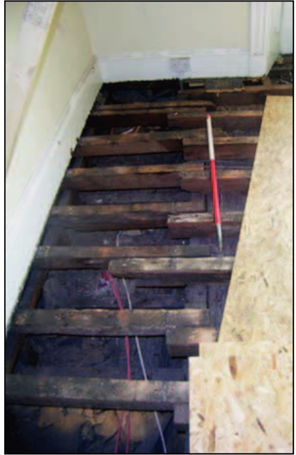
Plate 28: 27 Holywell, second floor reception room extension to floor joists
