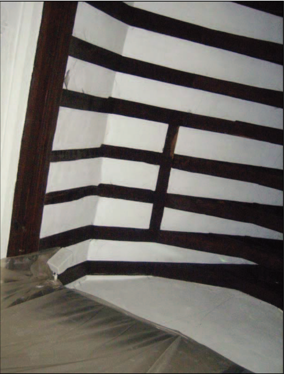
Plate 28: Trimmer visible from beneath in chapel
