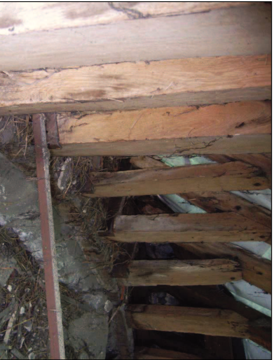
Plate 24: Detail of studs in semi circular east part of roof
