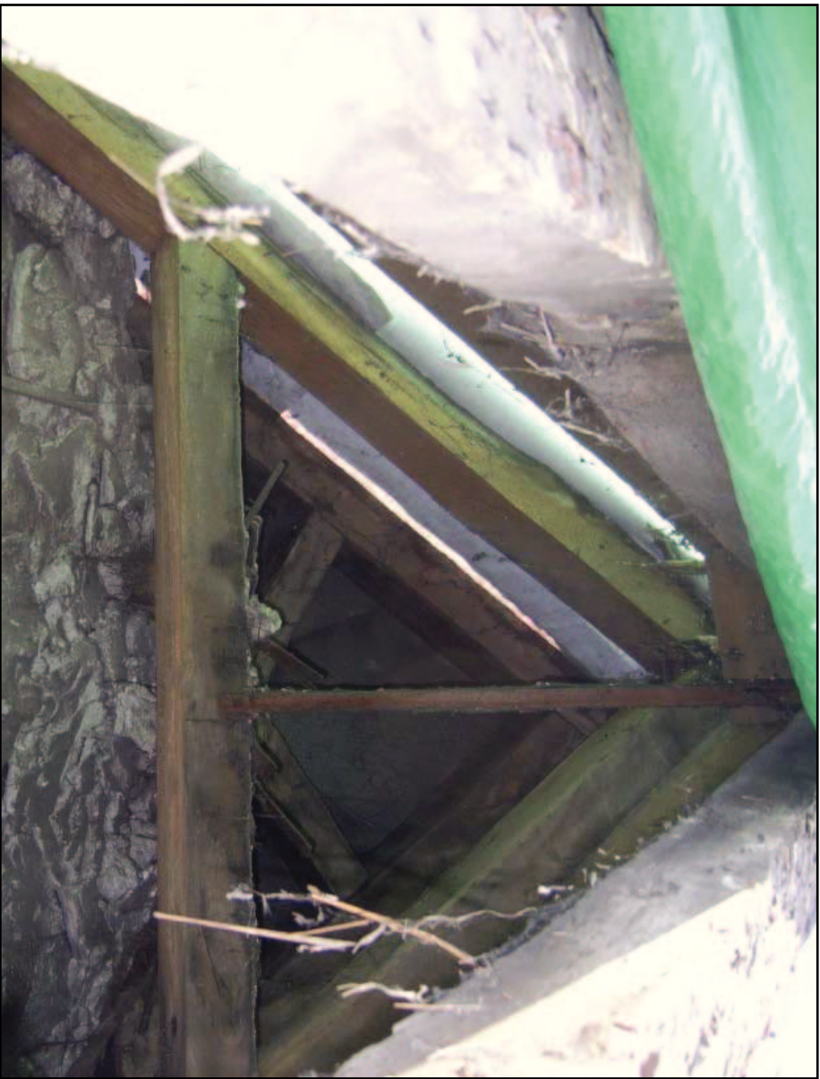
Plate 23: Roof apex at east end
