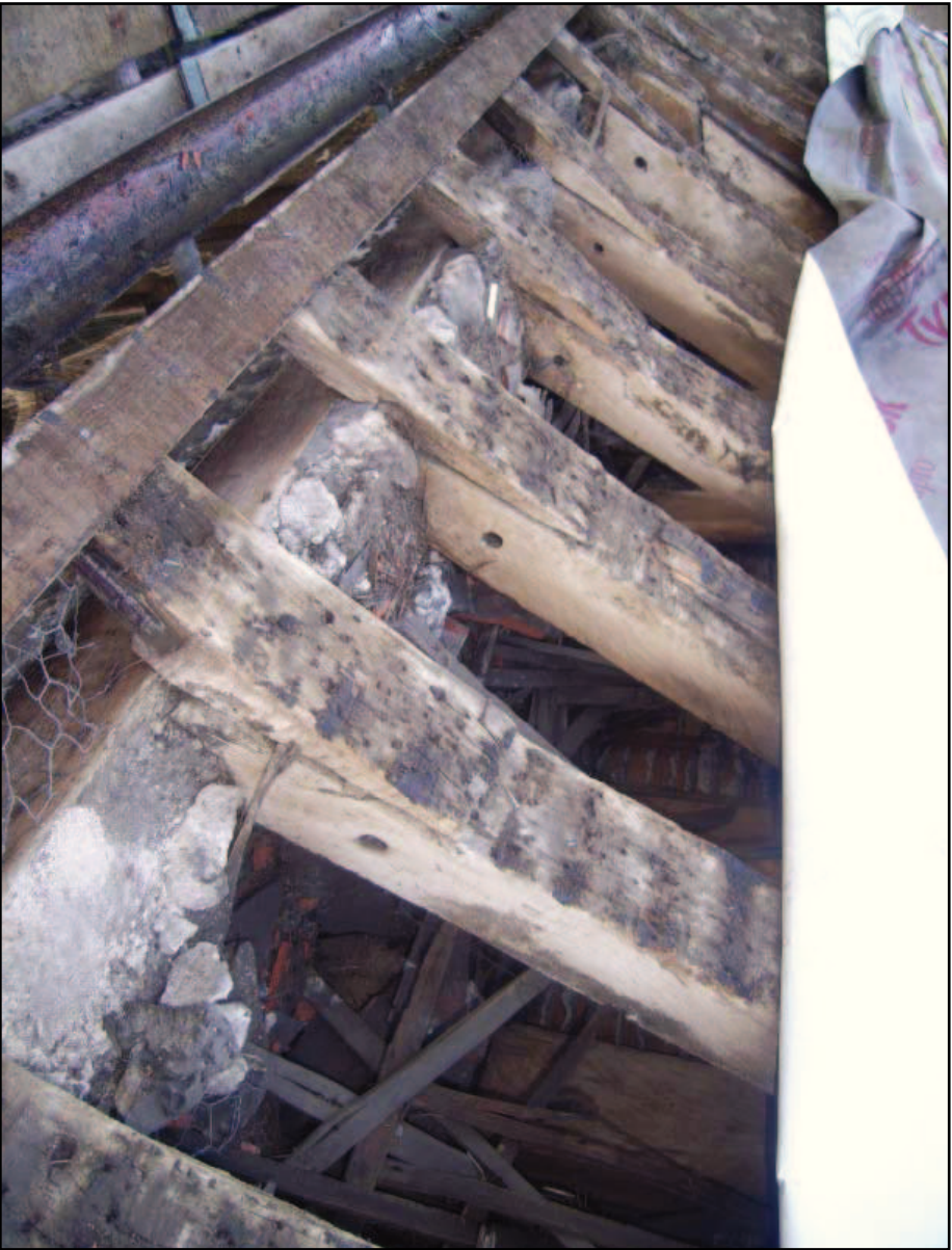
Plate 11: Rafter feet exposed on north side of roof
