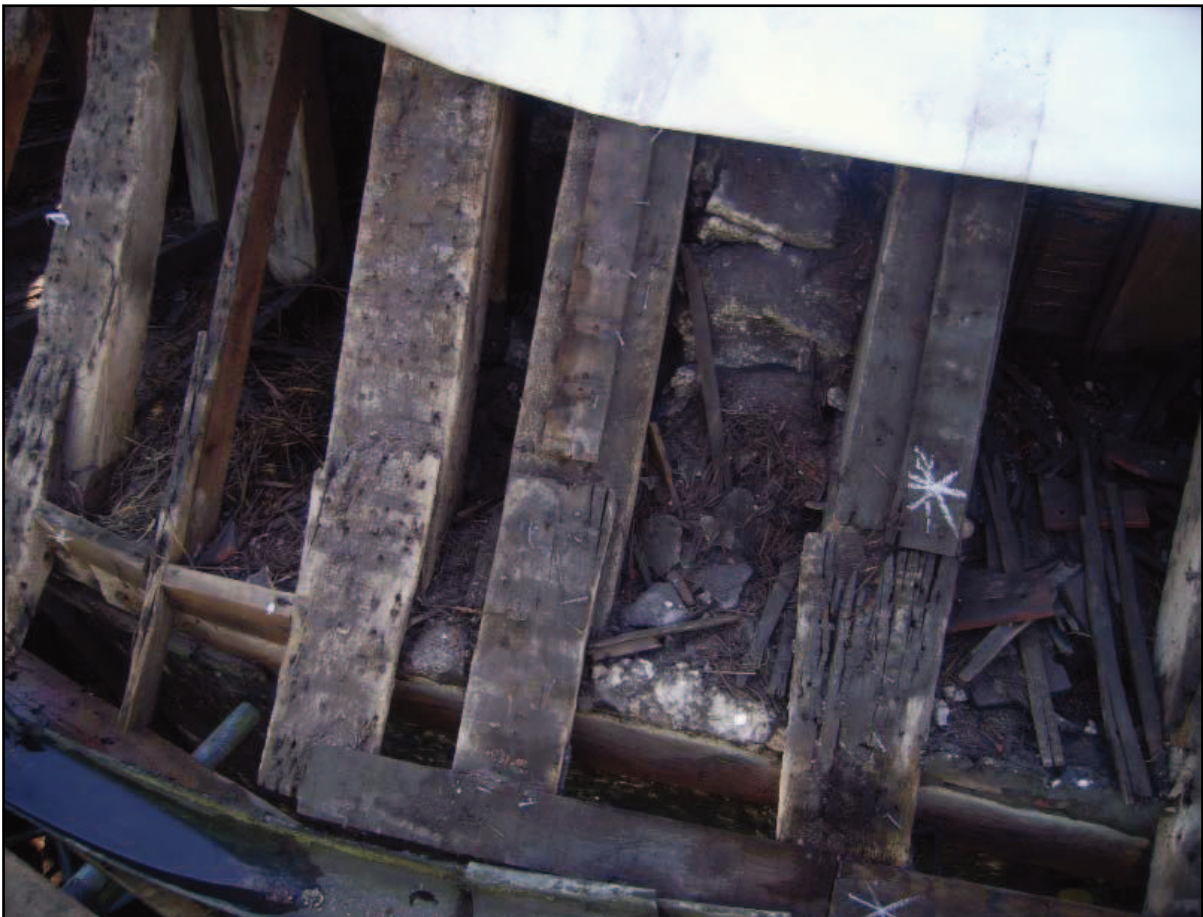
Plate 14: Three principal rafters at junction between apsidal roof and main roof.
