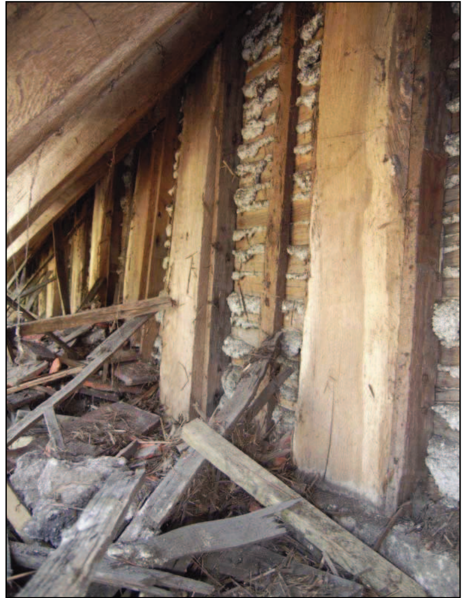
Plate 19: Ashlar studs along main part of roof
