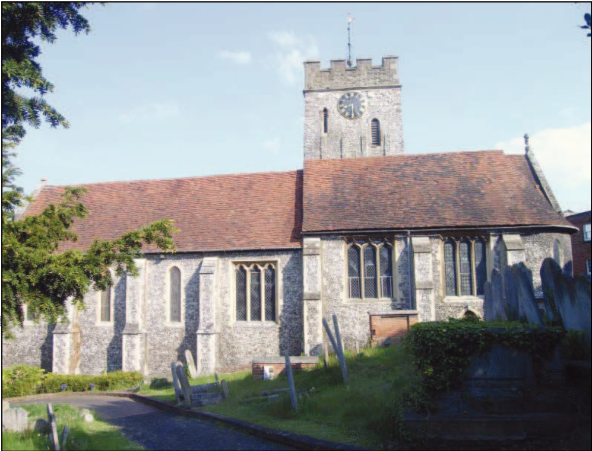
Plate 1: St. Mary's Church, general view
