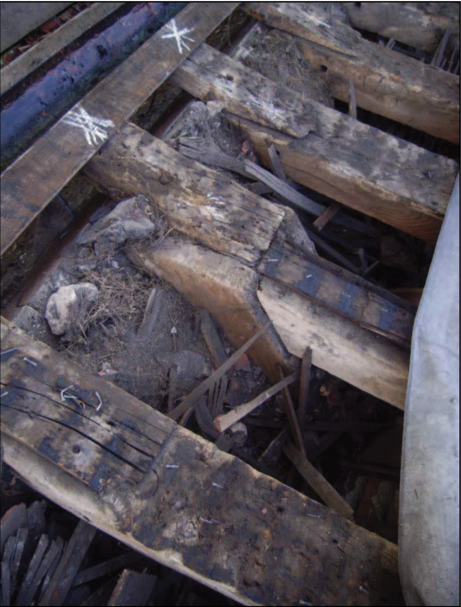
Plate 12: Tie-beam towards centre of chapel roof
