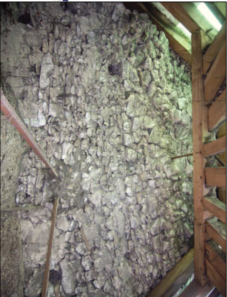
Plate 25: East face of wall between semi-circular end and main roof
