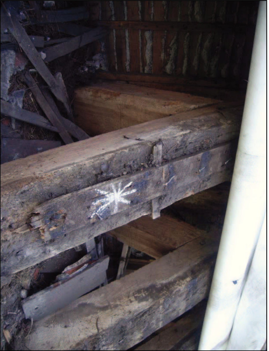
Plate 15: Rafter feed towards east end of main roof
