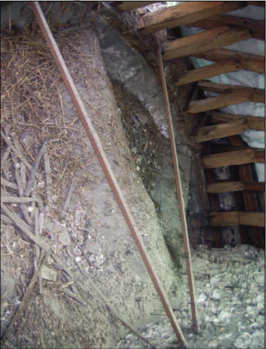
Plate 21: Tie rods in roof at east end
