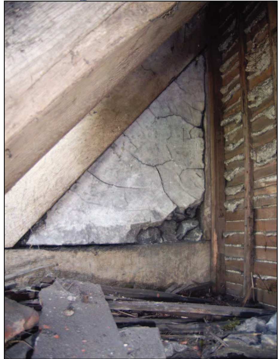
Plate 17: Plastered wall at east end of main roof
