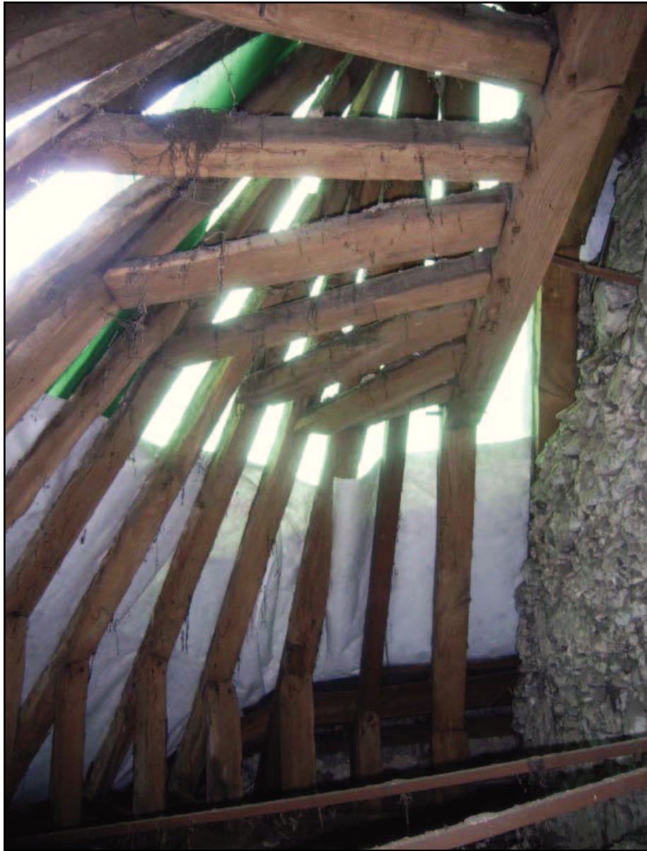
Plate 20: Roof at semi-circular east end
