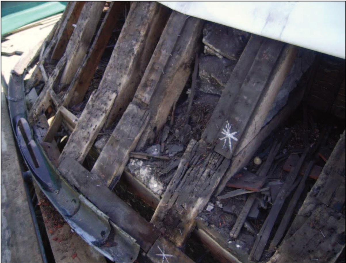
Plate 13: Rafter feet at semi-circular east end
