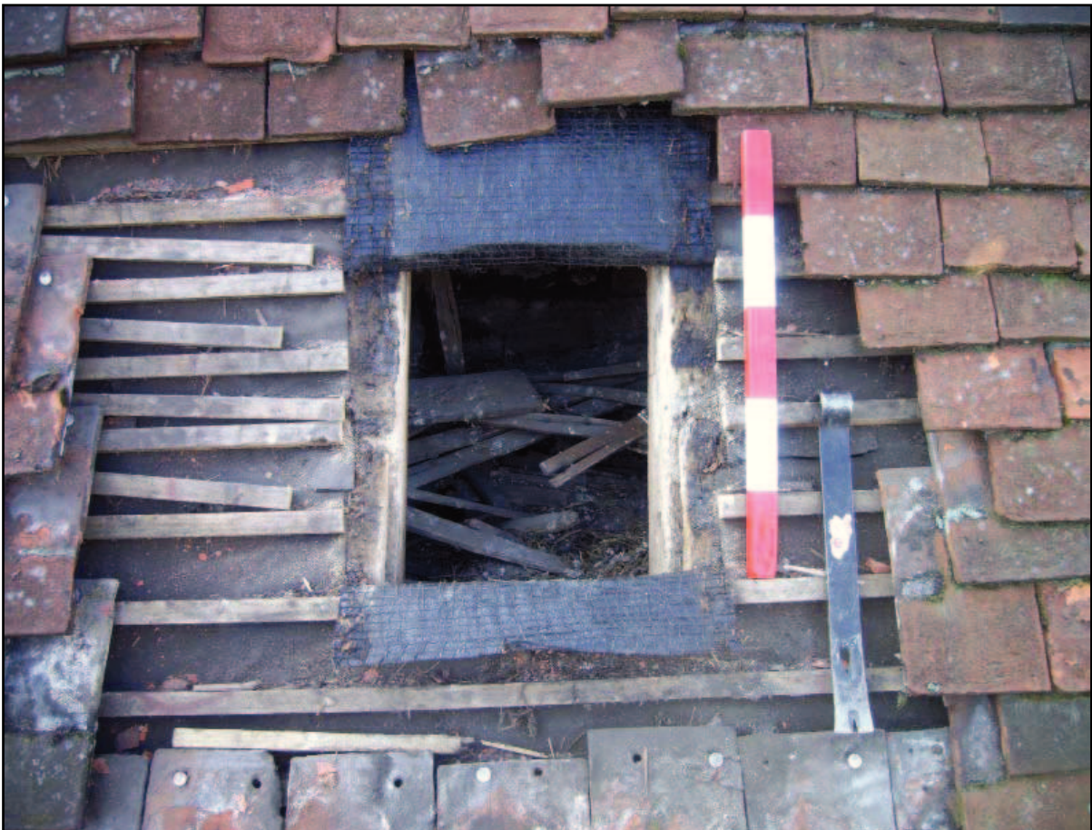
Plate 2: St. Mary's Church roof, showing pegged tiles and laths overlying joists
