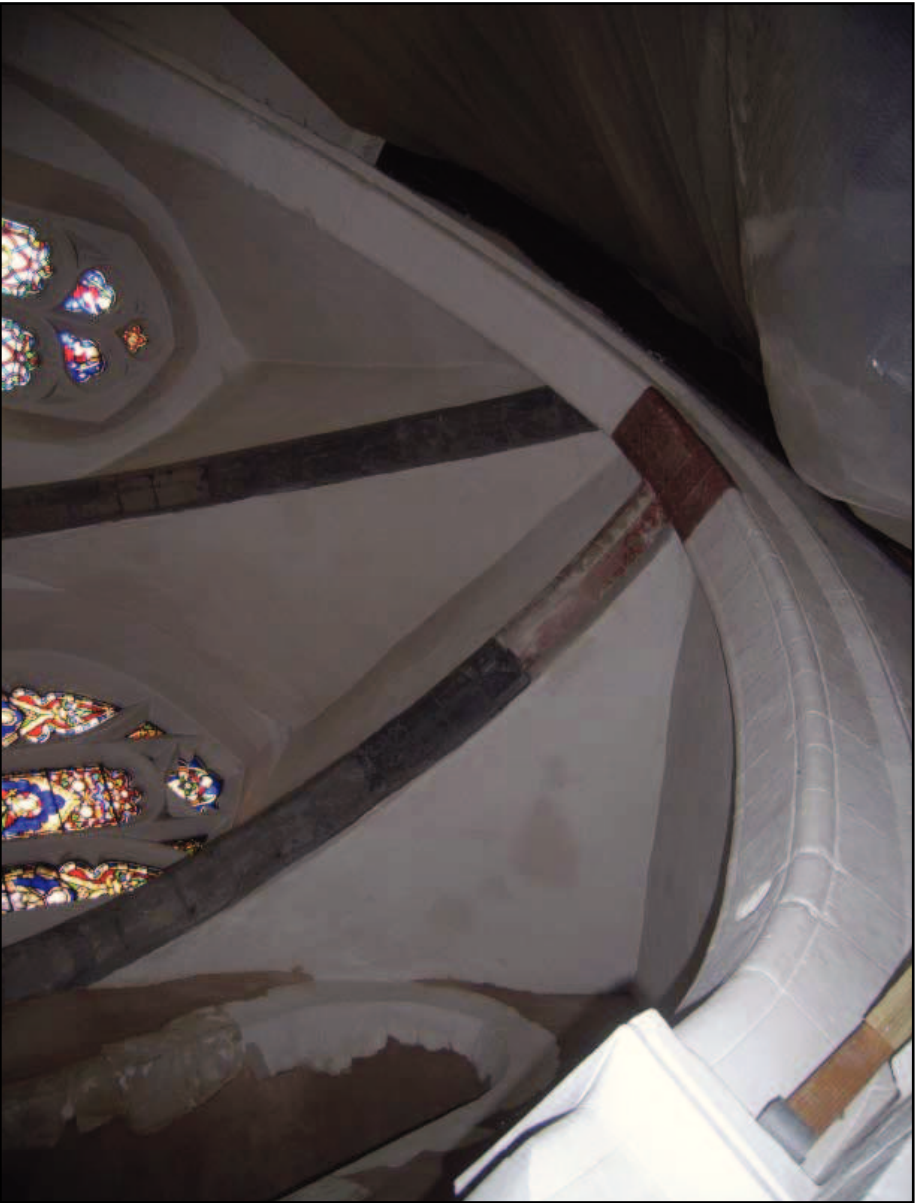
Plate 27: Vaulting in St John's Chapel
