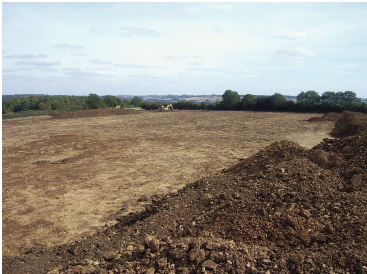
Plate 1: The quarry site after removal of topsoil and subsoil
