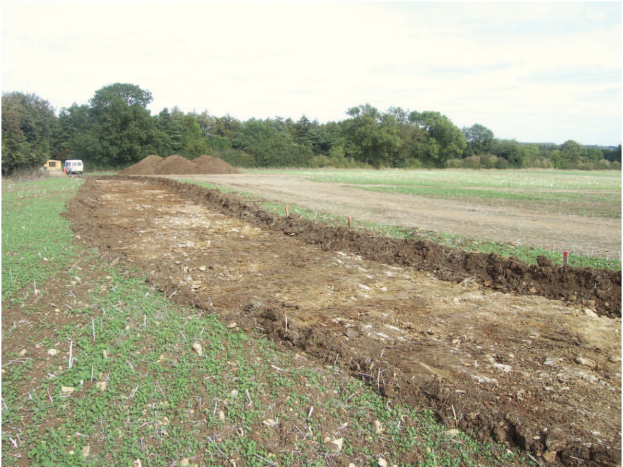
Plate 2: The haul road
