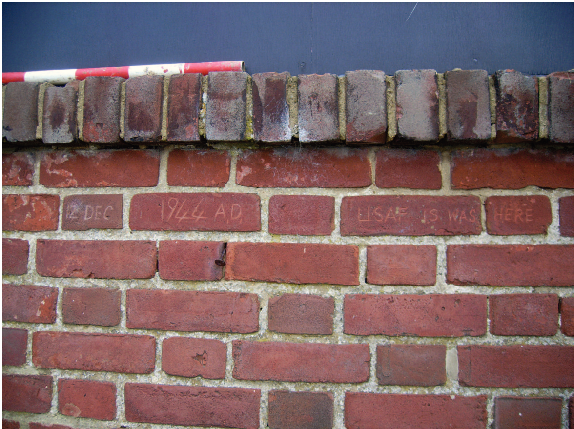
Plate 8: American Air Force graffiti on substation building
