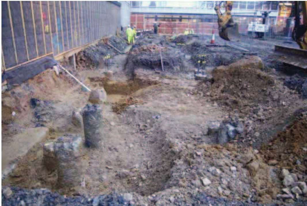
Building C: subsoil being mechanically reduced – natural sands exposed in ground beam and pile cap excavations, as well as profiles of both natural and subsoil being revealed
