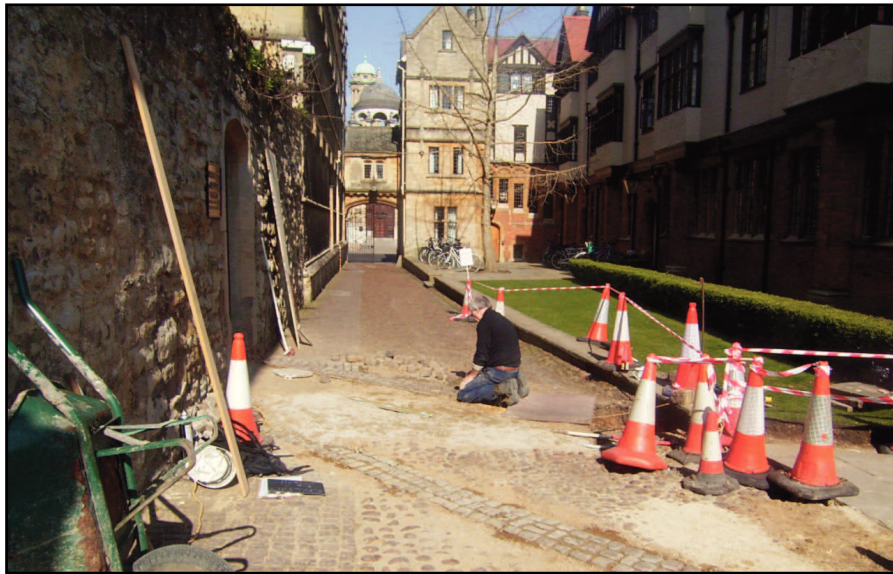
Plate 4: Logic Lane, looking north during works
