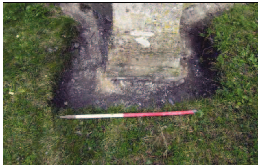
Plate 3: Shot of the excavated trench around footings, view looking north-west
