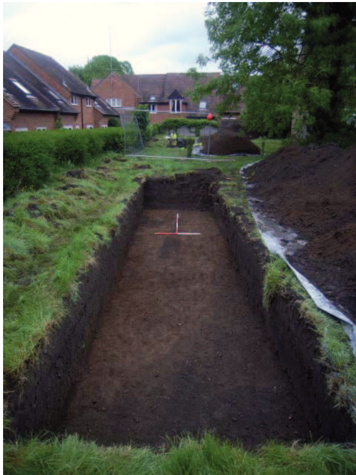
Plate 8: Trench 4 after machining and cleaning, looking east
