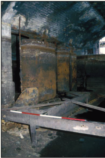
Plate 13: North-east view of box weirs at east termination of precipitation lanes
