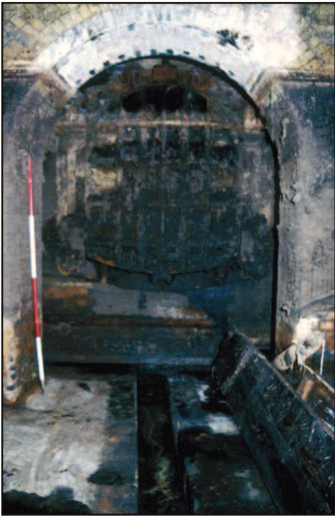
Plate 11: Penstock at south-west termination of precipitation lane
