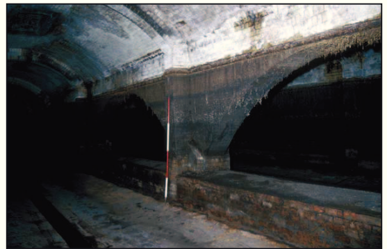
Plate 8: Internal north view of open arches dividing precipitation lanes
