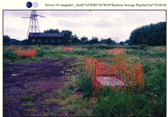
Plate 2: North-west view of covered precipitation lanes showing vents
