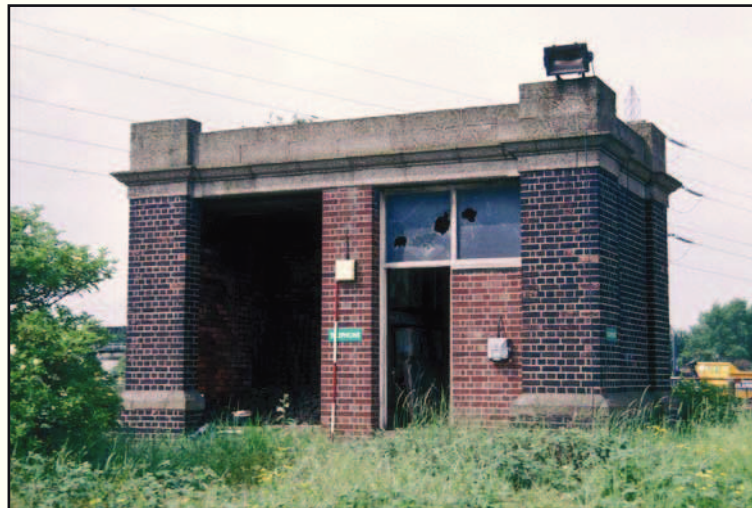
Plate 39: South-west view of Penstock Controller House
