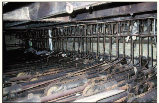
Plate 31: Internal north-east view showing the Valve House basement
