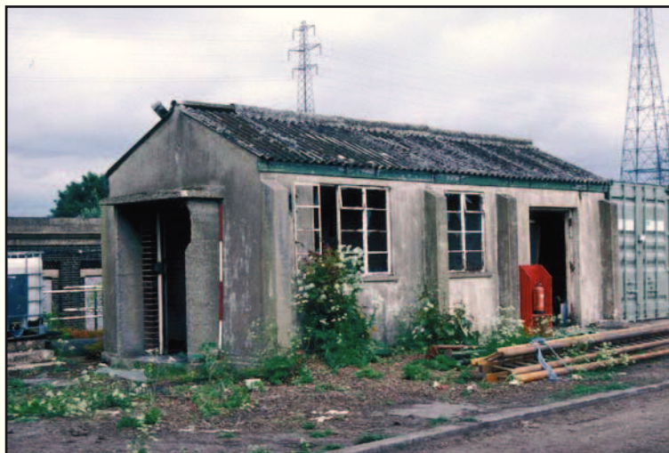
Plate 40: North-east view of administration building
