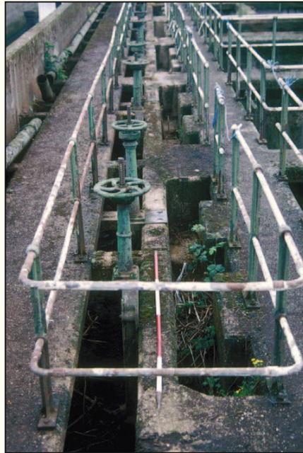
Plate 22: South view of penstocks at east
