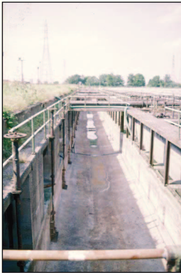
Plate 26: South view of weir chamber
