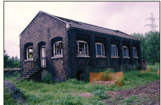
Plate 27: North view of valve house
