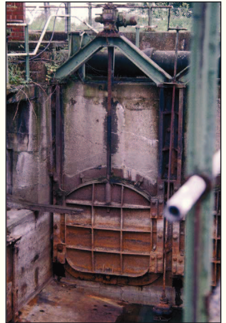
Plate 23 North view showing weir chamber penstocks
