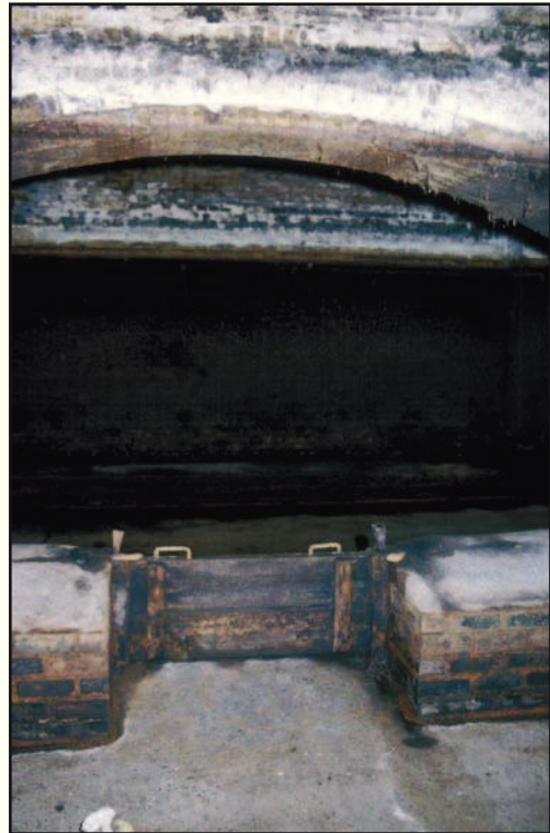
Plate 10: Internal north view of precipitation lanes showing partition walls and wooden gates
