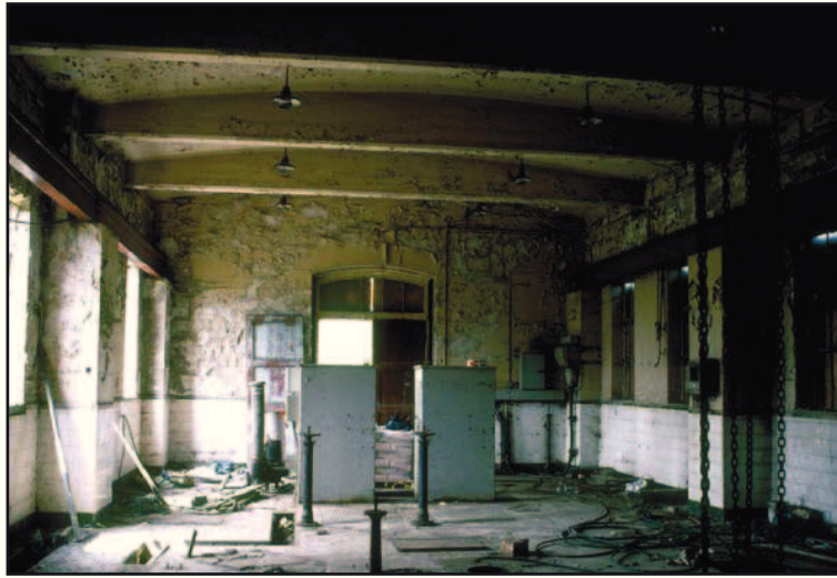
Plate 35: Internal west view of Drainage Pumping Station no.2
