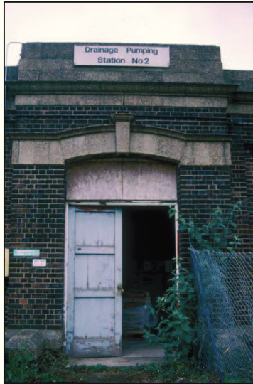
Plate 34: East view showing entrance of Drainage Pumping Station no. 2
