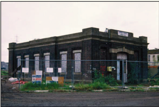
Plate 32: South-east view of Drainage Pumping Station no.2
