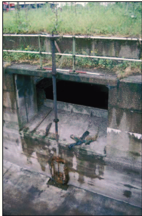
Plate 12: South-west view of weir chamber penstock
