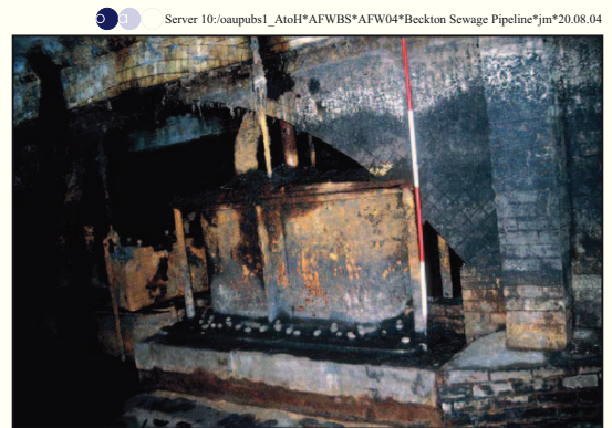
Plate 14: North view of weir located in south-west length of precipitation lanes
