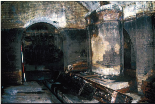
Plate 15: Box weir located at south-west termination of precipitation lanes
