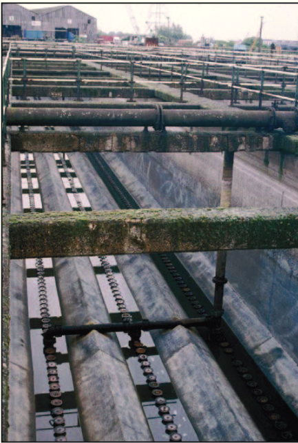
Plate 21: East view showing base of re-aeration lanes
