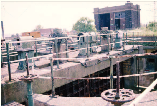
Plate 24: West view of venturi channel penstocks
