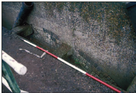
Plate 18: North-east view of blocked precipitation lane arch at east termination of re-aeration lanes
