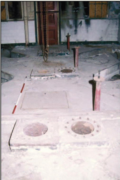
Plate 36: Internal east view of square platforms within Drainage Pumping Station no. 2
