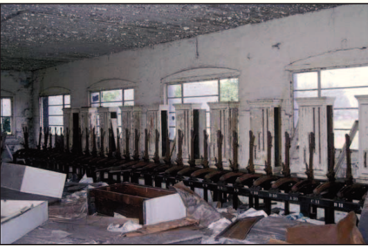
Plate 30: Internal north-east view showing upper room of Valve House
