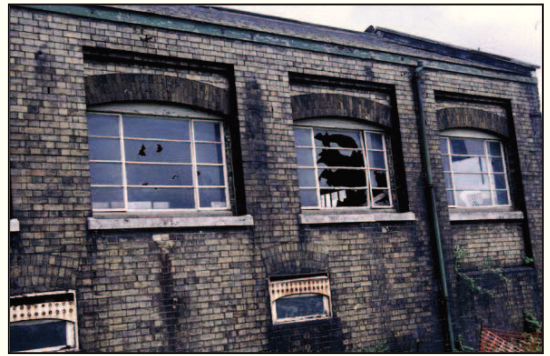
Plate 29: Valve House windows, south-west elevation
