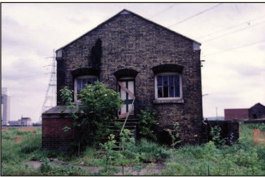
Plate 28: Valve House, south-west elevation
