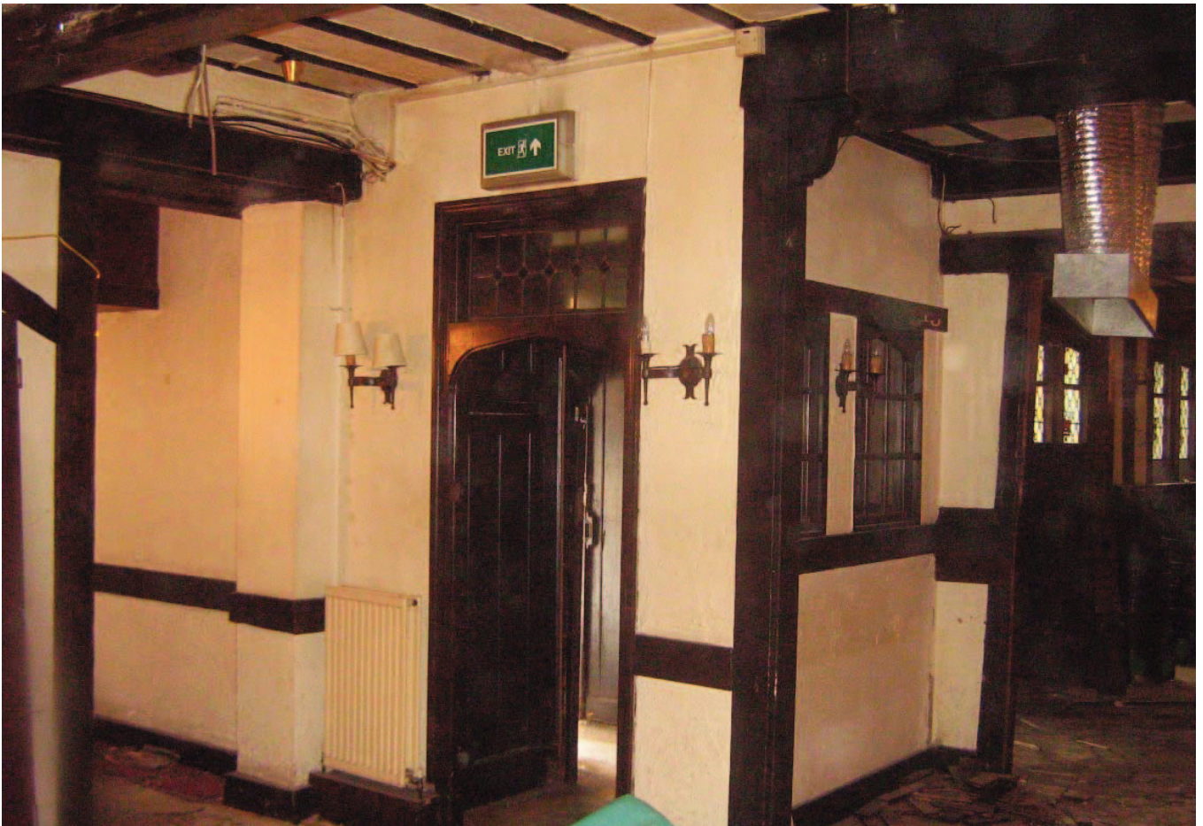
Plate 24: Entrance lobby in Area 4 looking towards south-east.
