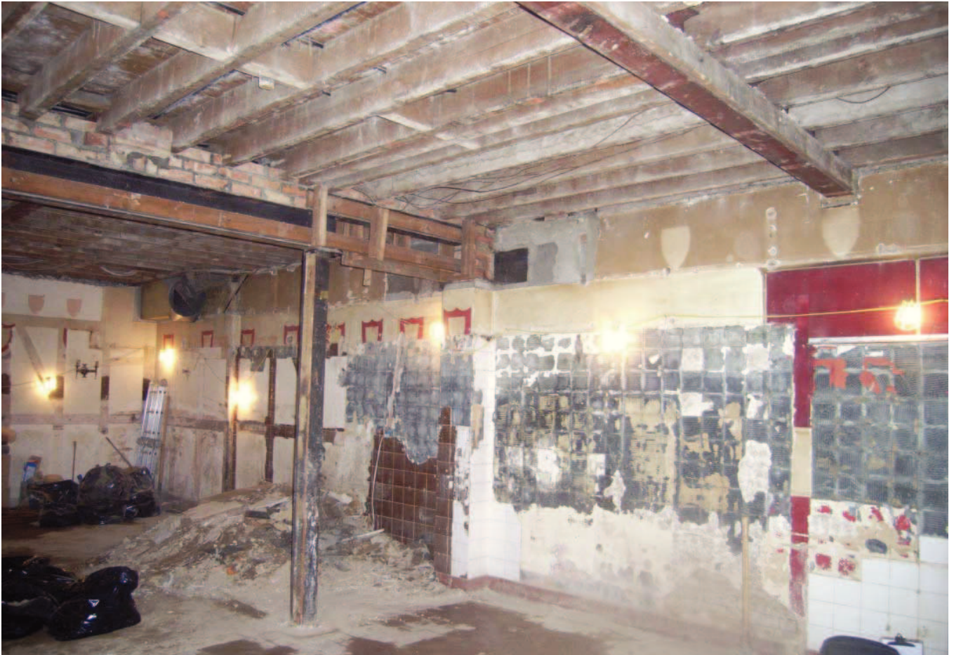
Plate 19: Area 4 and 5 after removal of partition
