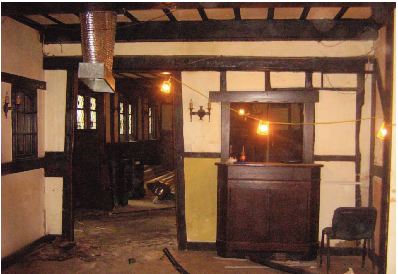
Plate 10: Interior looking south at start of current work
