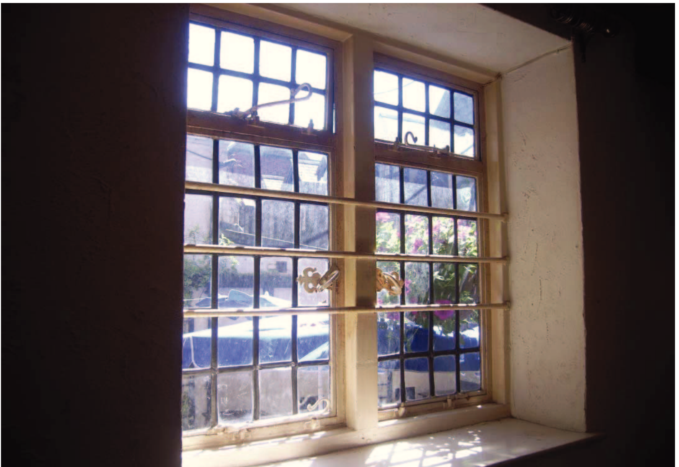
Plate 8: Window latches in North Range
