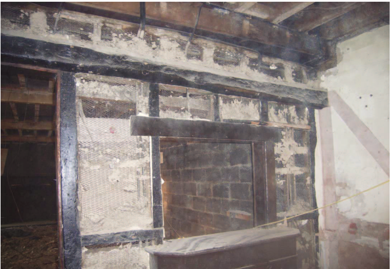
Plate 12: North side of historic frame after partial clearance of 20th-century plaster
