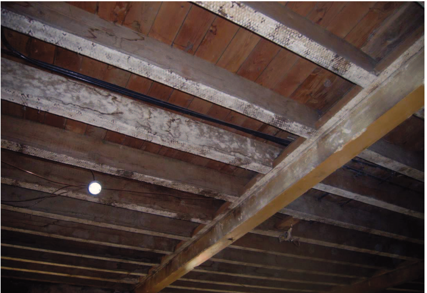
Plate 22: Ceiling in Area 3 after soft strip
