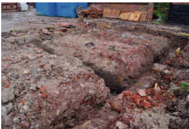
Plate 11: Trenches at west end of House 4
