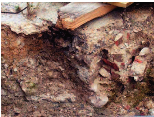
Plate 2: Construction feature in Service Trench B to north of barn
