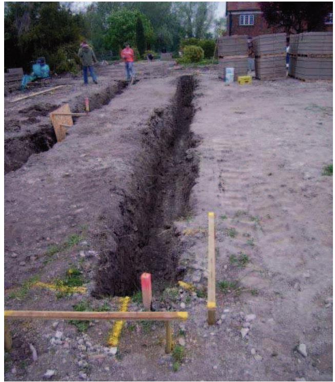
Plate 6: General view from south of excavations for House 3
