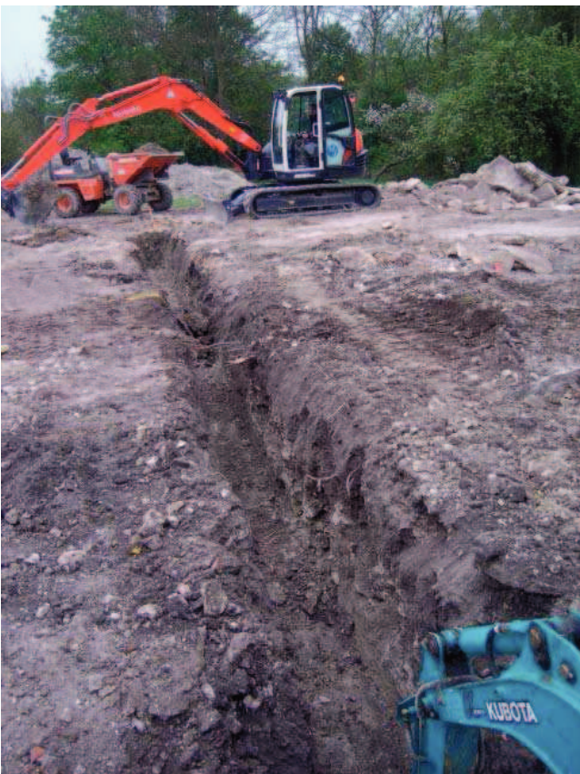
Plate 7: Foundation trench (N-S) for House 3
