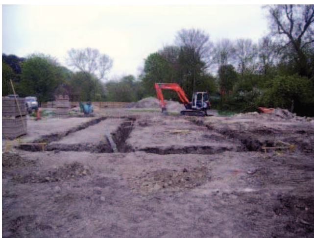
Plate 3: General view of excavations for House 3
