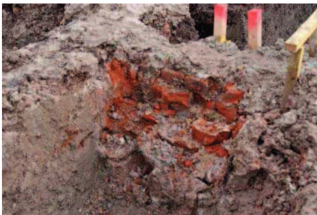
Plate 9: Stub of brick wall towards centre of excavations for House 4
