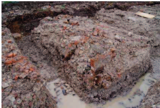
Plate 14: View from south of trenches in House 4 including remains of WC
