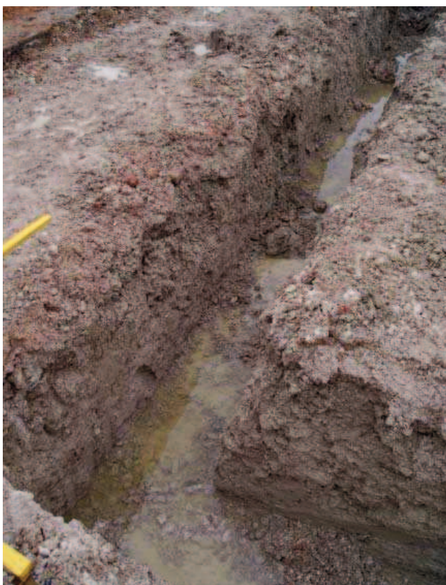
Plate 19: Foundation trench at south-west corner of East Range of House 4
