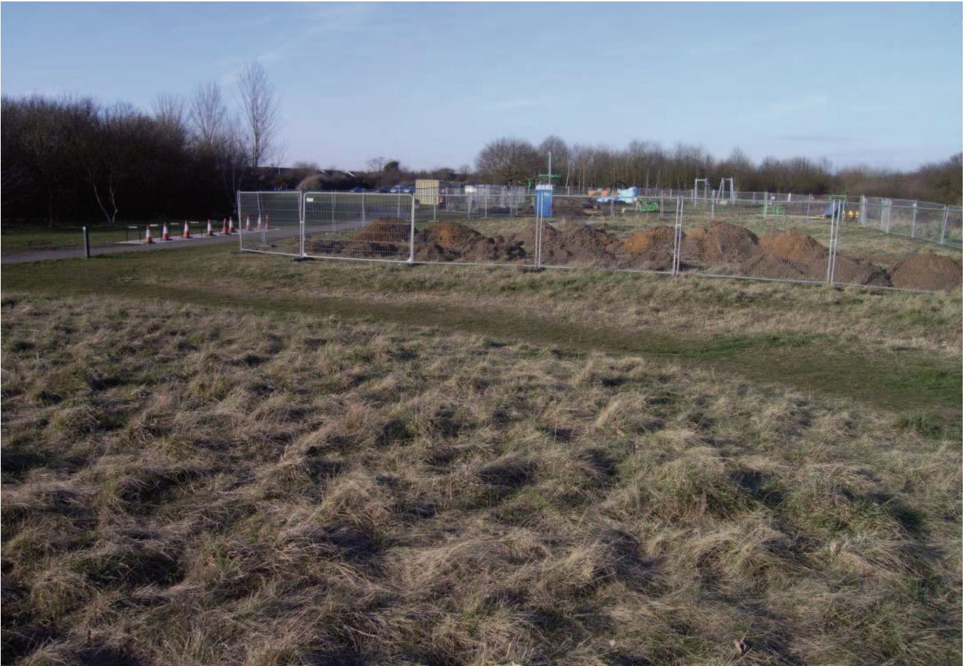
Plate 5: General view of area investigated
