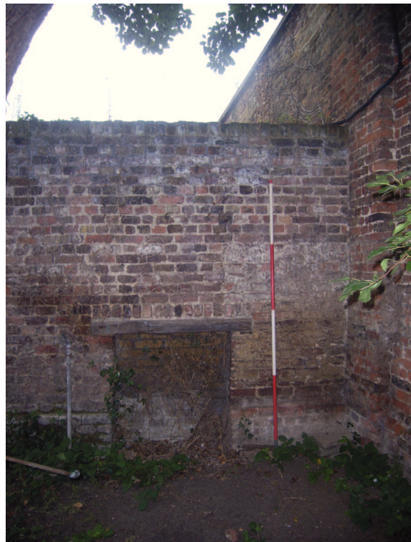
Plate 8: View of infilled opening on section 3, east facing elevation
