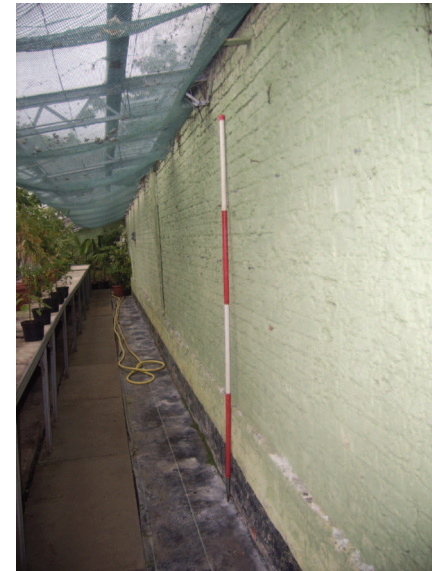
Plate 16: View of section 3, west facing elevation
