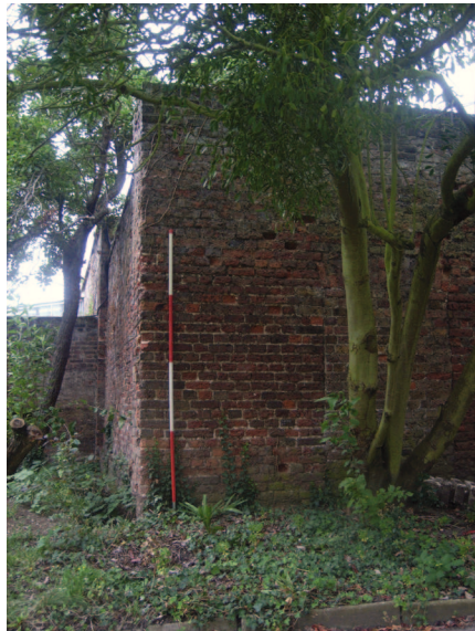
Plate 3: Detail of south end of east facing elevation
