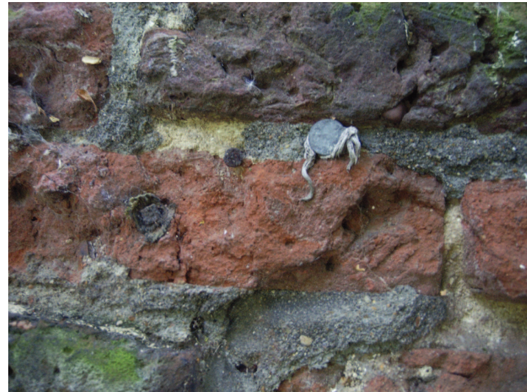
Plate 20: Detail of planting fixing Section 1 east facing elevation
