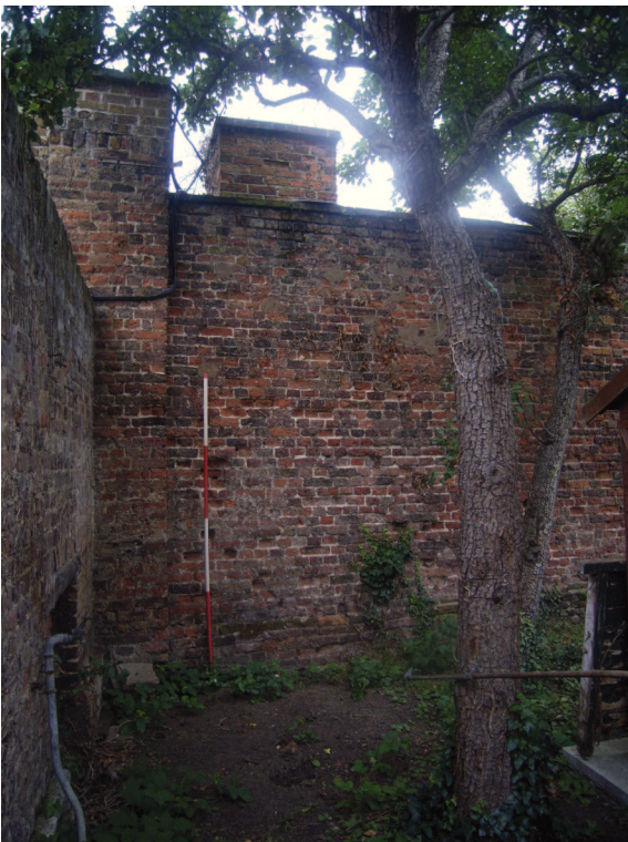
Plate 7: View of west end of south facing elevation
