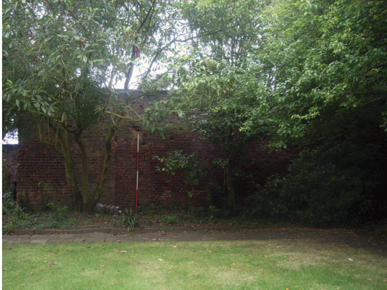
Plate 1: View of section 1 east facing elevation
