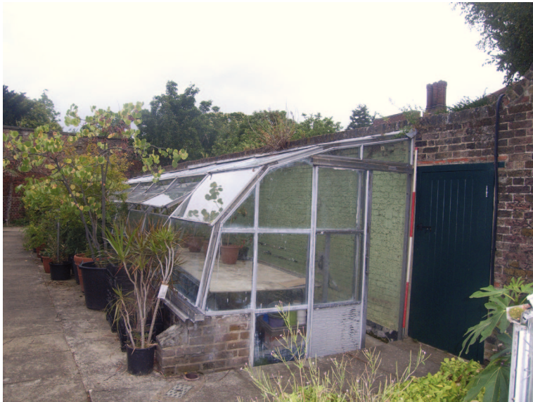
Plate 15: View of greenhouse on section 3, west facing elevation
