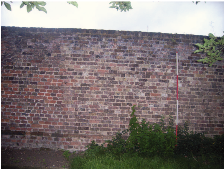
Plate 11: Detail of changing brickwork on section 3, east facing elevation
