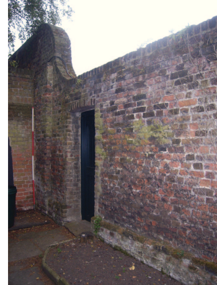
Plate 14: View of gate on section 3, east facing elevation
