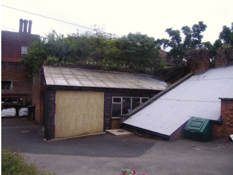
Plate 17: View of garage/store, section 1 and 2
