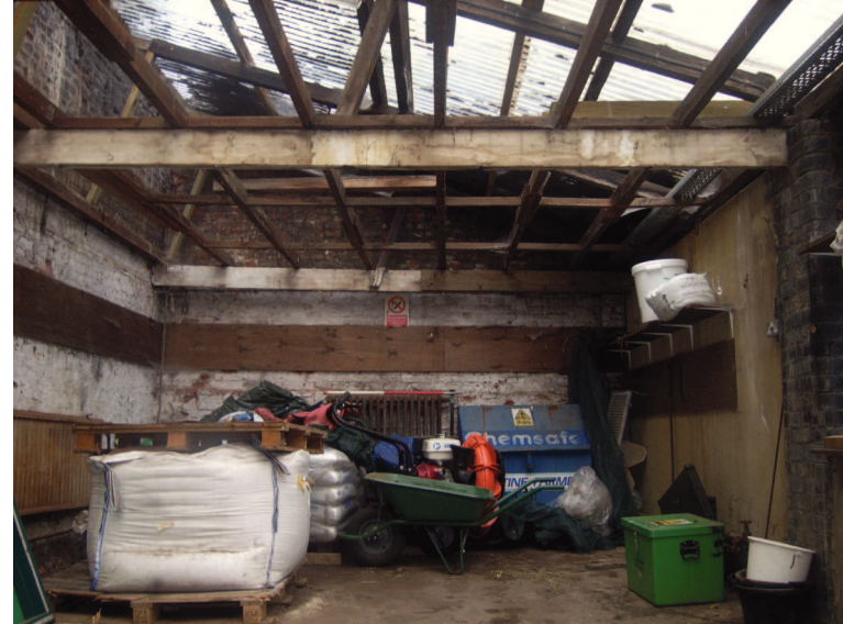
Plate 18: View of garage/store, section 2
