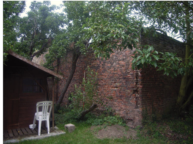
Plate 4: View of section 2 south facing elevation
