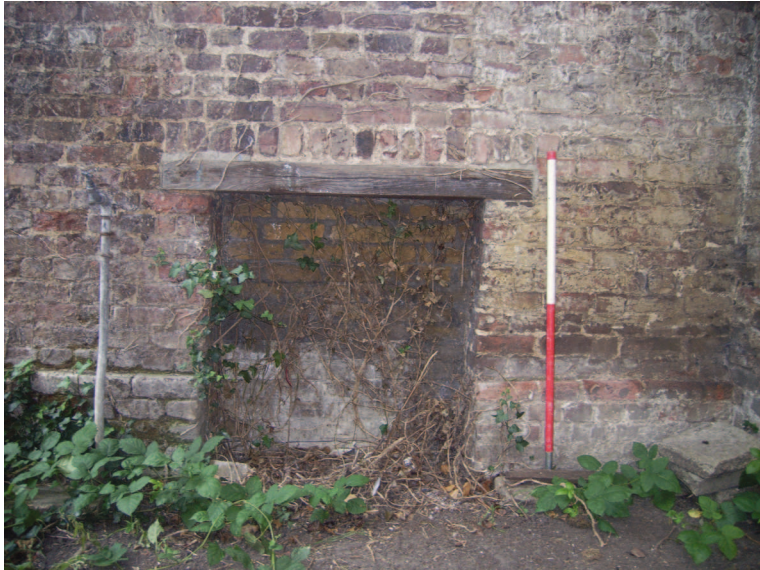
Plate 9: Detail of infilled opening on section 3, east facing elevation
