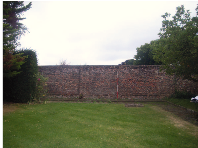
Plate 12: View of section 3, east facing elevation
