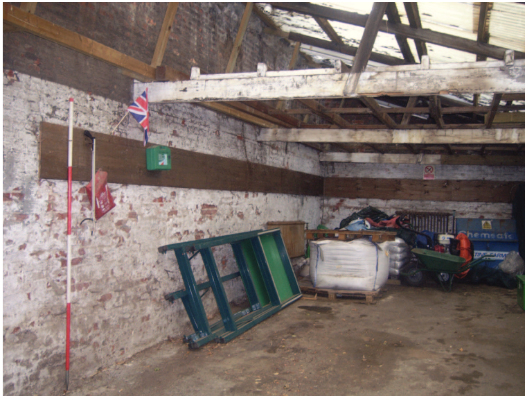
Plate 19: View of garage/store, section 1
