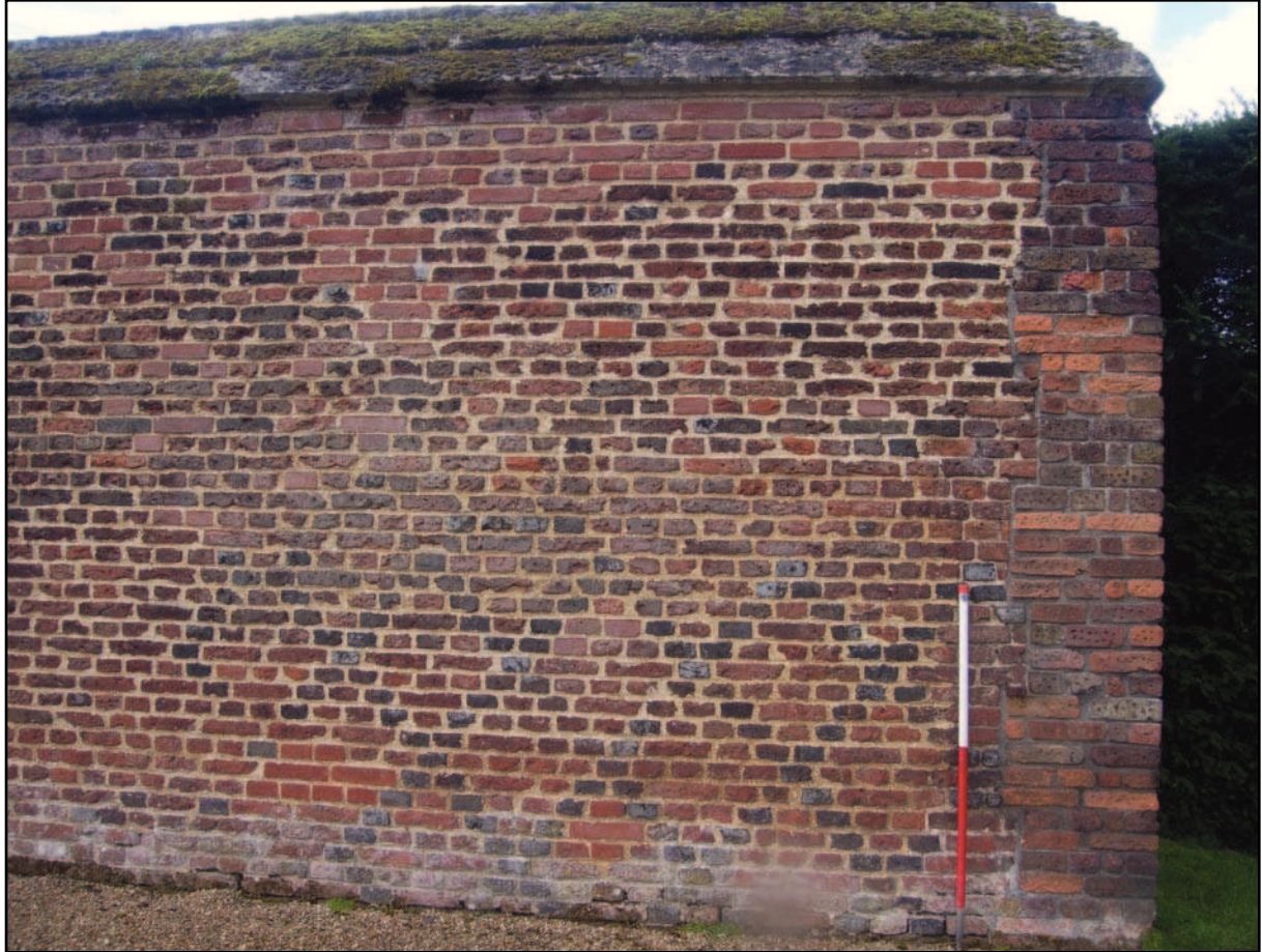
Plate 12: Tudor diaperwork and later rebuilt corner on north west end of wall
