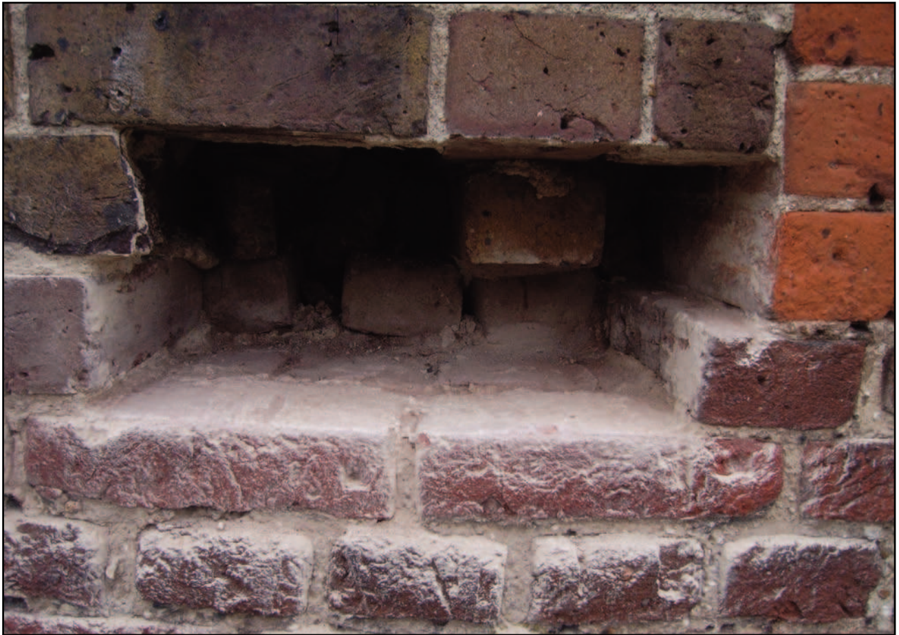
Plate 27: Opening up of lower infill brickwork on south west elevation
