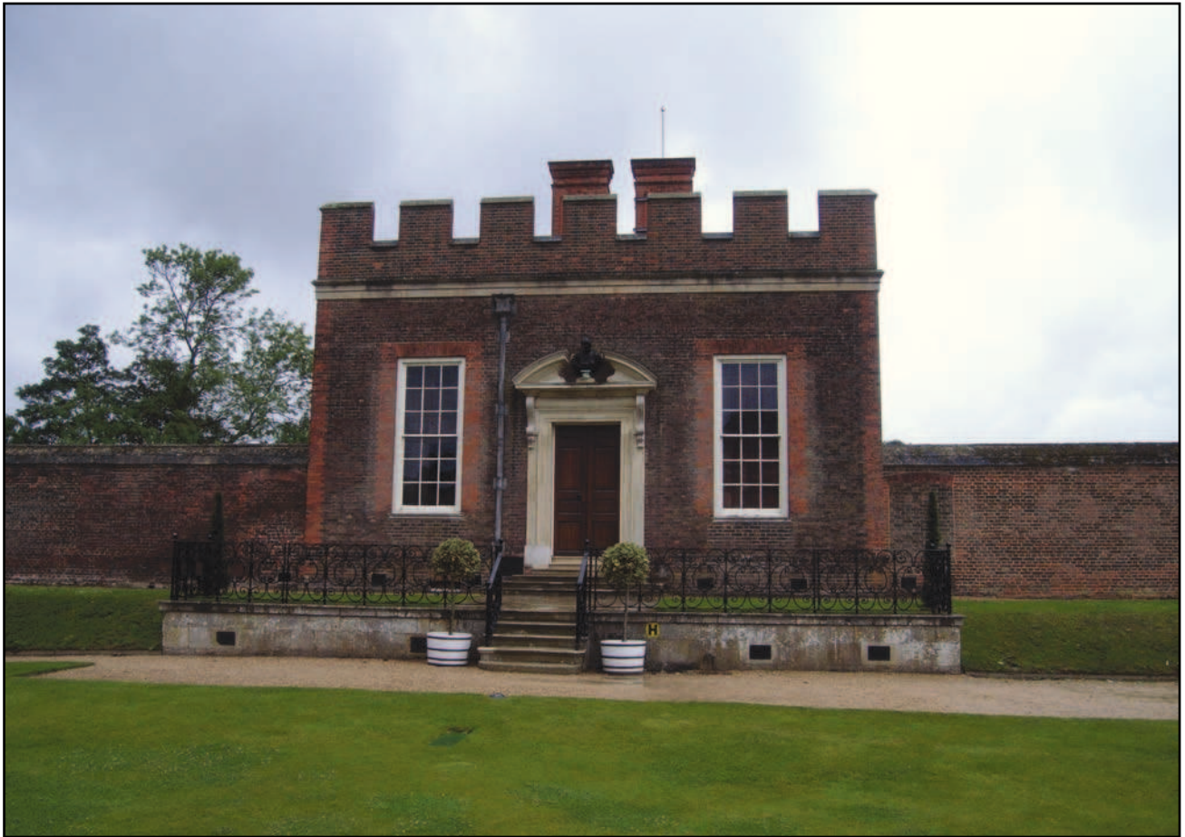
Plate 3: The Banqueting house west elevation
