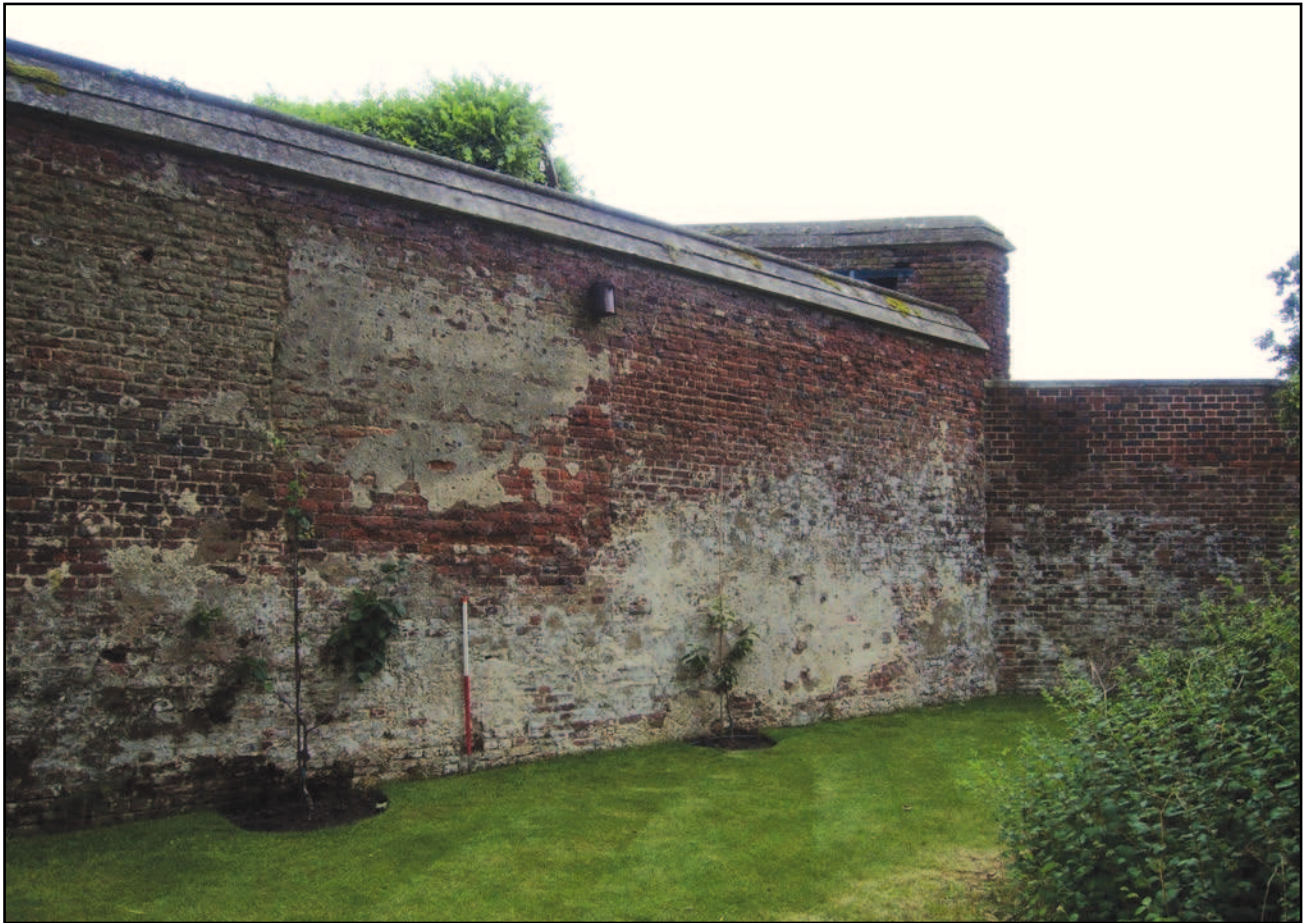
Plate 21: View of large infill patch on south east elevation and southern garden wall
