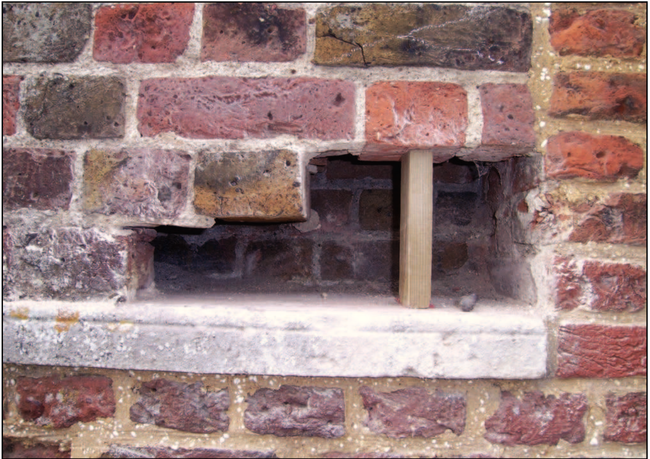
Plate 23: Opening up of lower infill brickwork on north west elevation
