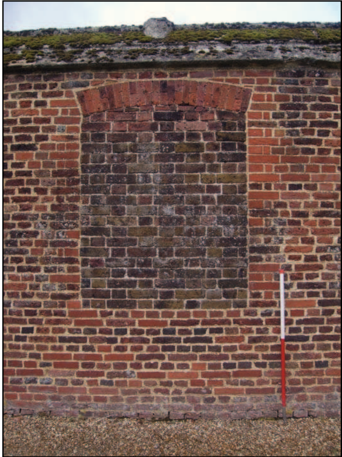
Plate 9: Infilled window opening on north west elevation of wall
