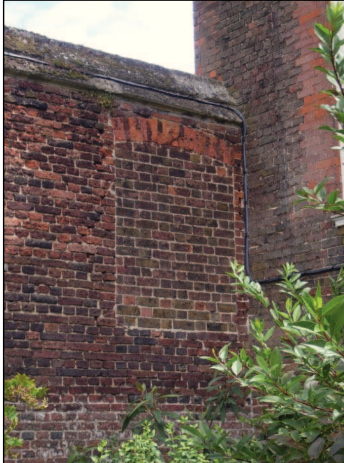
Plate 16: North east elevation detail of infilled window beside Banqueting House
