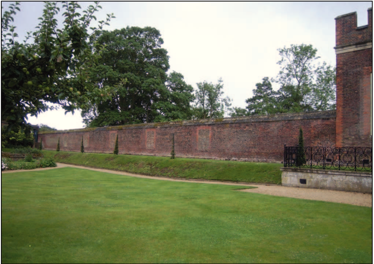
Plate 1: View of south west elevation of wall
