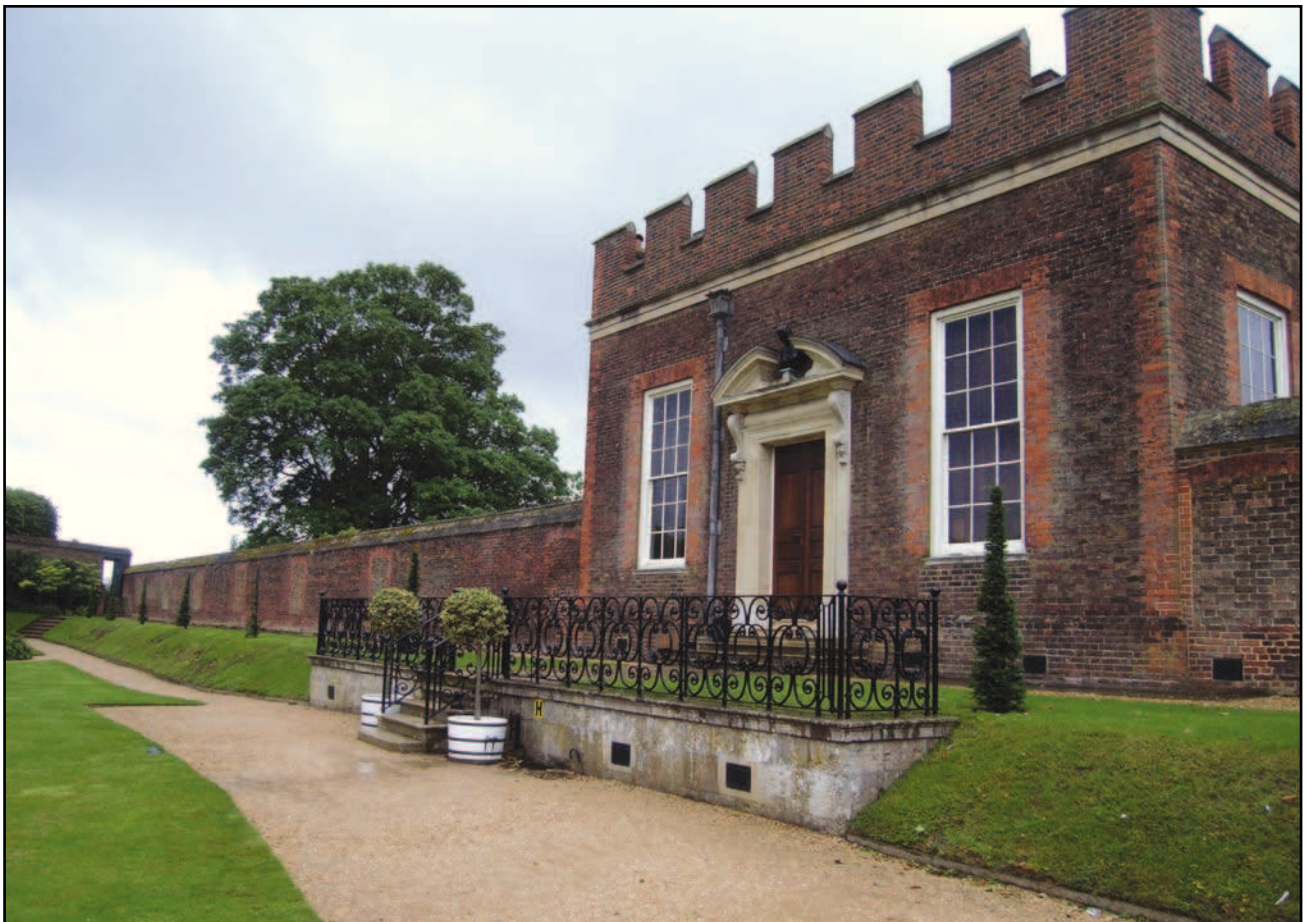
Plate 2: View of south west elevation of wall and Banqueting House
