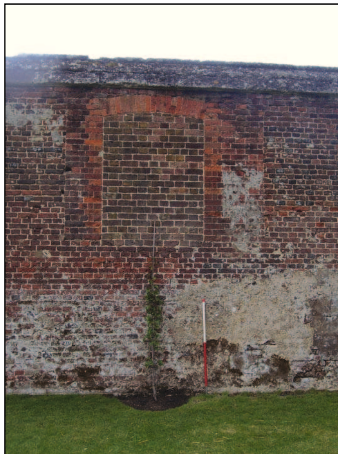
Plate 20: South east elevation detail of infilled window
