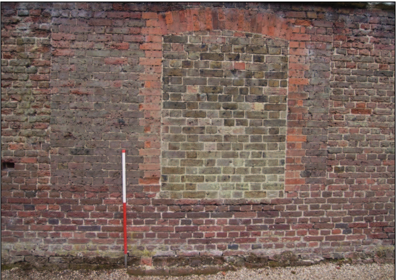
Plate 6: Infilled window opening on south west elevation of wall
