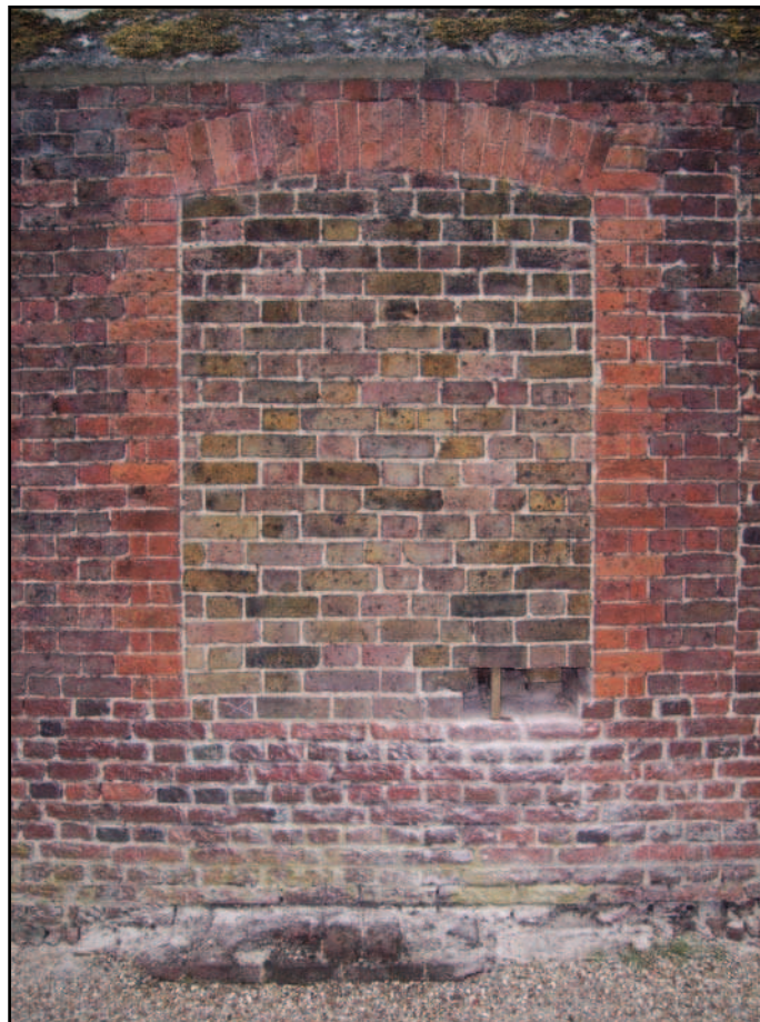
Plate 28: View of infilled window following opening up on south west elevation
