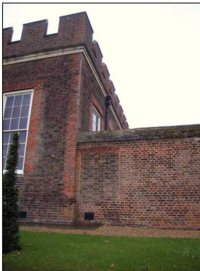
Plate 8: Infilled doorway on north west elevation of wall
