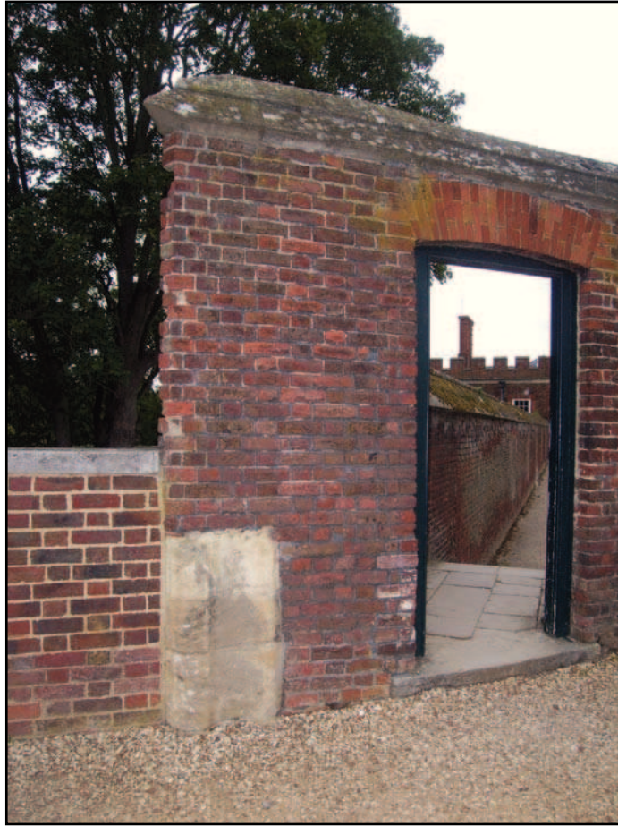
Plate 11: Moulded stone quoins on south garden wall
