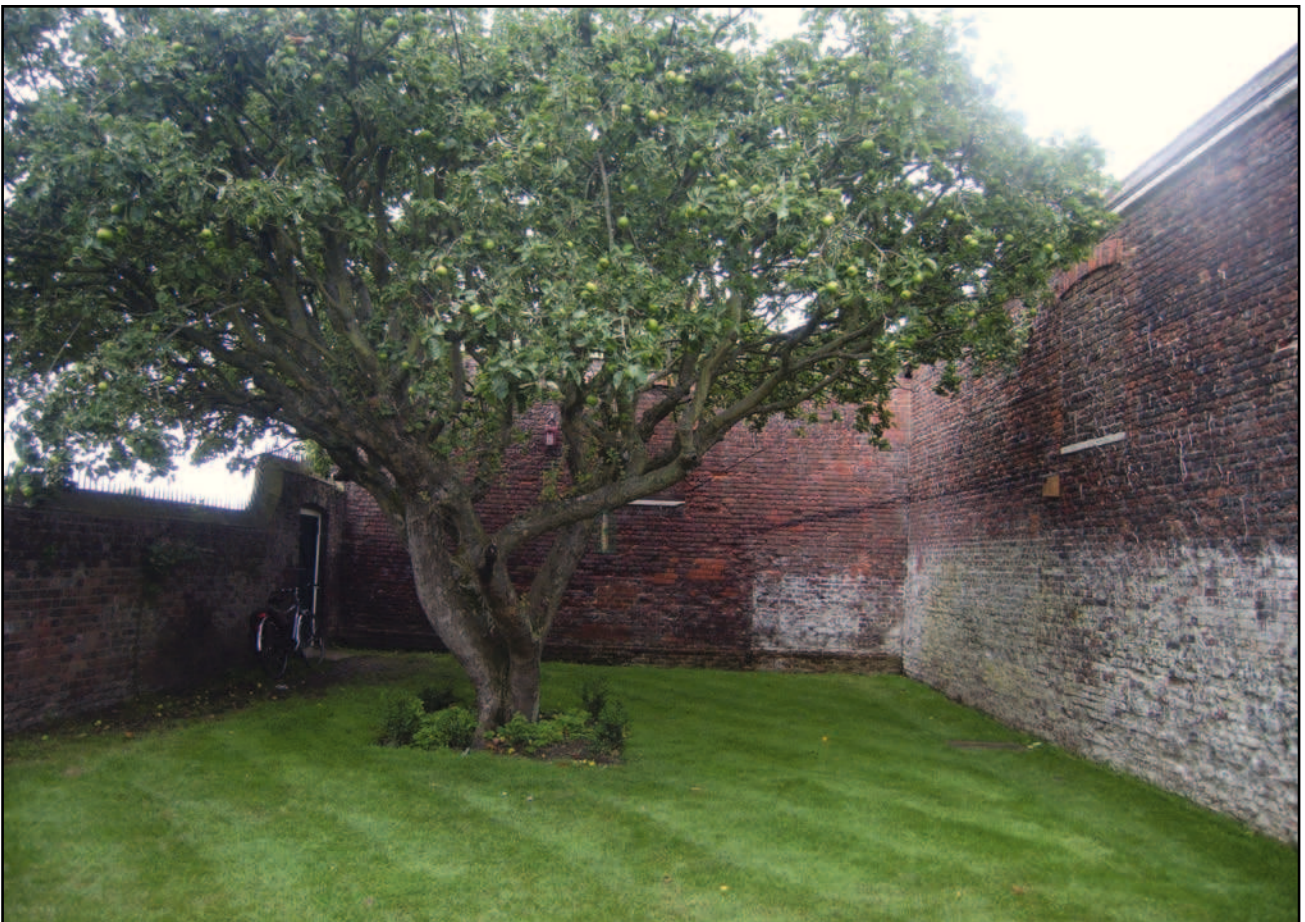
Plate 18: View of north elevation of garden wall showing extent of former lean to
