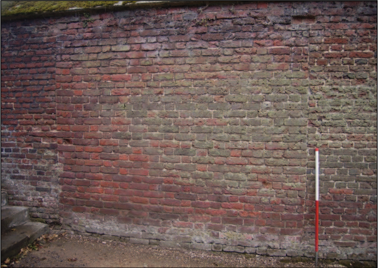
Plate 5: Infilled opening adjacent to south west garden stairs
