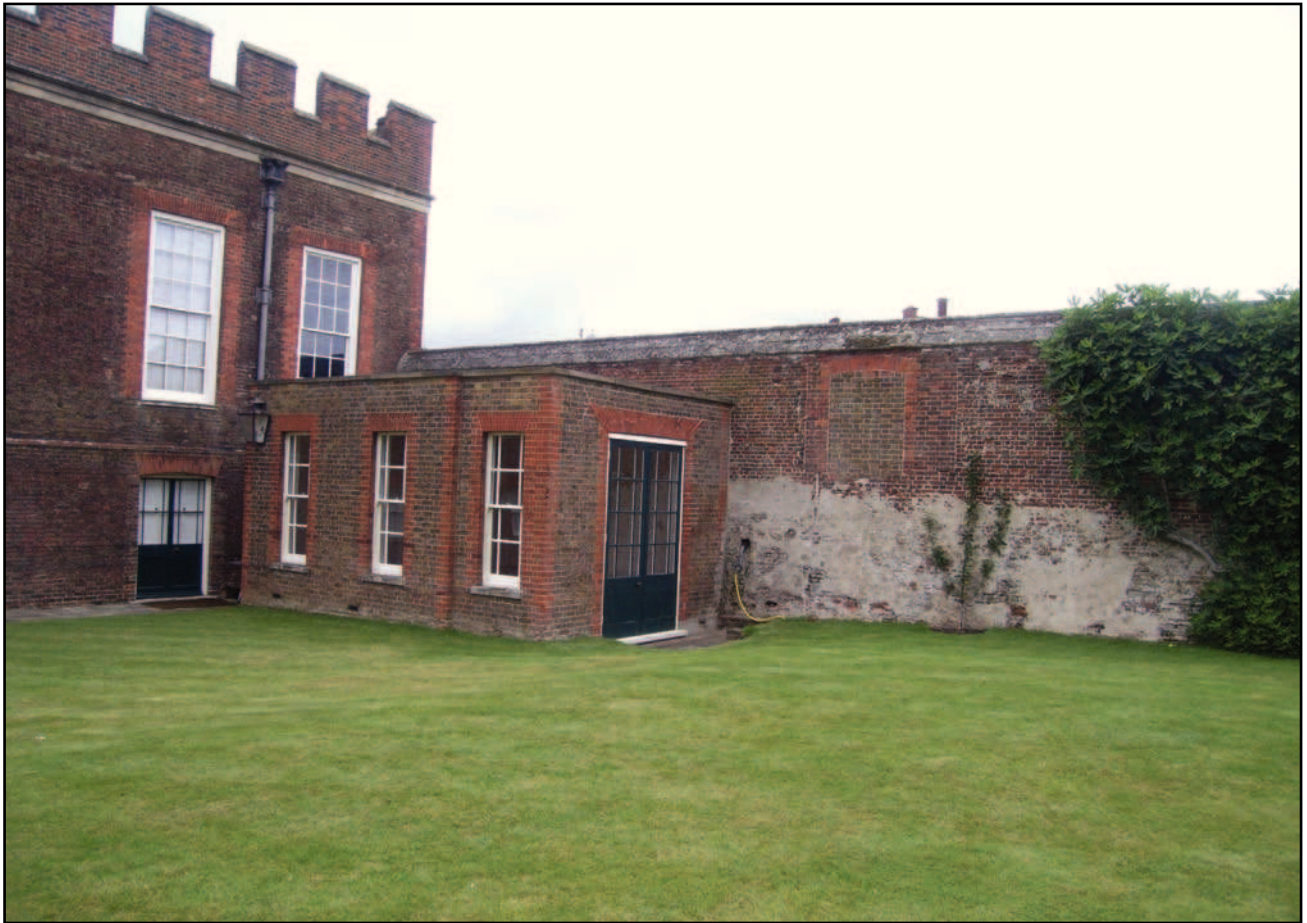
Plate 19: View of south east elevation
