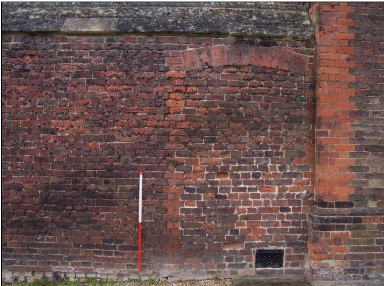
Plate 7: Infilled doorway on south west elevation of wall
