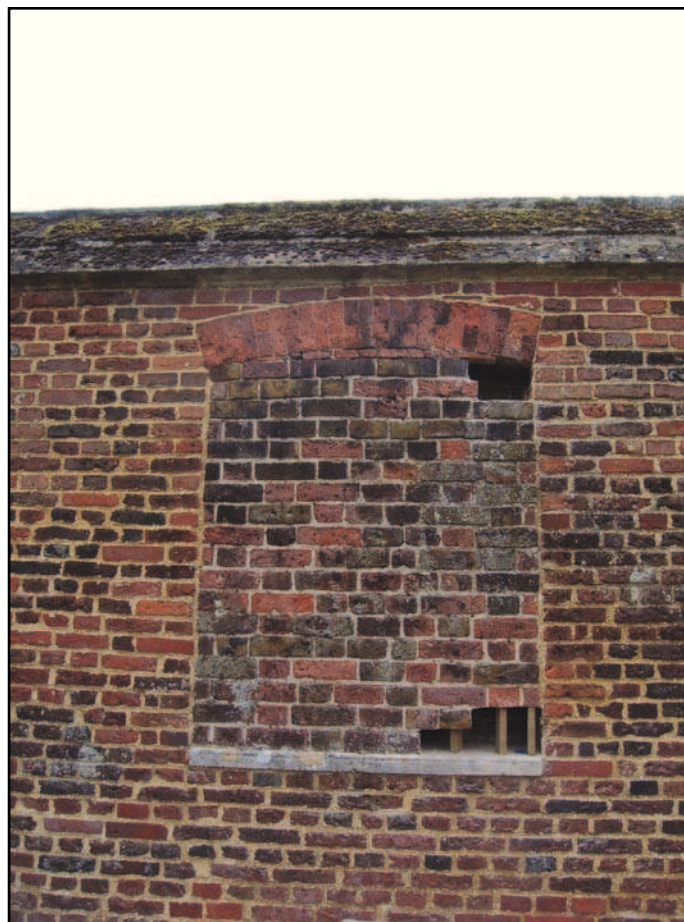
Plate 26: View of infilled window following opening up on north west elevation
