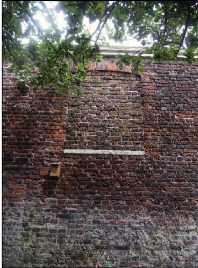
Plate 15: North east elevation detail of infilled window with stone sill
