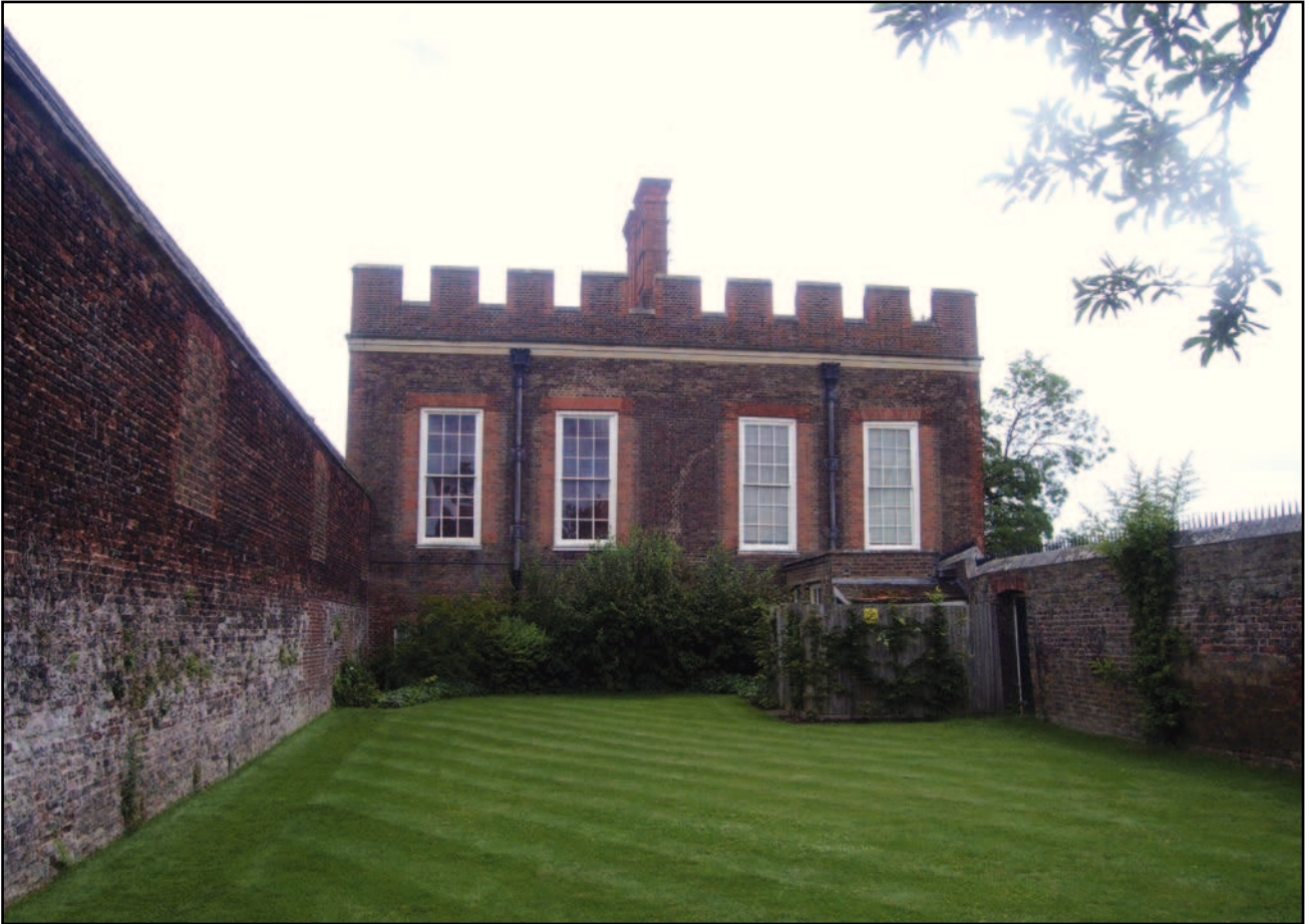
Plate 17: View of south elevation of Banqueting House
