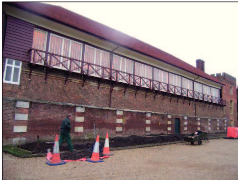
Plate 30: View of elevation following works
