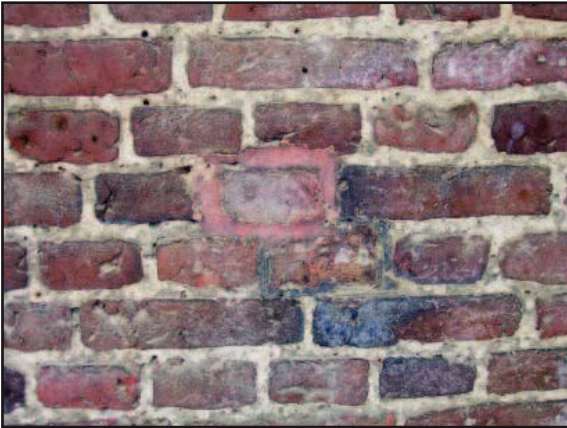
Plate 20: Mortar repairs
