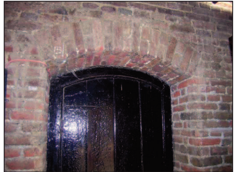
Plate 15: Detail of rebuilt arch lintel
