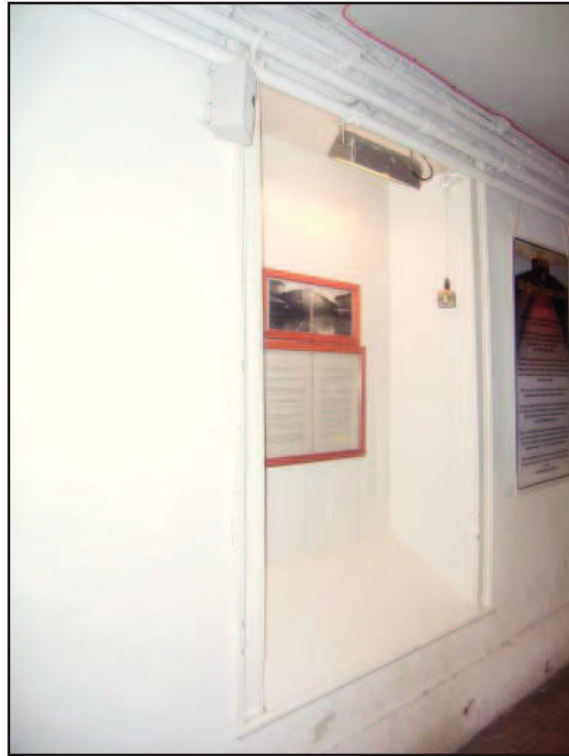
Plate 21: Internal view of north blocked window
