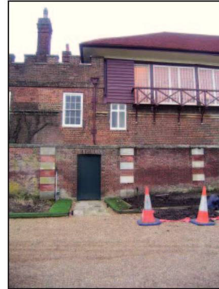
Plate 29: Entrance to south of tennis court, changing rooms and storage
