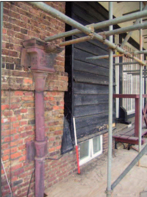
Plate 22: View of 19th century windows and adjoining brickwork
