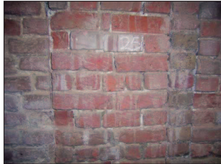
Plate 19: Infilled window opening to north end of elevation
