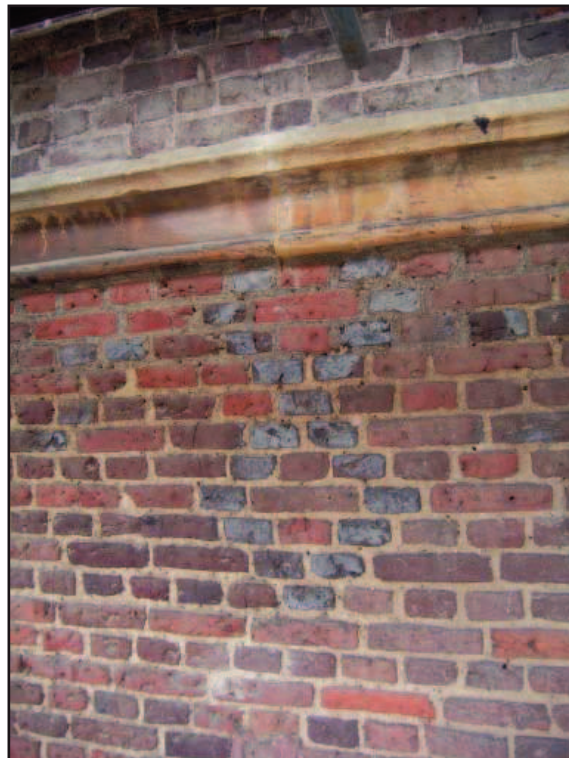
Plate 23: Open diamond diaperwork detail
