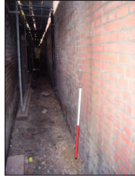
Plate 13: View of lower section of east elevation prior to works
