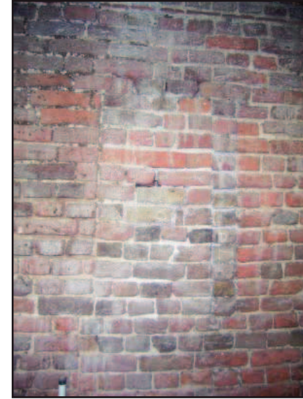
Plate 17: Detail of infilled window opening to south end of elevation
