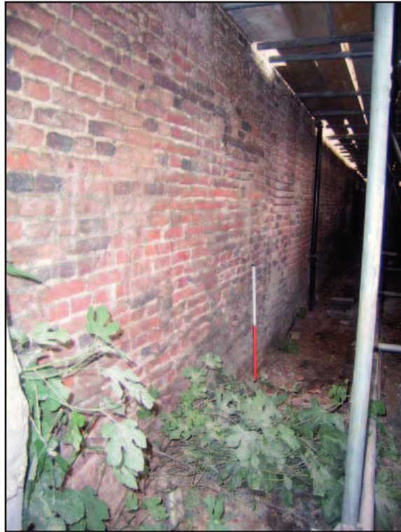
Plate 9: Lower section of east elevation prior to works
