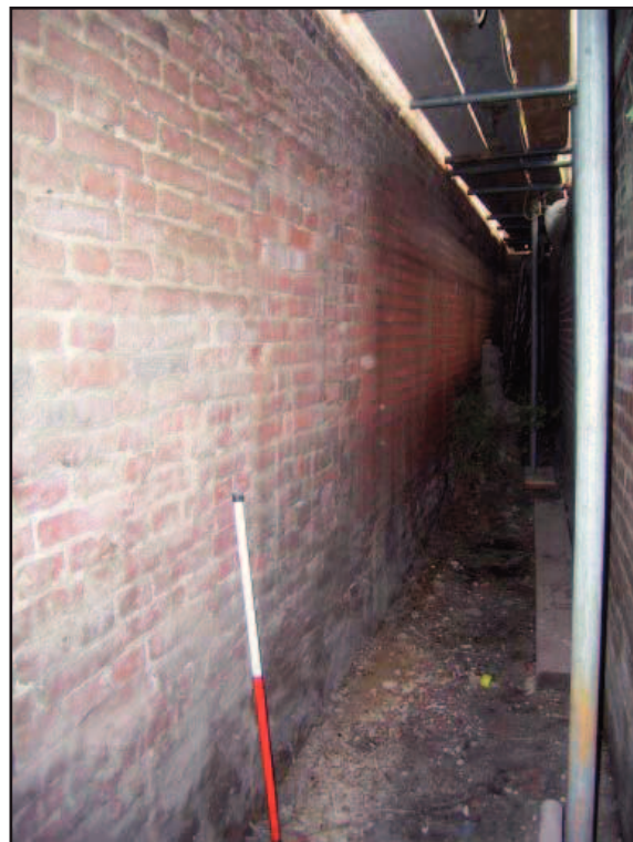
Plate 11: View of lower section of east elevation prior to works
