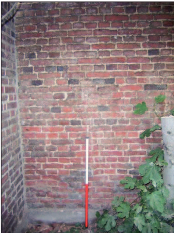
Plate 10: Tudor brickwork at south end of elevation
