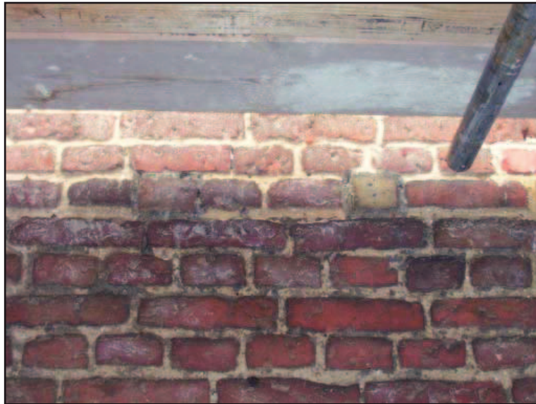
Plate 18: 18th/19th century putlog set within primary Tudor brickwork
