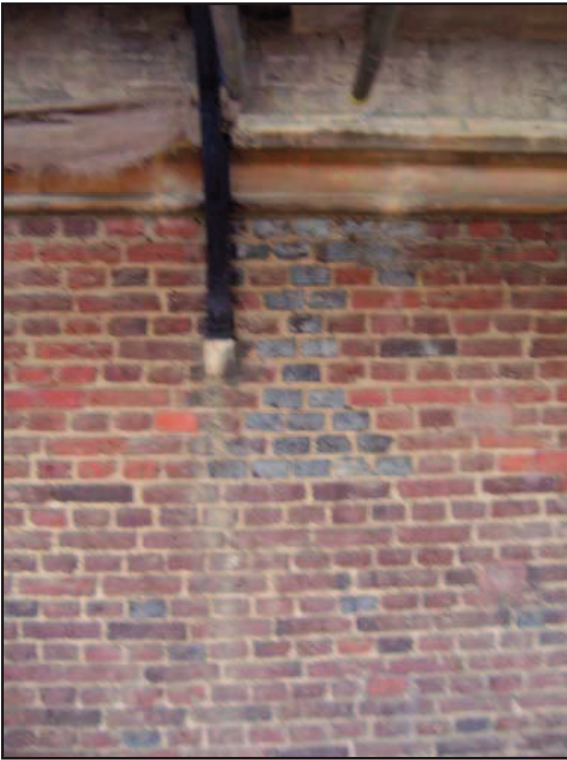
Plate 24: Closed diaperwork detail
