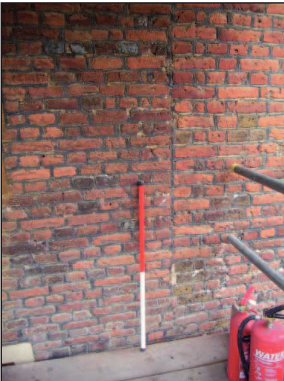
Plate 26: Straight joint showing extension to tennis court range
