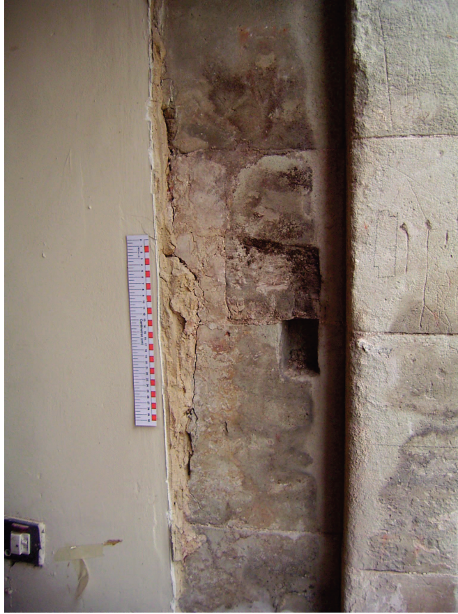
Plate 19: Detail of door fixing slot on southwest jamb
