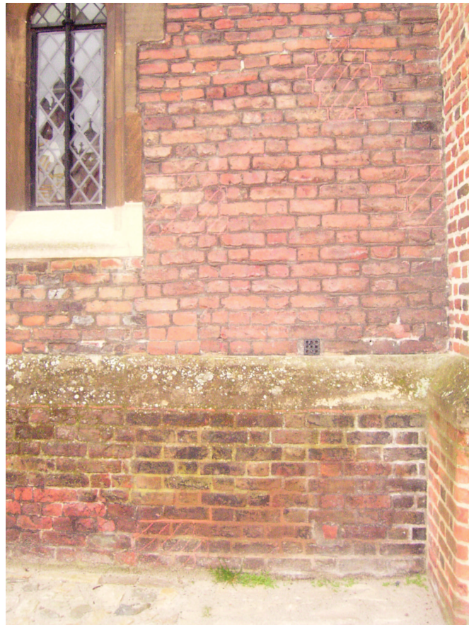
Plate 10: The brickwork covering the blocked doorway prior to removal
