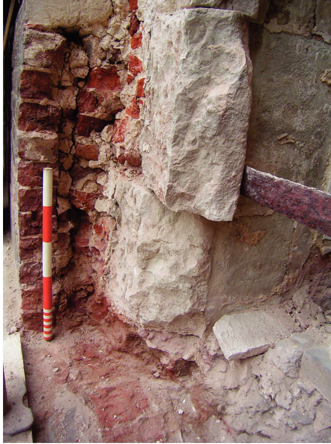
Plate 15: Detail of adjacent plinth northwest jamb
