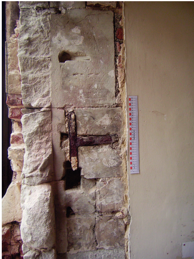
Plate 18: Detail of door fixing on northwest jamb
