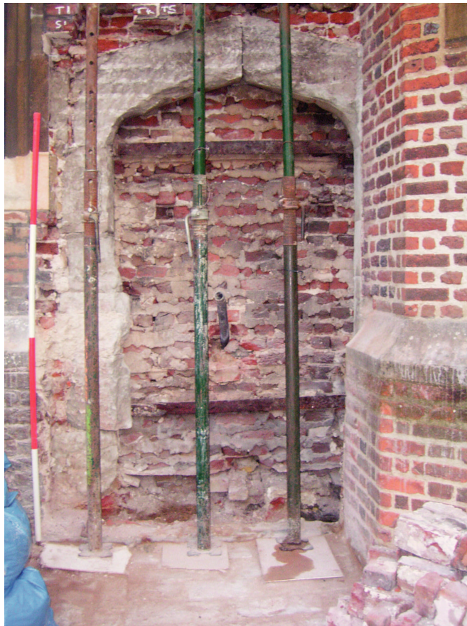
Plate 12: Following removal of all brick infill
