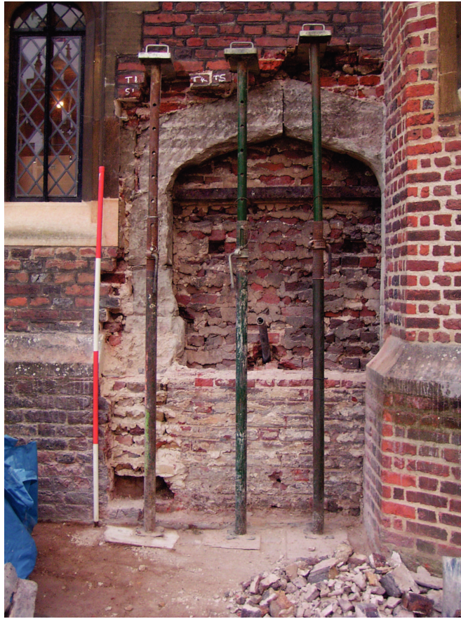
Plate 11: Following removal of facing and topmost infill brickwork
