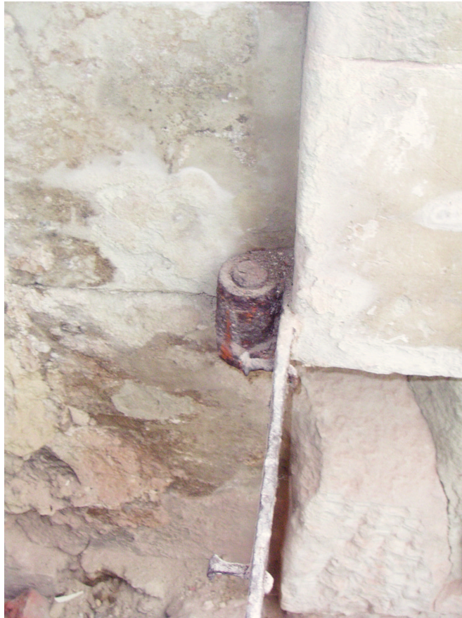
Plate 20: Detail of door lower pintle on southwest jamb
