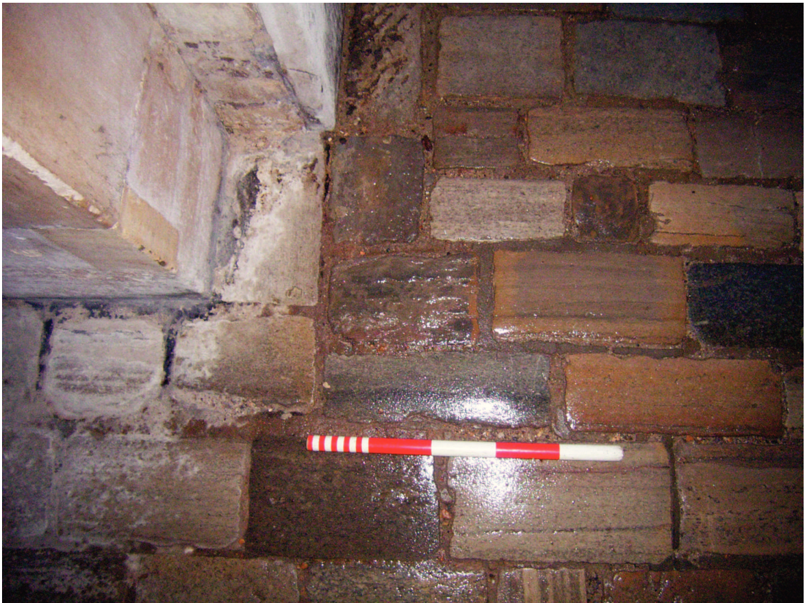
Plate 8: The southwest jamb granite setts prior to removal
