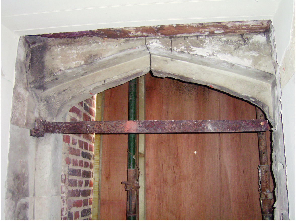
Plate 21: Detail of upper stonework from within shop
