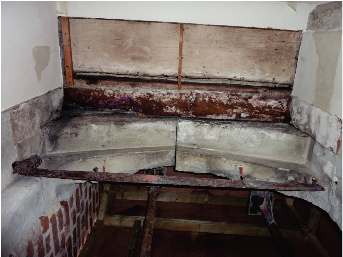
Plate 22: Detail of timber lintel replaced during works
