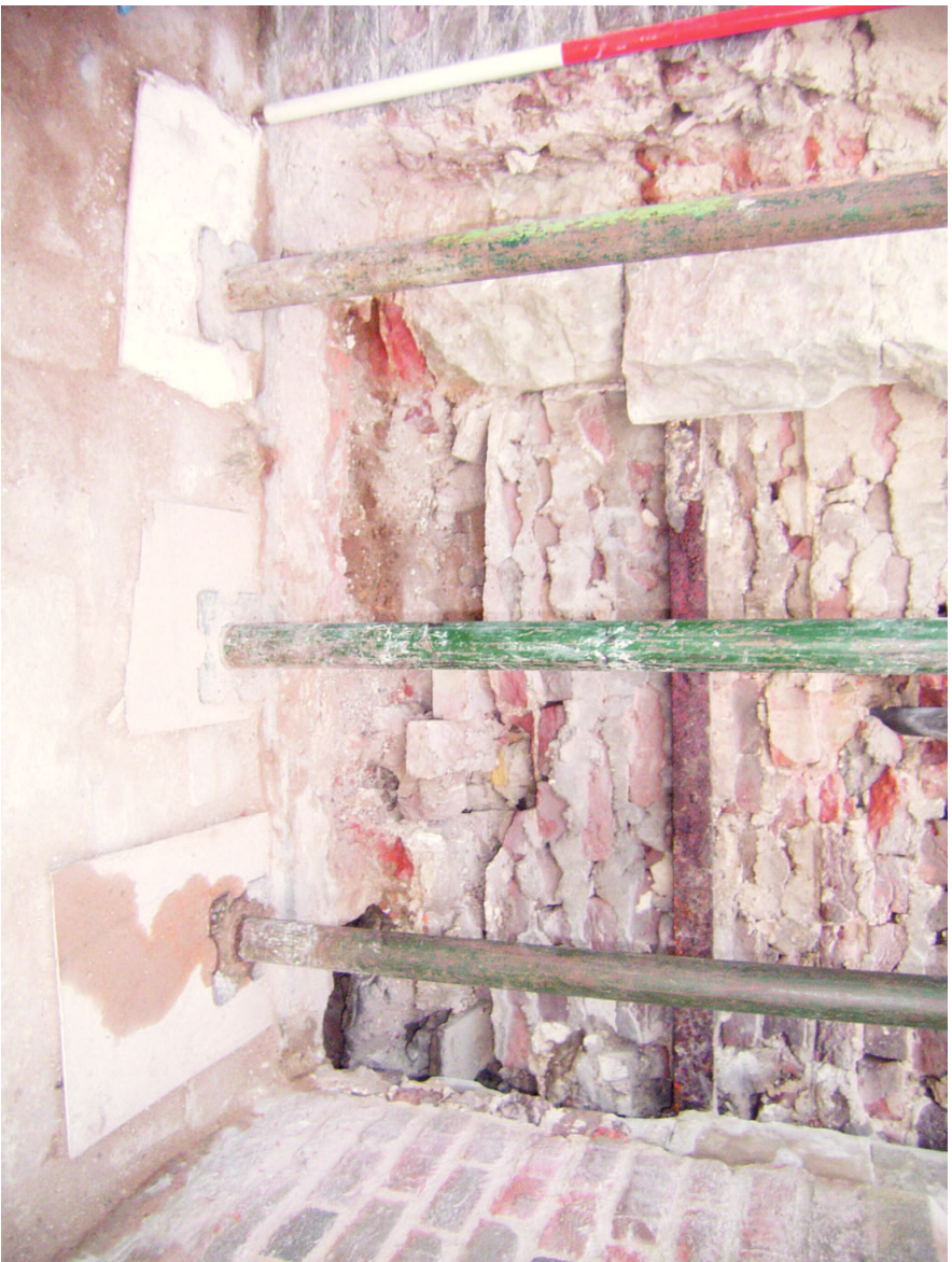
Plate 13: Detail of threshold
