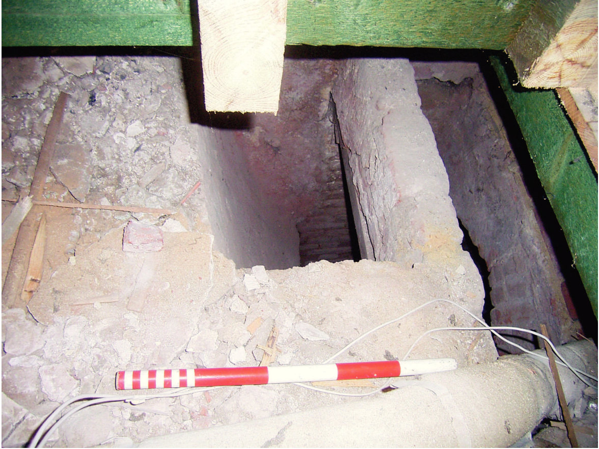
Plate 17: View of pre Wolsey vaulted area beneath floor within the shop
