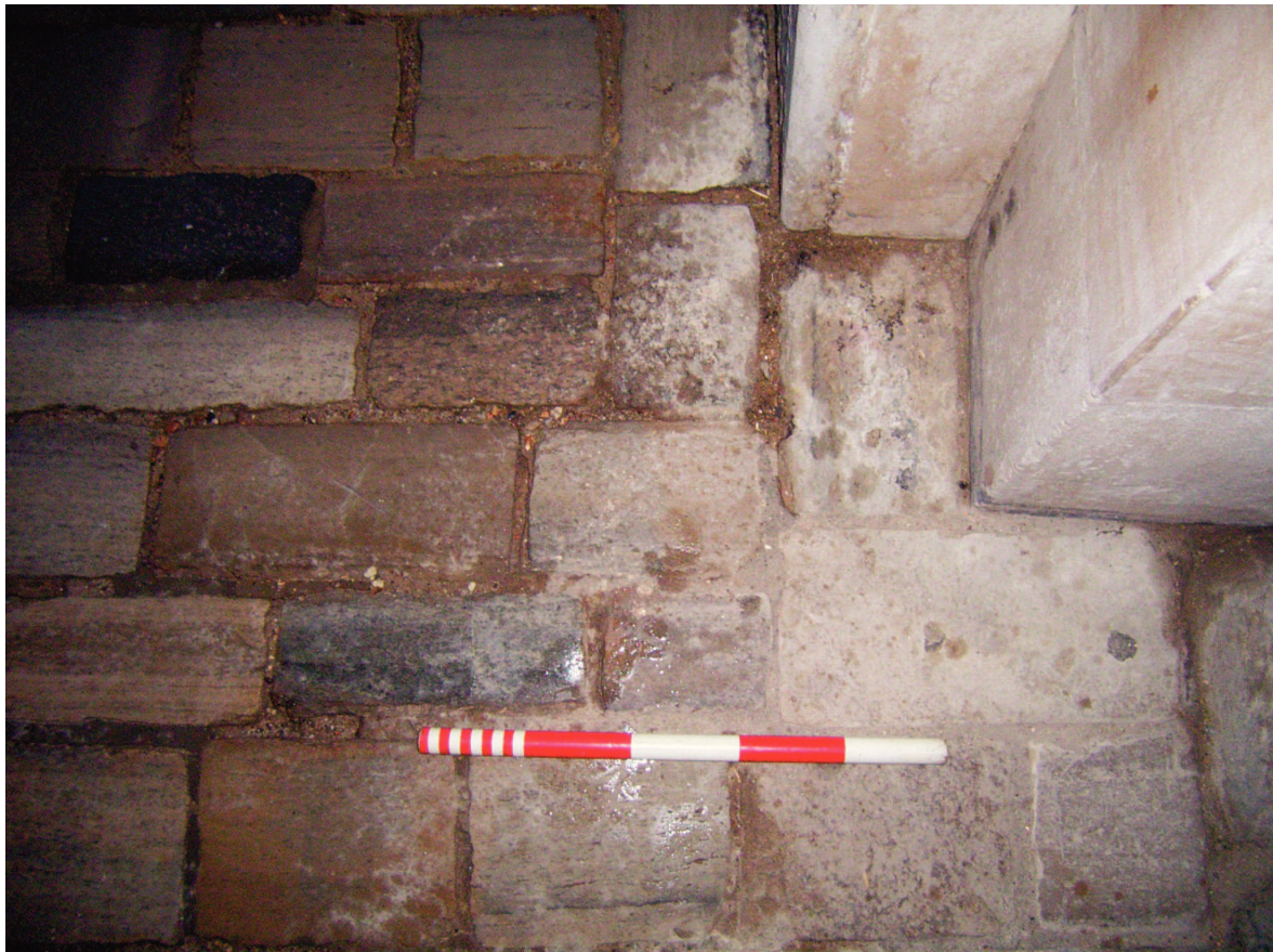
Plate 6: The northwest jamb granite setts prior to removal
