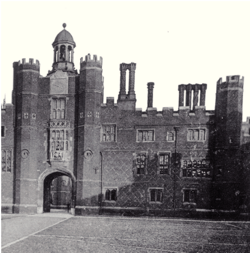
Plate 4: Detail from photograph of east range of Base Court showing blocked doorway with recent addition of plinth (pre 1891) © Historic Royal Palaces
